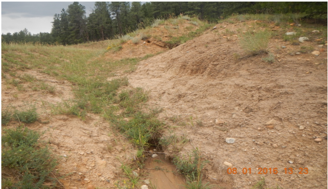
photo 6: North side of the location facing southwest. Diversion ditch is directing stormwater to the north side of the location.
