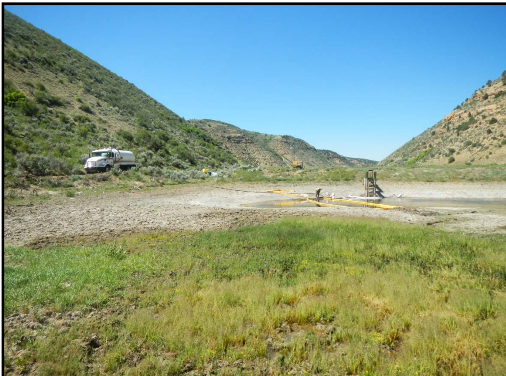
Stock pond. Skimming system pumping free-product and impacted water to truck. Gate could not be completely closed. Some flow continues downstream beyond pond.
