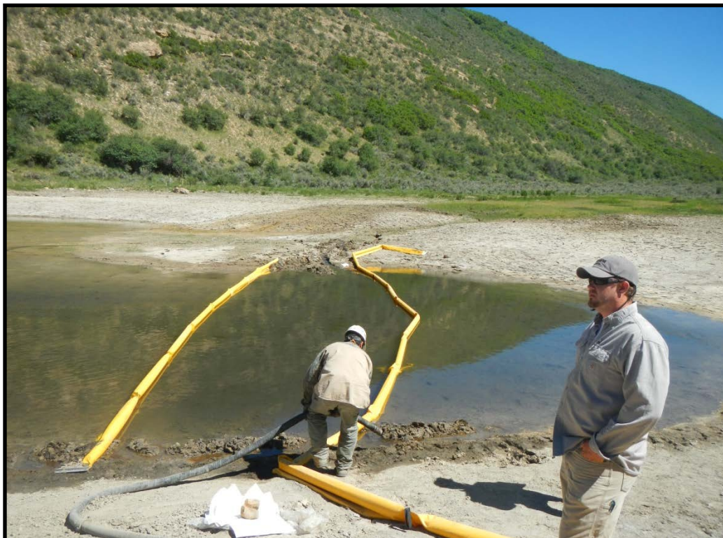
Stream channeled to concentrate free-product between yellow tubing. Skimming operation in process.
