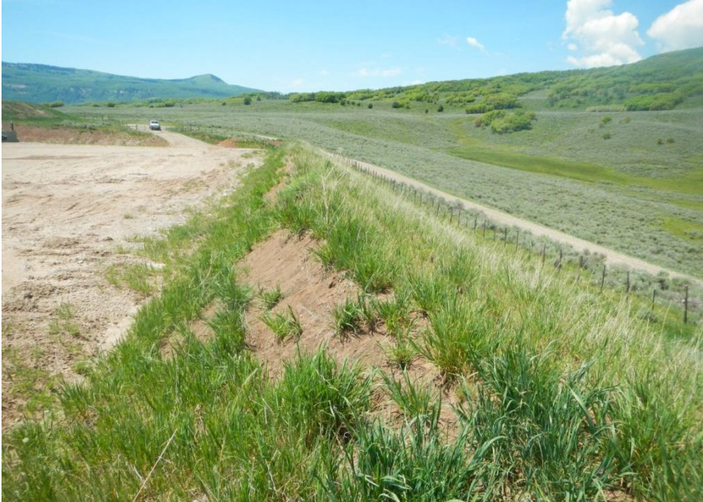
Photo 1. View of the northwestern portion of the project area from the northern corner facing southwestward. Cut and fill slopes are revegetating.
