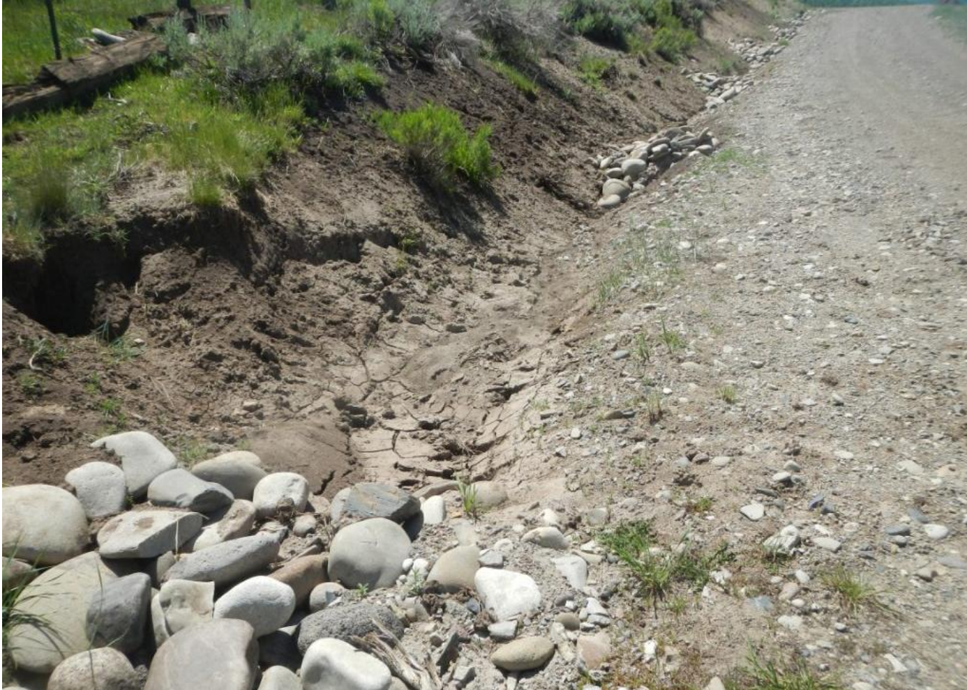
Photo 8. View of rock check dams placed along access road. Appear to be functioning at this time, but will soon need maintenance.
