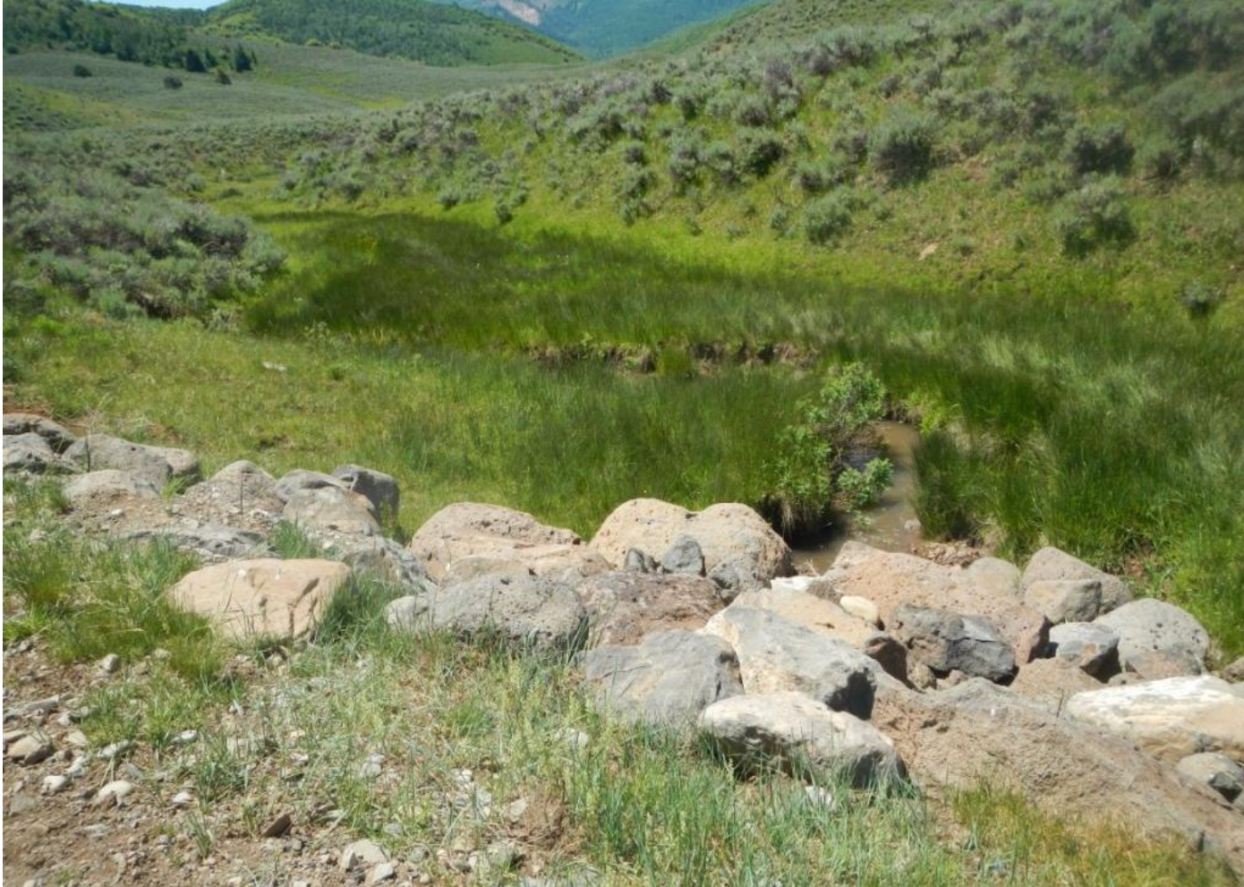
Photo 7. View of armoring at culvert along access road. Appears to be in good condition.
