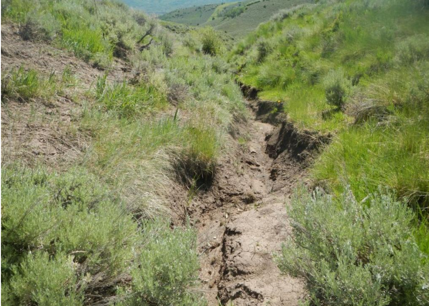
Photo 8. View of erosional channel that has formed on the south side of the access road where concentrated flows from the well pad and access road are eroding the drainage. Channel is approximately 3 feet wide and deep. Stormwater controls are needed stabilize erosion along this drainage.
