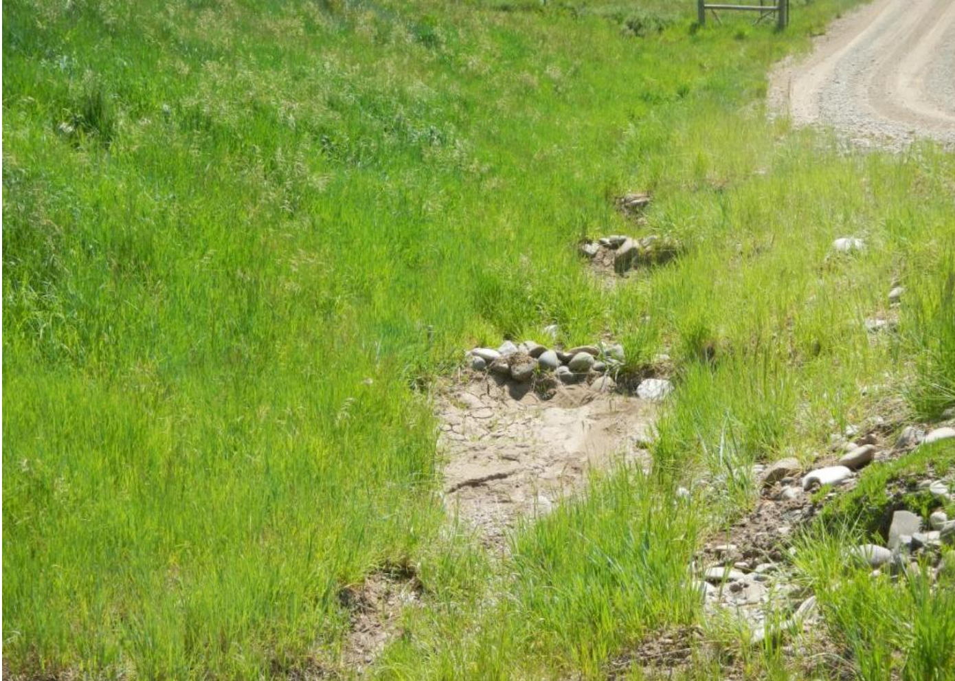
Photo 6. View of stormwater controls along the access road. Cobble check dams are used to de-energize flows. These are largely filled with sediment and need to be cleaned.
