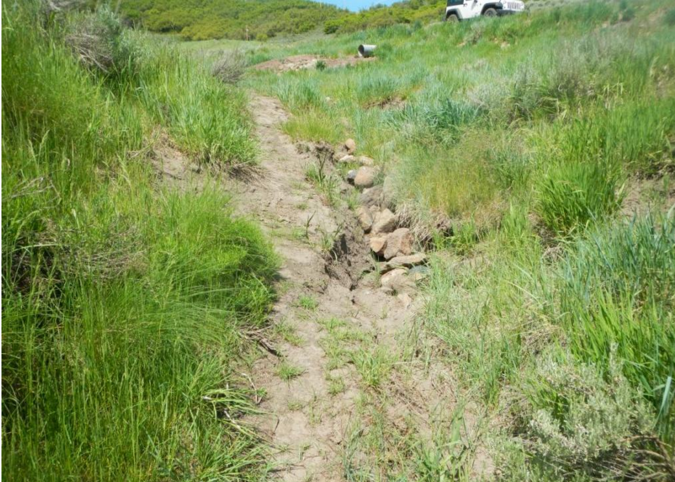
Photo 7. View of erosional channel on south side of access road. Stormwater BMPs are not functioning and stormwater is eroding the slope. Photo facing upslope toward where stormwater flows exit culvert on access road.
