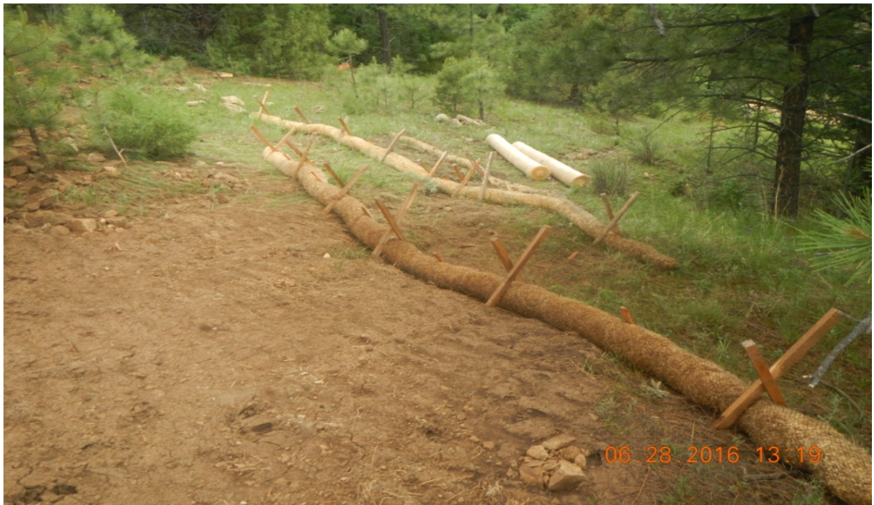
photo 12: There were excelsior wattles installed at the north perimeter of the location.
