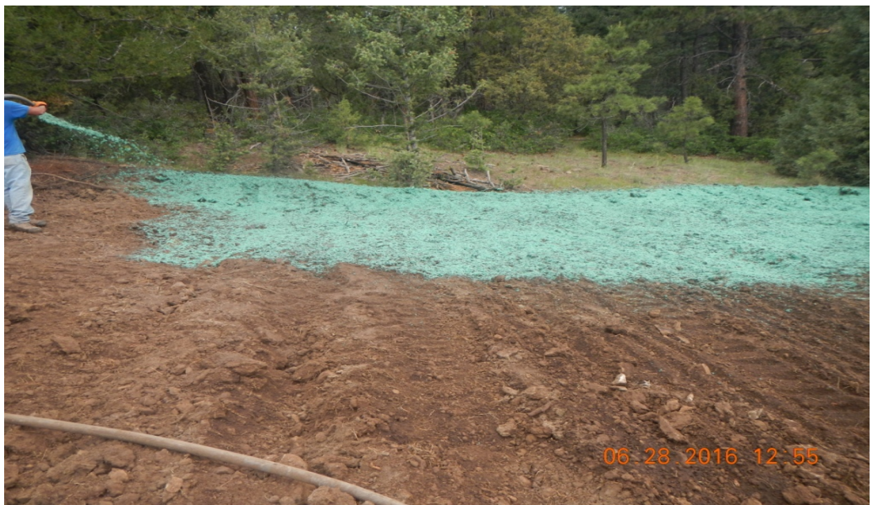
photo 6: A hydro mulch was in the process of being applied at the time of this inspection.
