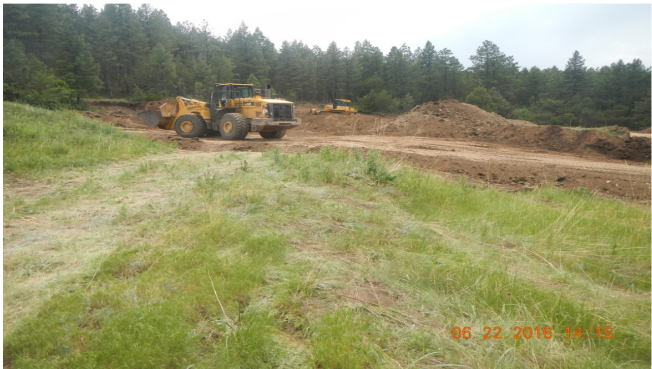
photo 2: Equipment in process of recontouring the location.
