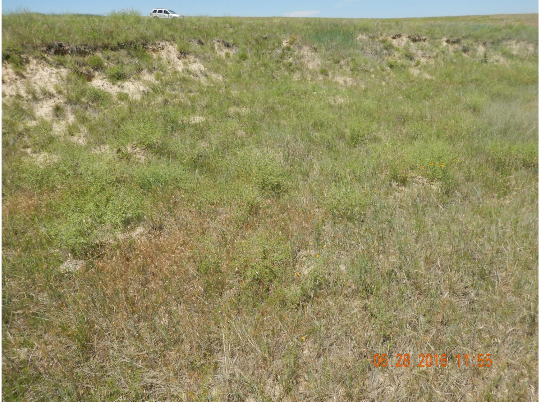
Figure 8: Photo taken from the southwest corner of the location, facing west. Photo shows erosion on cut bank. Photo shows location had not been recontoured.
