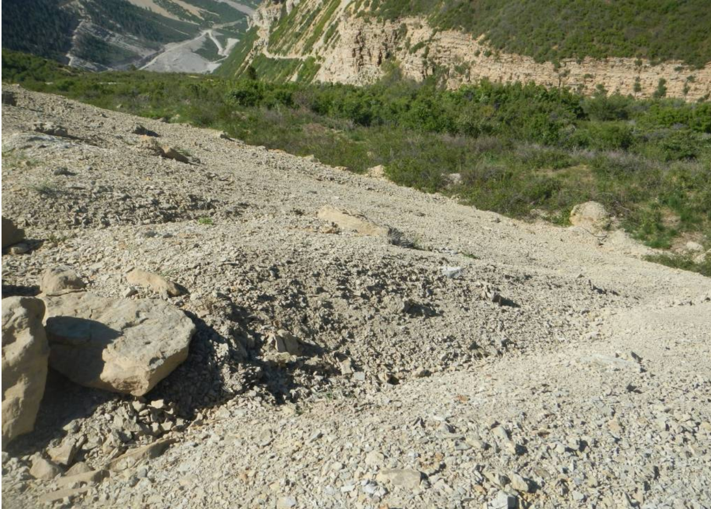
Photo#4:. Areas of Fill Slope where material begins to slough and Channel Down Slope.
