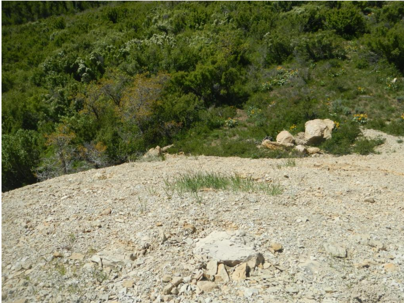
Photo#9: Fill Slope at East side of Location Bellies out; accelerating movement of Material off Location.
