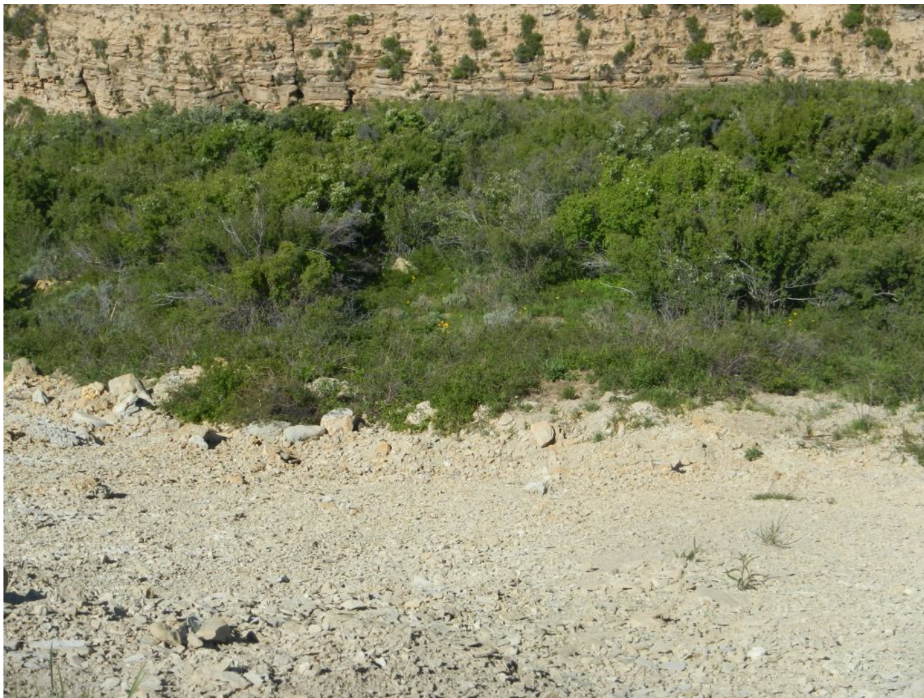
Photo#5: Fill Slope on West side of Location; Material is rattling, migrating into Vegetation.
