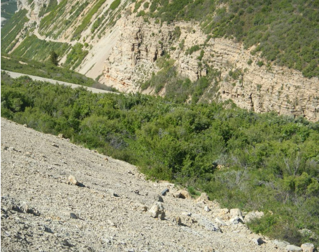
Photo#8: Unstabilized Fill slope Material again moving into Vegetation & lack of effective BMP at base of Slope.
