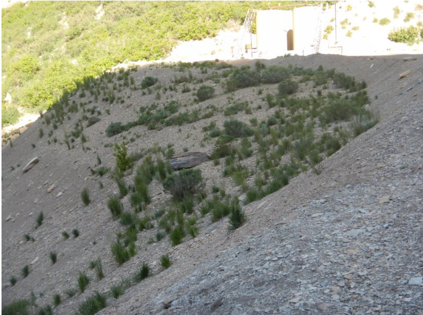
Photo#4: Upper Portions of Fill Slope have vegetation establishing, while Lower areas remain unstabilized .
