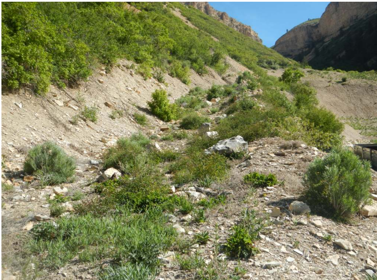
Photo#3: This Bench has been & is effective in stabilizing Slope behind Wells
