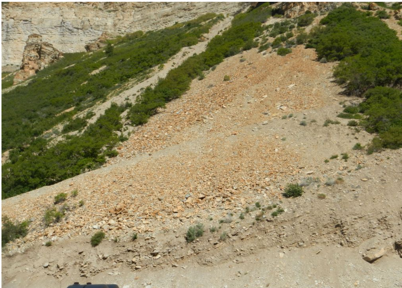
Photo#2: Cut Slope and Disturbance associated with site need to be Stabilized
