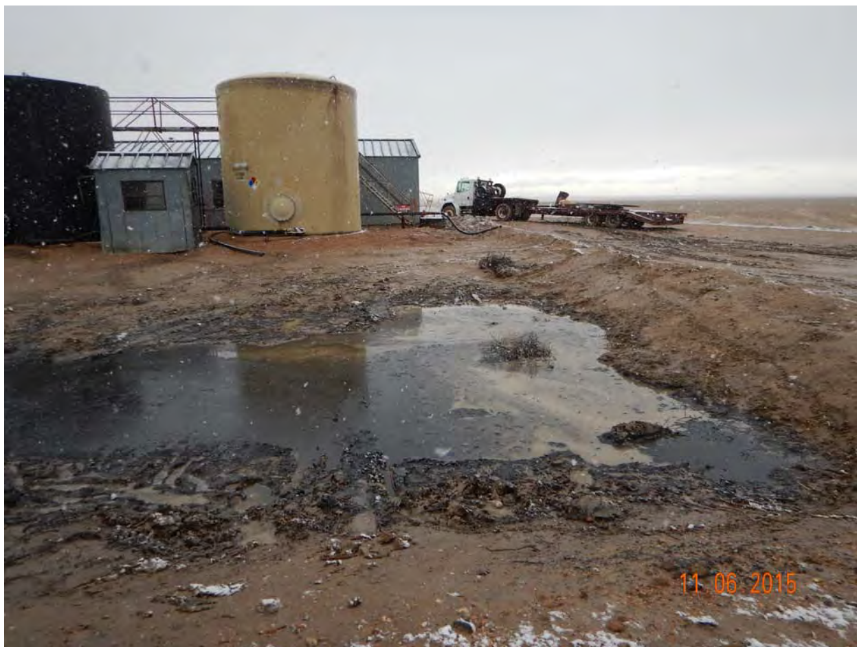
Field Photo 3: Oil and Water in secondary containment at NE corner of berm (looking W).
