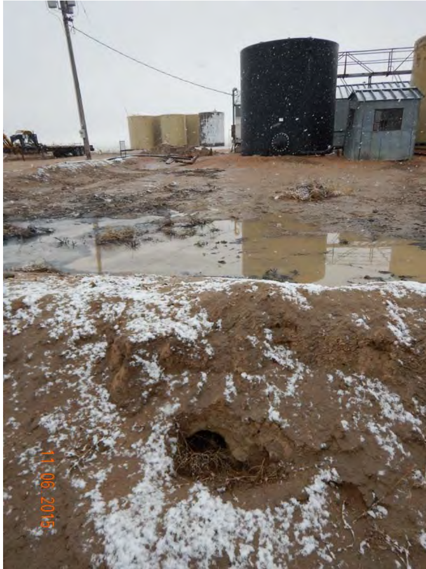
Field Photo 4: Large burrow in secondary containment (SE corner, looking W).
