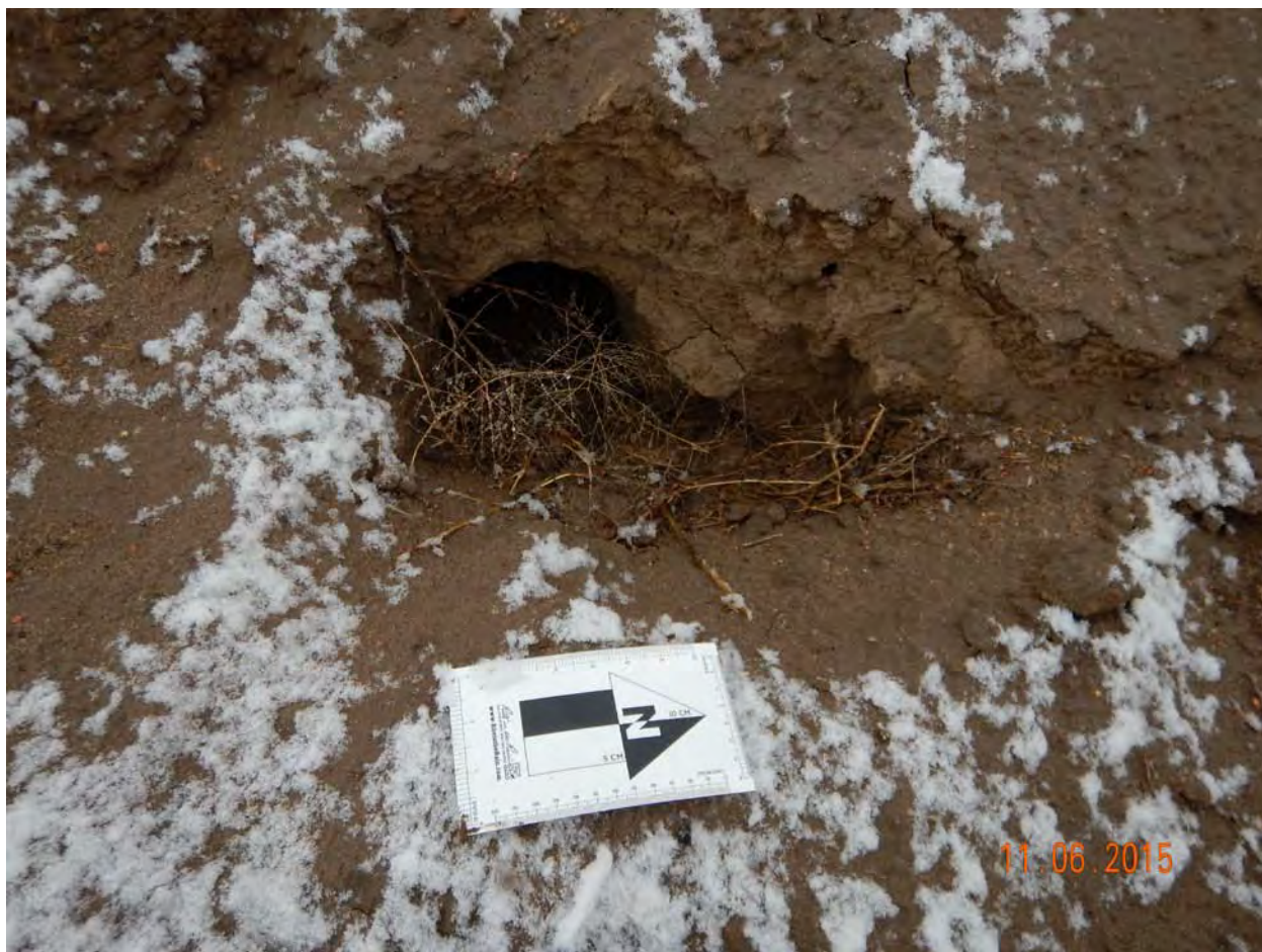
Field Photo 5: Close up shot of large burrow in SE corner of secondary containment with scale (looking W).
