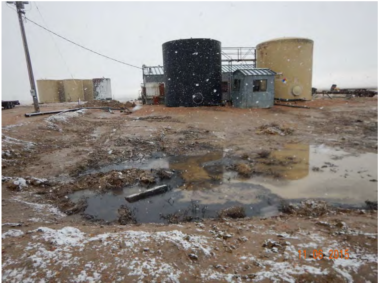
Field Photo 2: Oil and water in secondary containment at SE corner of berm (looking W).
