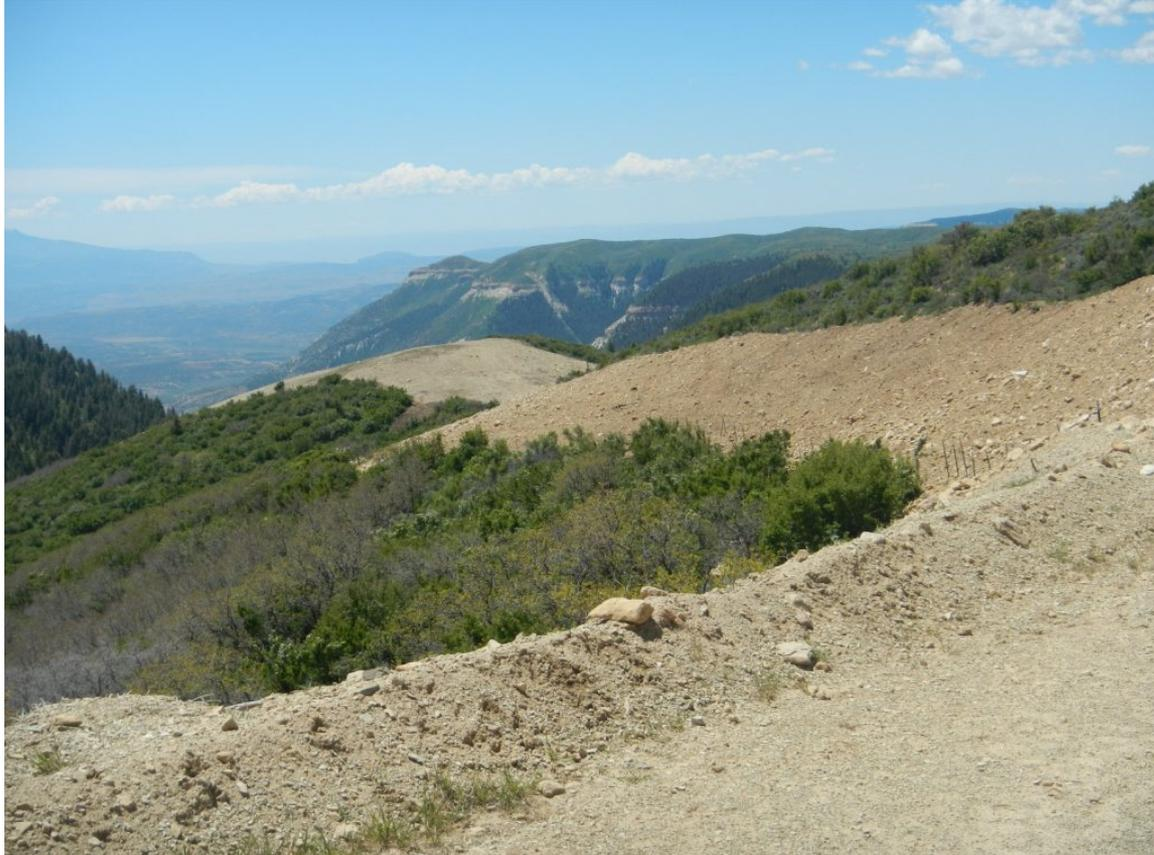
Photo#1: Access Road into Location in process of reclamation.
