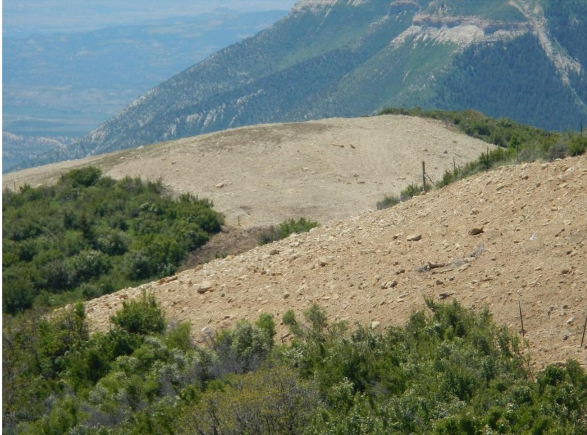
Photo#3: Steep Slopes will need monitoring to assess need for SW BMP's to stabilize Location until Vegetation establishes.
