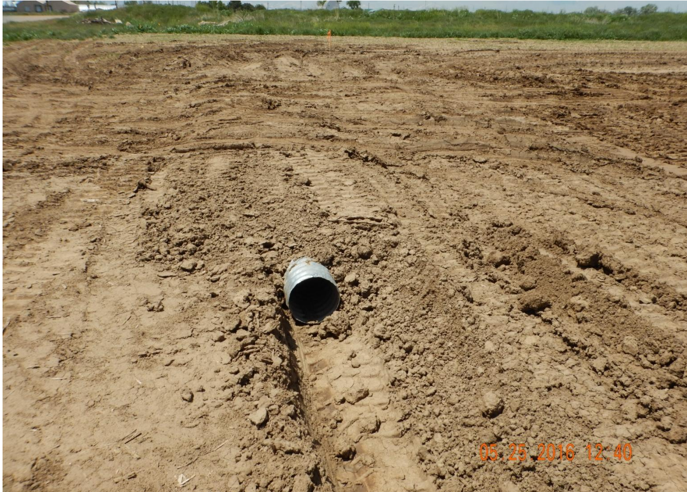
Photo 3. Photo taken from entrance of location, facing West. Second culvert installed along stormwater ditch.
