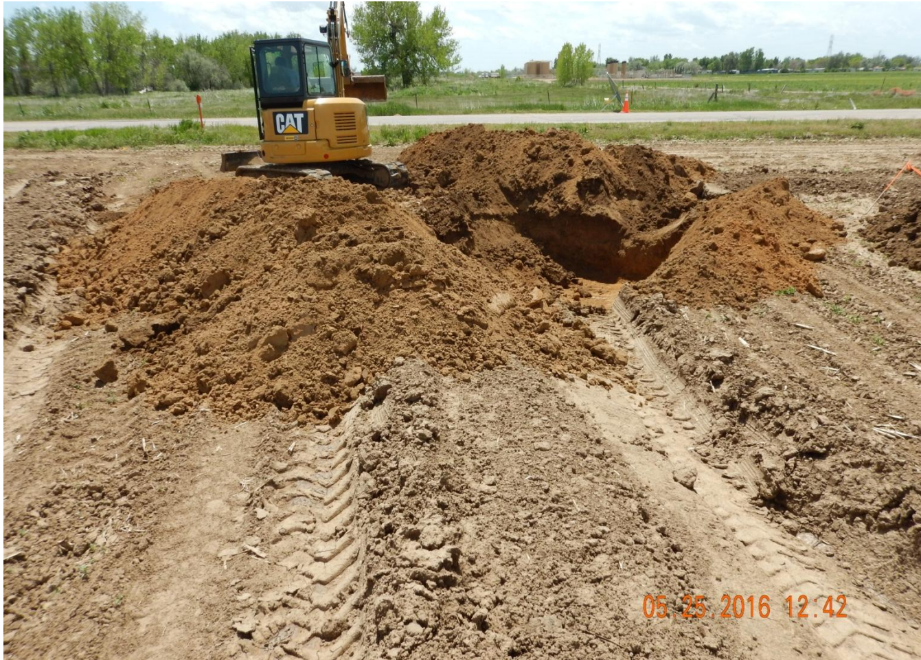
Photo 5. Photo taken from southeast location, facing South. Sediment trap being constructed.
