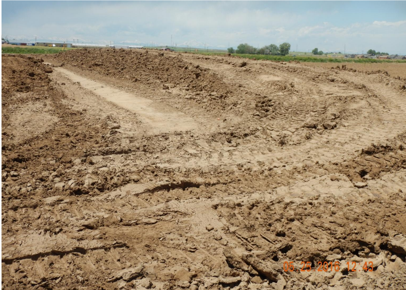
Photo 9. Photo taken from eastern location, facing West. Topsoil stockpile in center of photo. Topsoil stockpile needs to be stabilized upon completion of salvage process.
