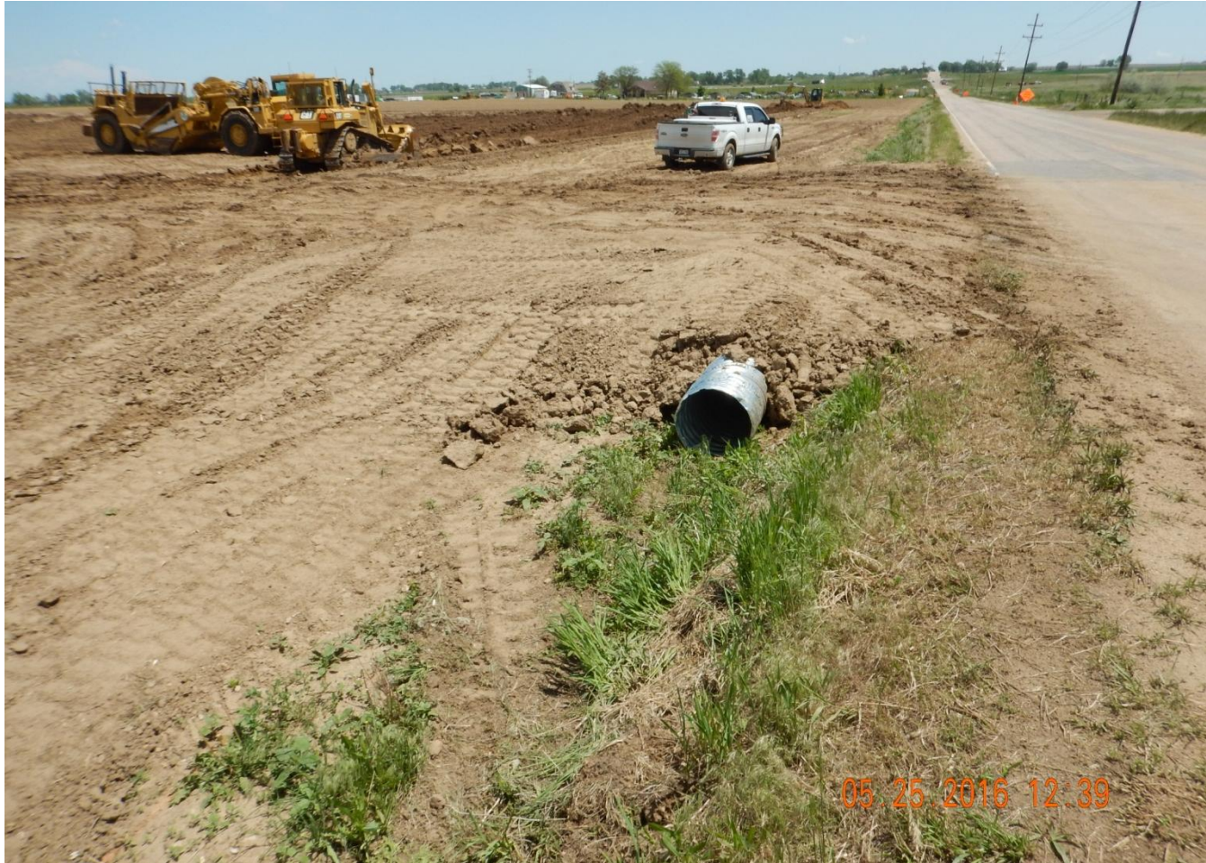
Photo 1. Photo taken from entrance of location, facing East. Culvert installed at entrance.
