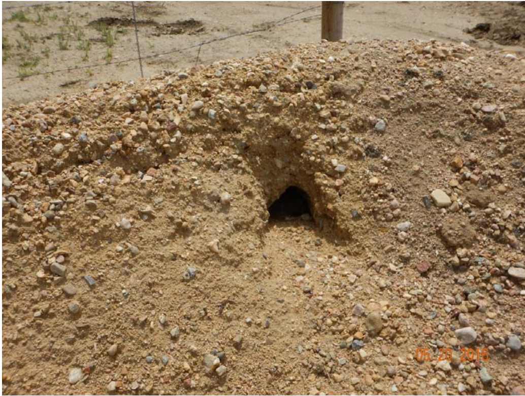
Burrows observed around tank battery berm at KPK/Extraction Becky #1 Tank Battery – 5/20/2016, Arauza.
