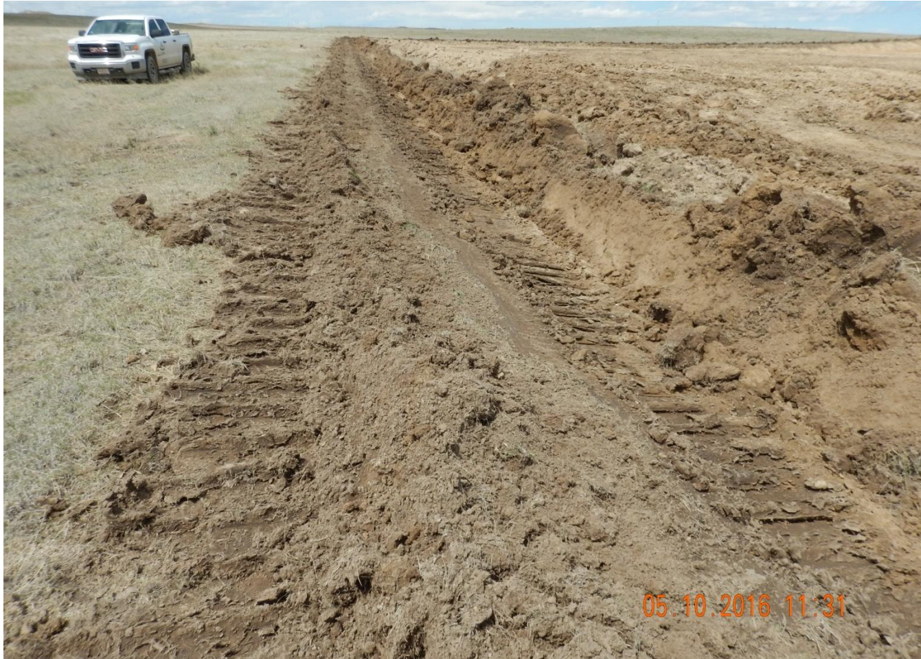
Photo 1. Photo taken from southeast location, facing West. Stormwater BMP installed in center of photo.
