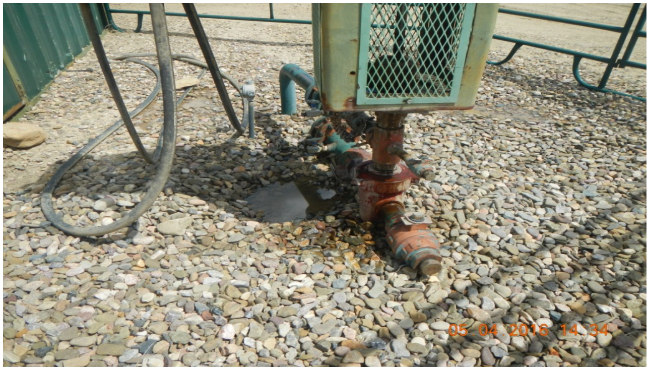
photo 2: There is a dripping water leak from the well which was noticed in the previous inspection.
