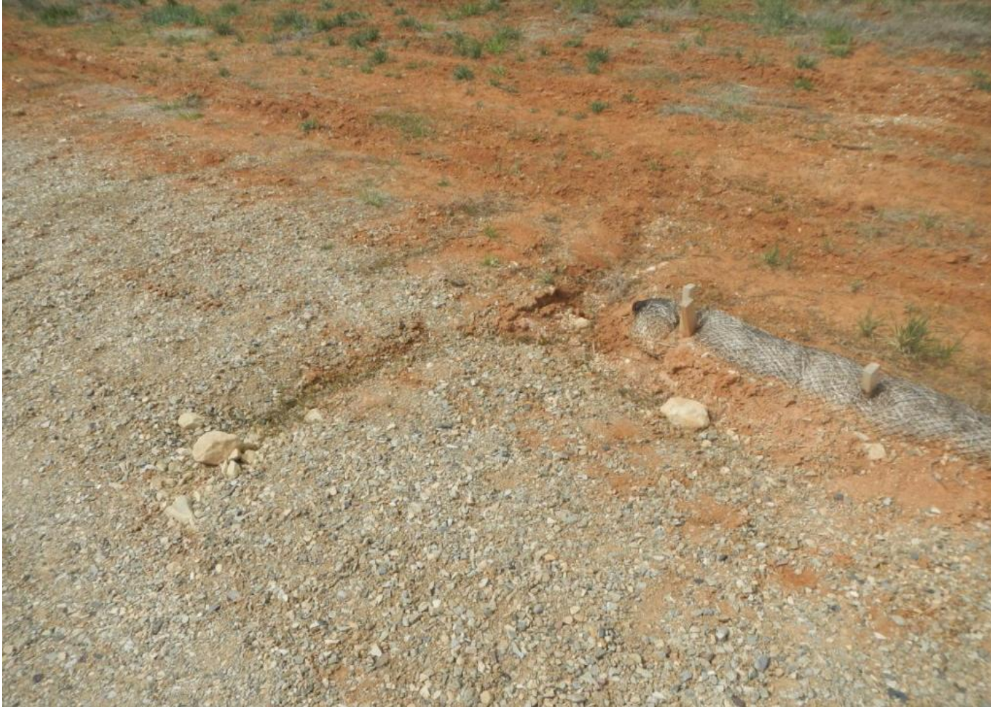
Photo 6. View of erosion occurring along the edge of a wattle on the southwestern edge of the well pad.
