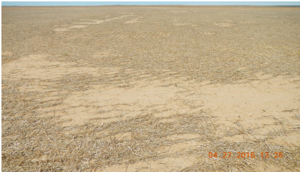
photo 3: South side of the location facing north. Straw mulch is providing temporary soil stabilization.
