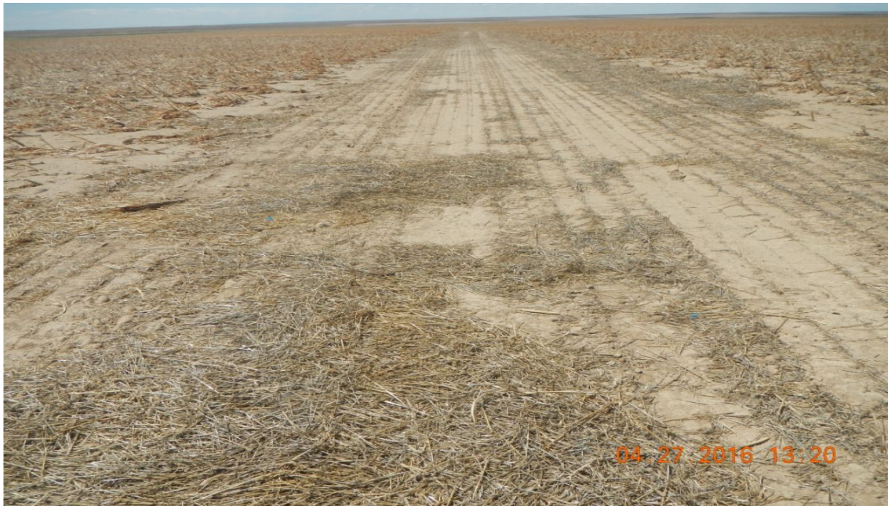
photo 1: Facing west along the former access road. Straw mulch has been applied and crimped into the soil.
