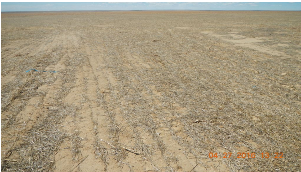
photo 2: East side of the location facing west. Straw mulch has been applied and crimped into the soil.
