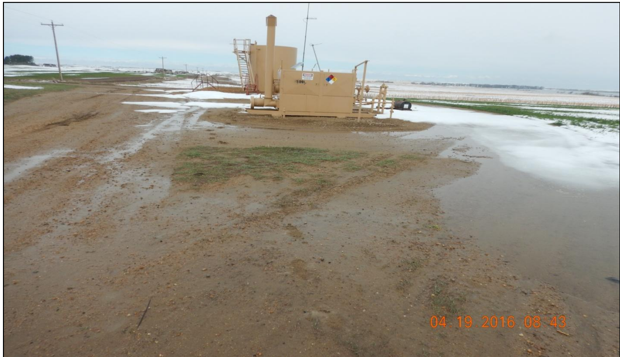
Photo 2: Photo taken 4/19/16 east of tank battery location, facing West. This photo illustrates where stormwater initiates then travels west onto cropland.
