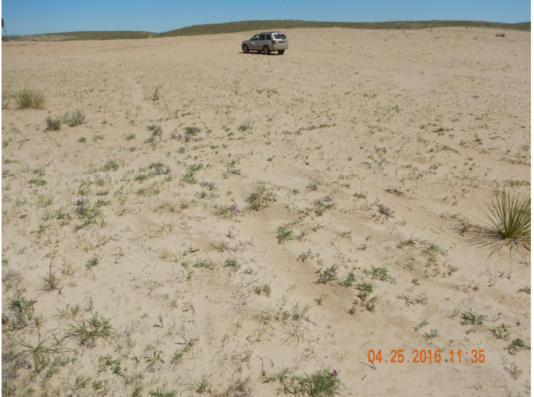
Figure 3: Photo taken from the southwest corner of the location, facing east. Photo shows large areas of the location where revegetation is not progressing.
