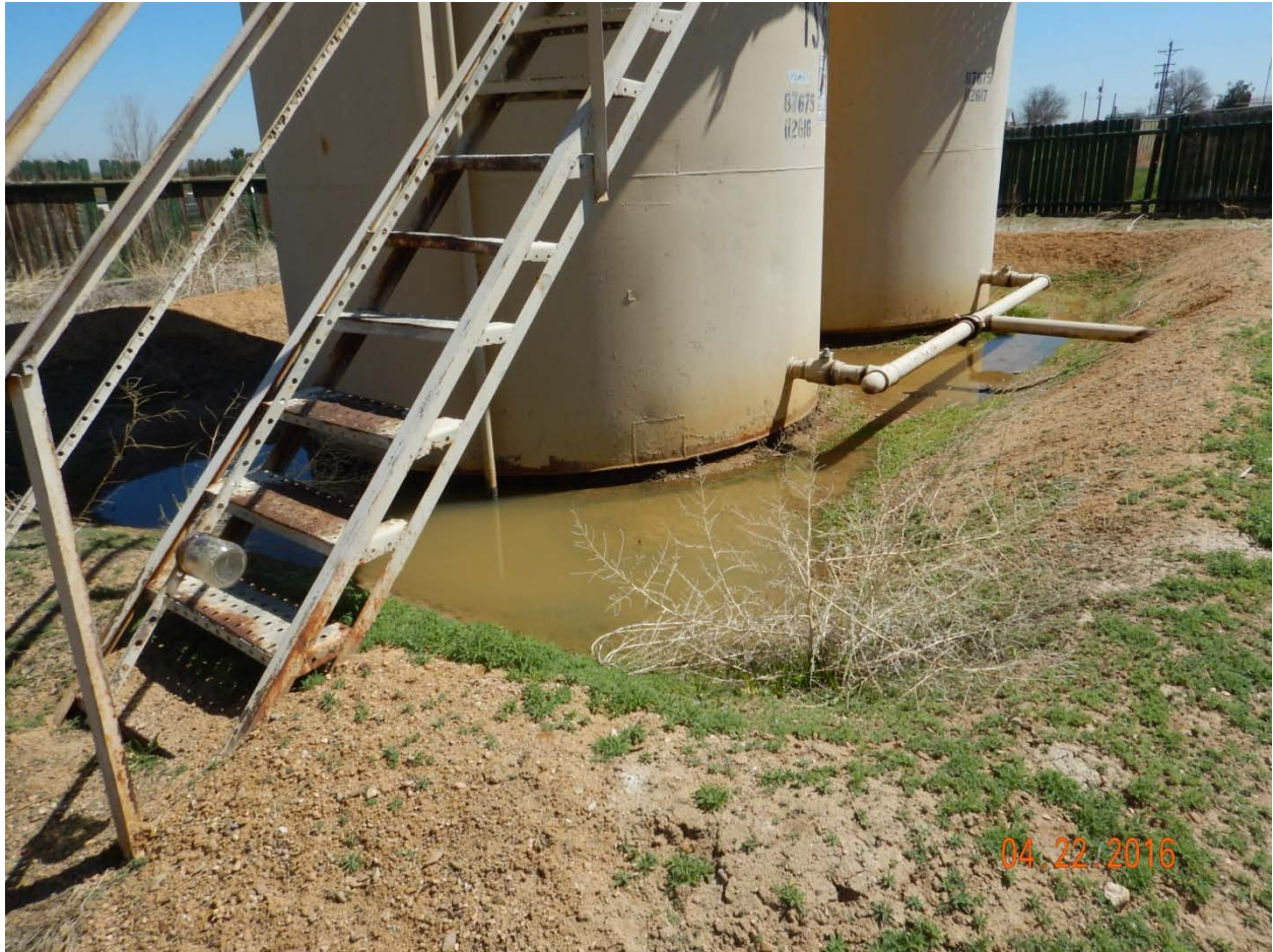
Figure 10 - Water inside of tank berm.
