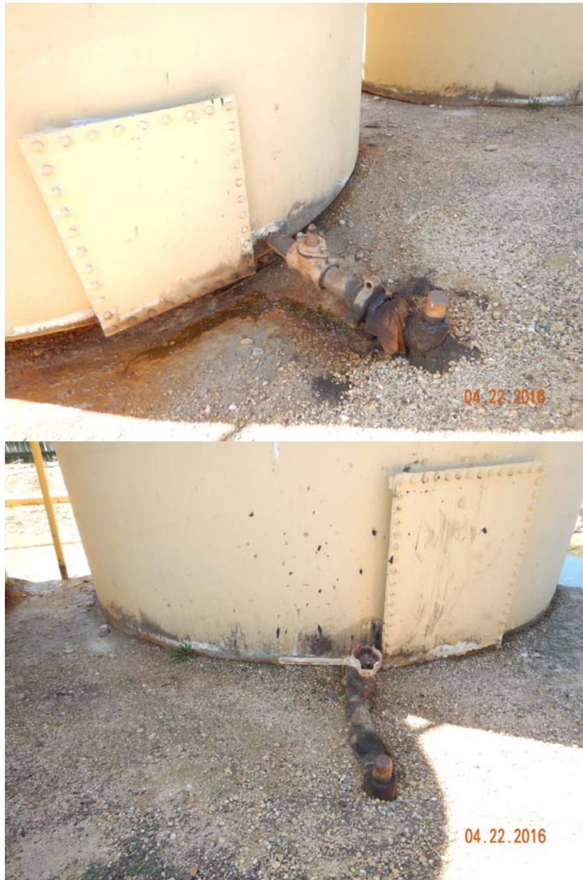
Figure 11 - Localized, oil stained soil at leaking valves on both crude oil tanks.
