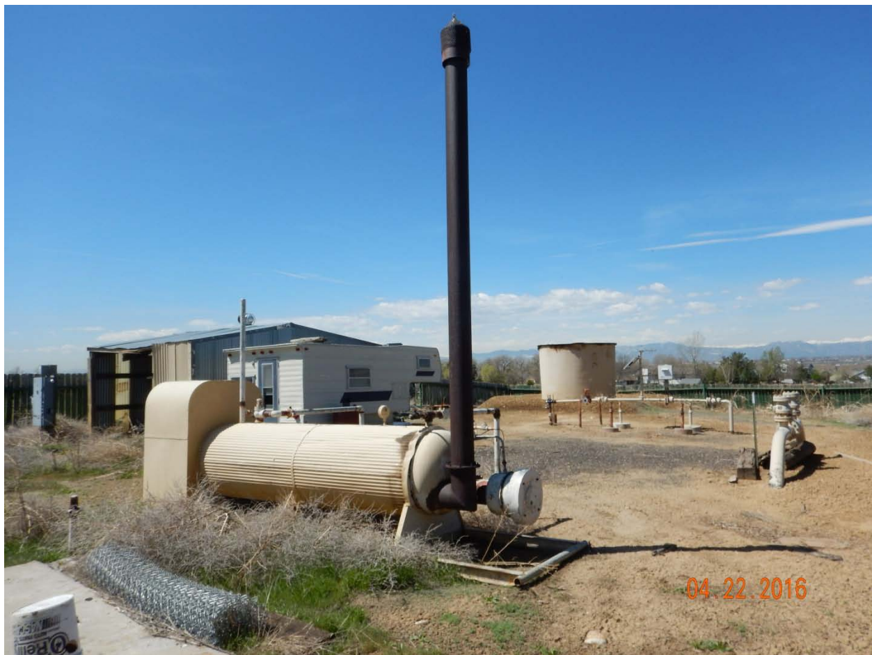
Figure 15 - Heated horizontal separator with view of shed, produced water tank, and pig launcher. Note site-wide weeds, debris, and unused equipment.
