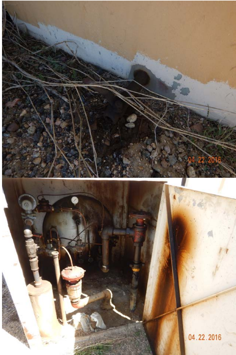
Figure 16 - Localized, oil-stained soil associated with heated horizontal separator.
