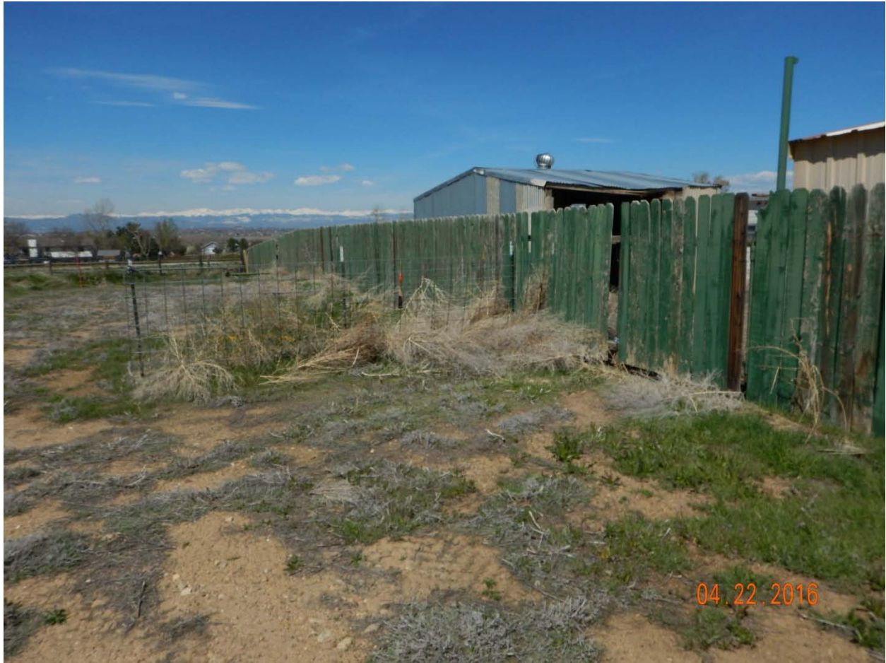
Figure 6 - Accumulation of weeds and gaps in tank battery fence.
