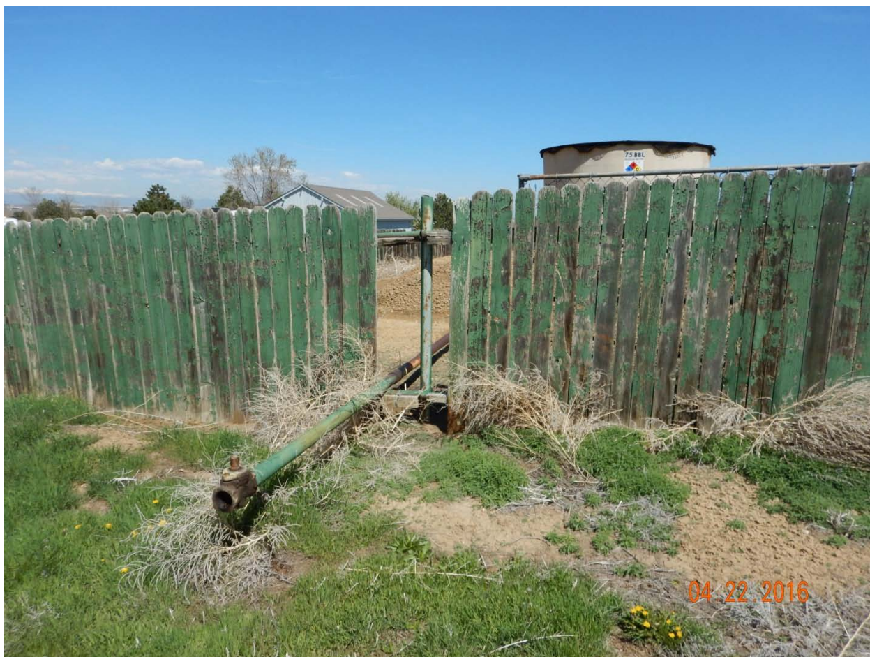
Figure 7 - Produced water tank loadout lacking secondary containment (note weeds and gap in fence).
