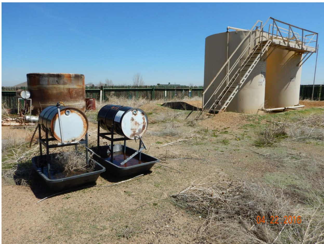
Figure 8 - Crude oil tanks, site-wide weeds/debris/unused equipment, chemical storage drums. Note water inside of secondary containment devices (foreground).
