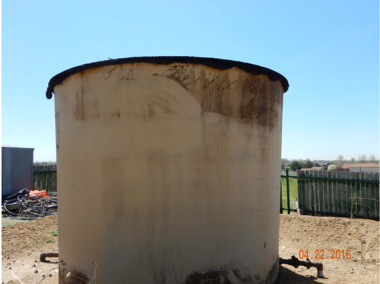
Figure 17 - Oil stains on top and bottom of fiberglass produced water tank.
