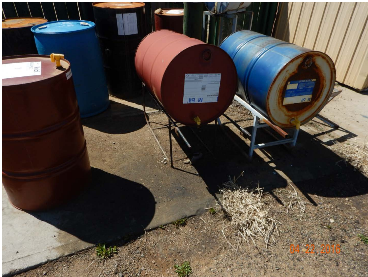
Figure 13 - Localized staining of cement and soil beneath chemical storage drums.
