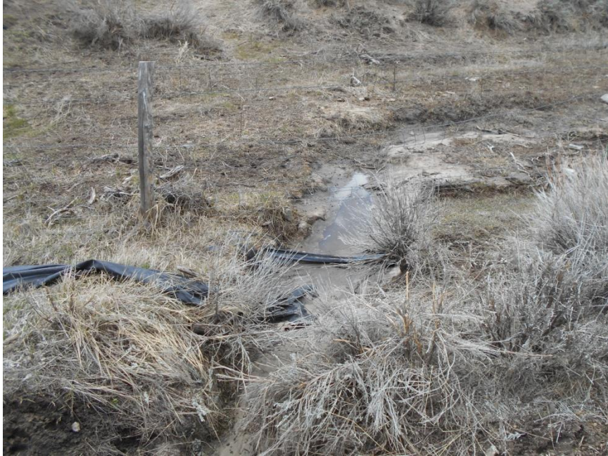
Breach in berm on SW side of pad
