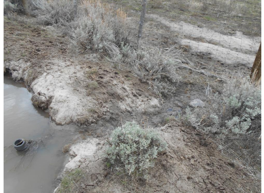
Breach in berm of retention pond
