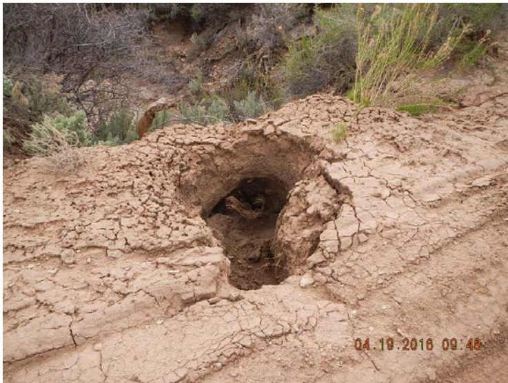
Area of erosion at the gate of the access road. Continued erosion may impede access to locations.
