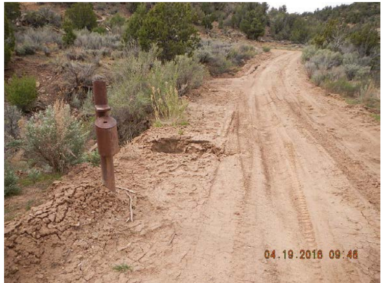
Area of erosion at the gate of the access road. Continued erosion may impede access to locations.
