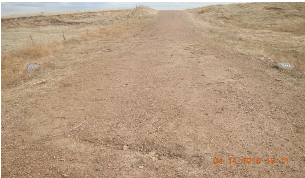
photo 4: Facing south along the access road. Area of subsidence and erosion has been repaired at Lat/Long: 38.74998,-104.55221.
