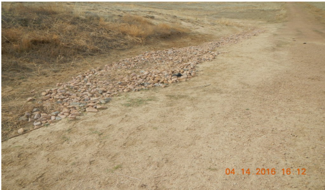
photo 8: Facing northwest. It appears rip/rap rock has been placed where erosion was occurring along the west side of the access road. Additional BMP's are needed in this area of the access road.
