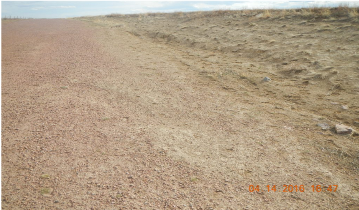
photo 7: Facing at the Opposite (west) side of the access road. This area along the access road is susceptible to further erosion.
