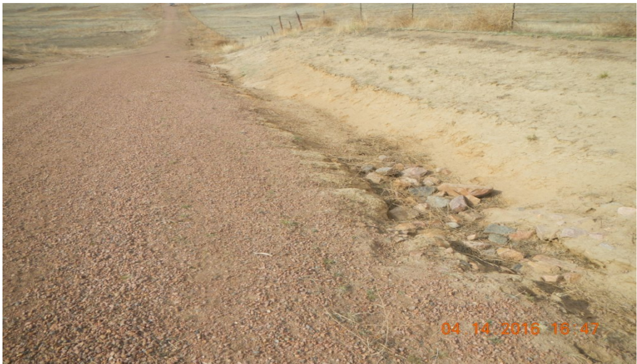
photo 6: Facing back north toward the east side of the access road. This area along the access road is susceptible to further erosion.
