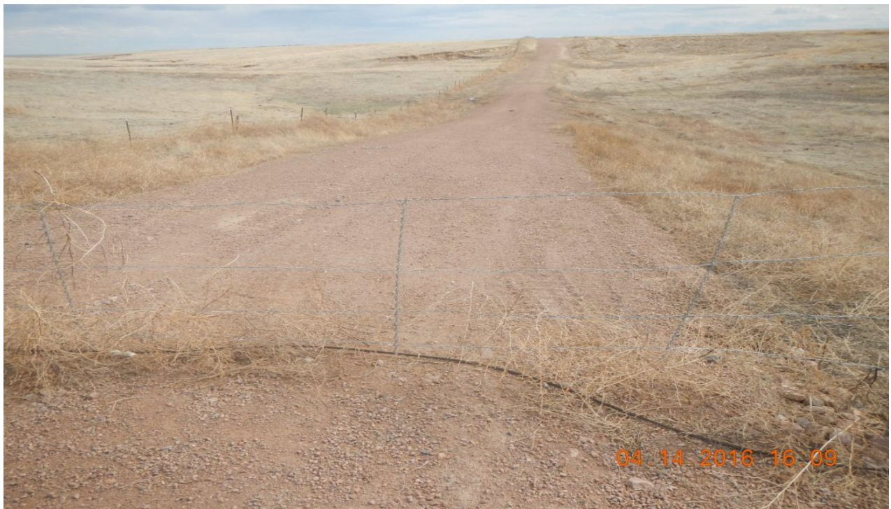
photo 2: Facing south along the access road. Metal gate and cattle guard removed which was replaced with a wire gate.
