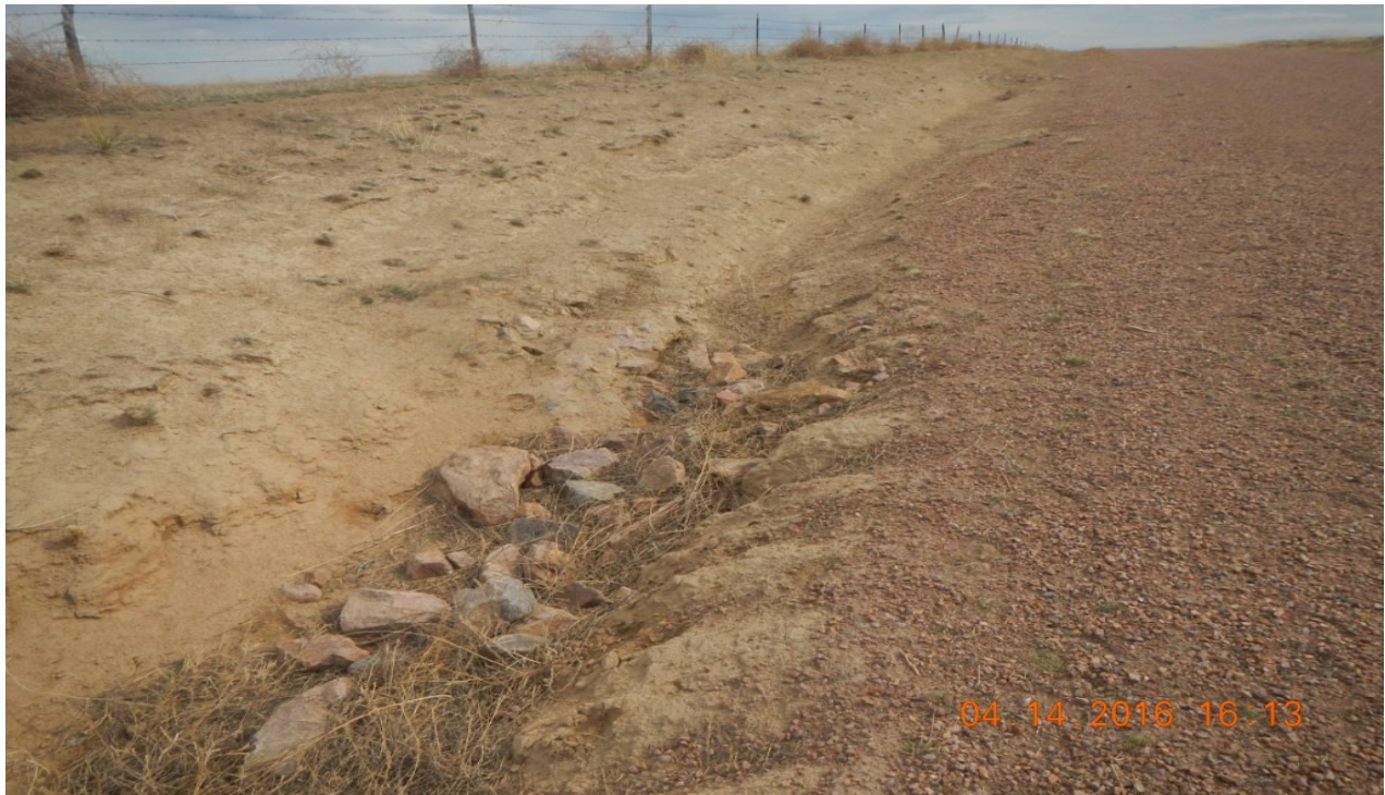
photo 5: BMP's have not been installed along the east side of the access road where the slope increases. This area along the access road is susceptible to further erosion.
