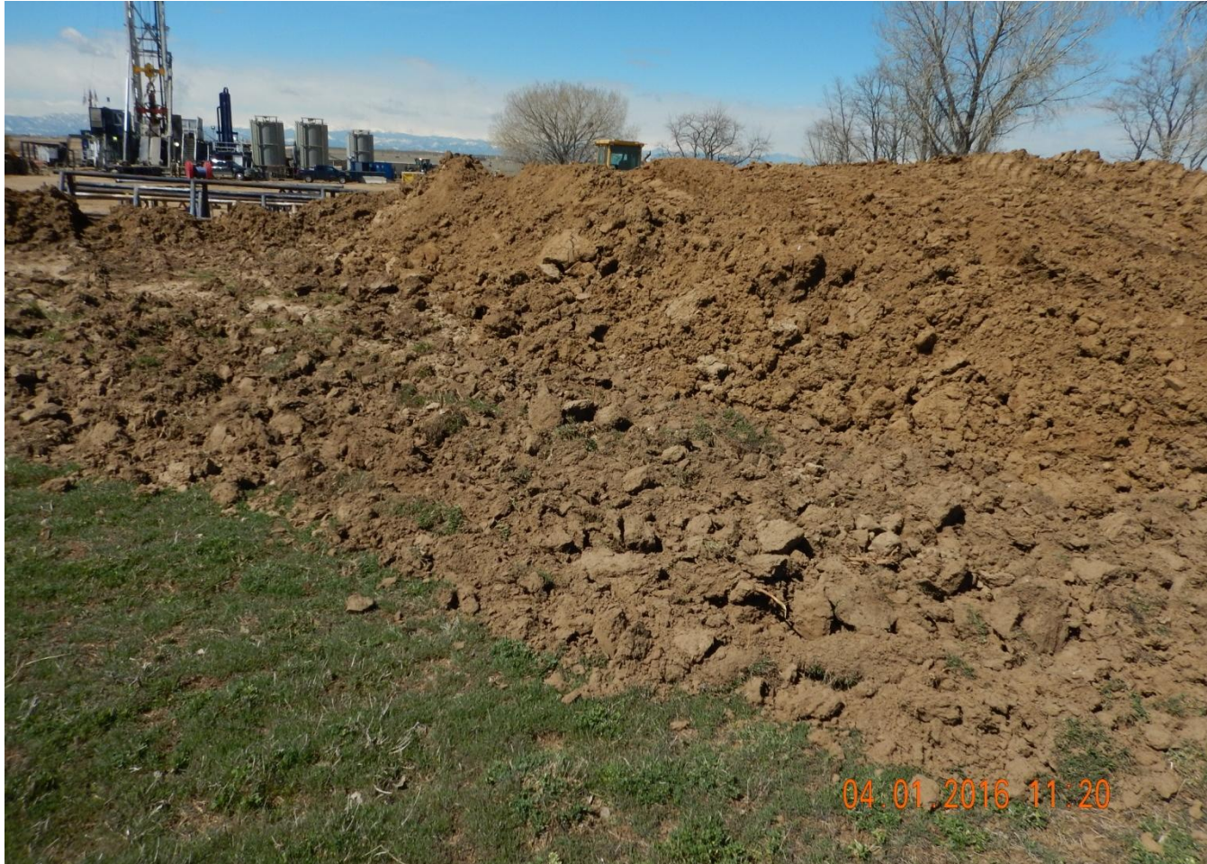
Photo 4. Photo taken from northeast Jacobucci well location, facing West. Need to stabilize perimeter of pad.
