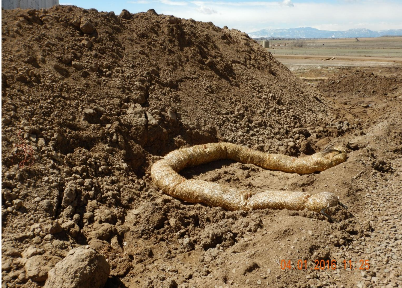
Photo 7. Photo taken from northwest Jacobucci well location, facing West. Need to stabilize perimeter of pad to prevent erosion off location.
