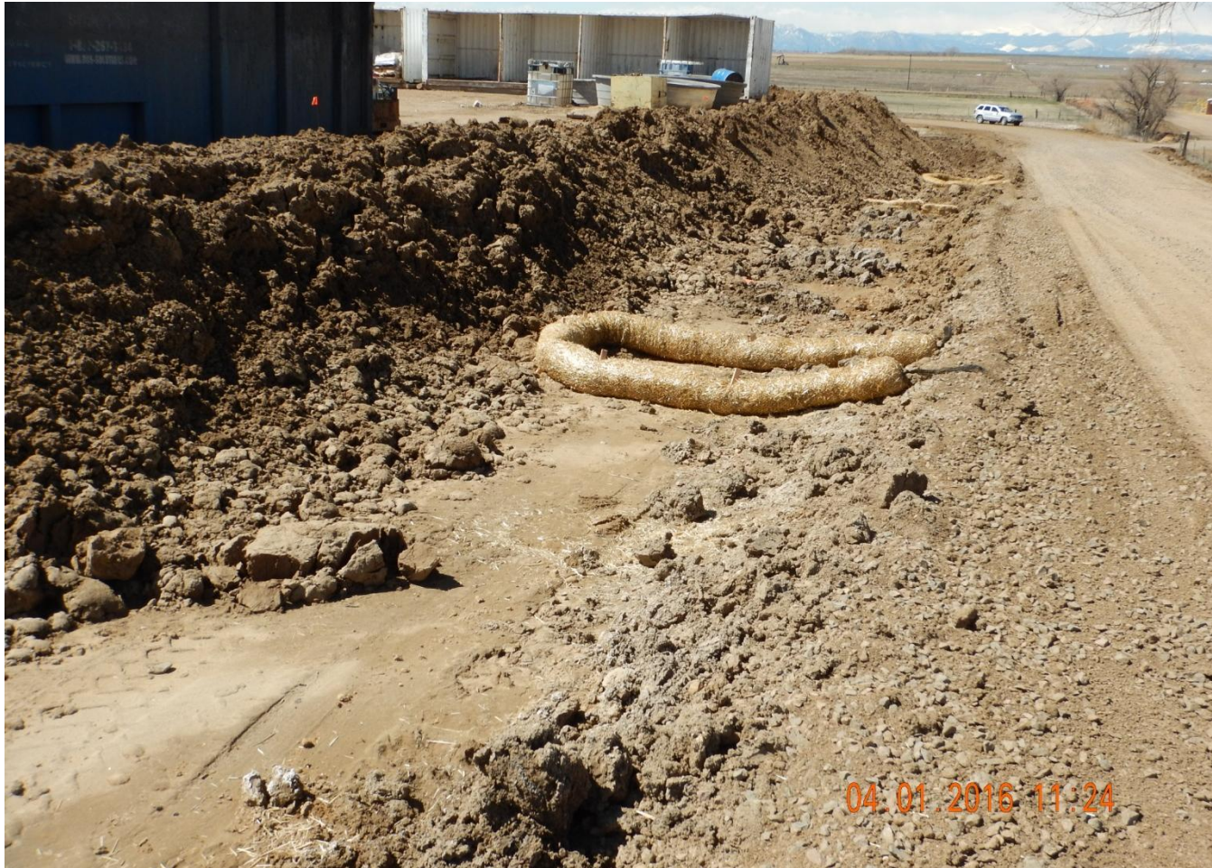
Photo 6. Photo taken from northern Jacobucci well location, facing West. Need to stabilize perimeter of pad to prevent erosion off location.
