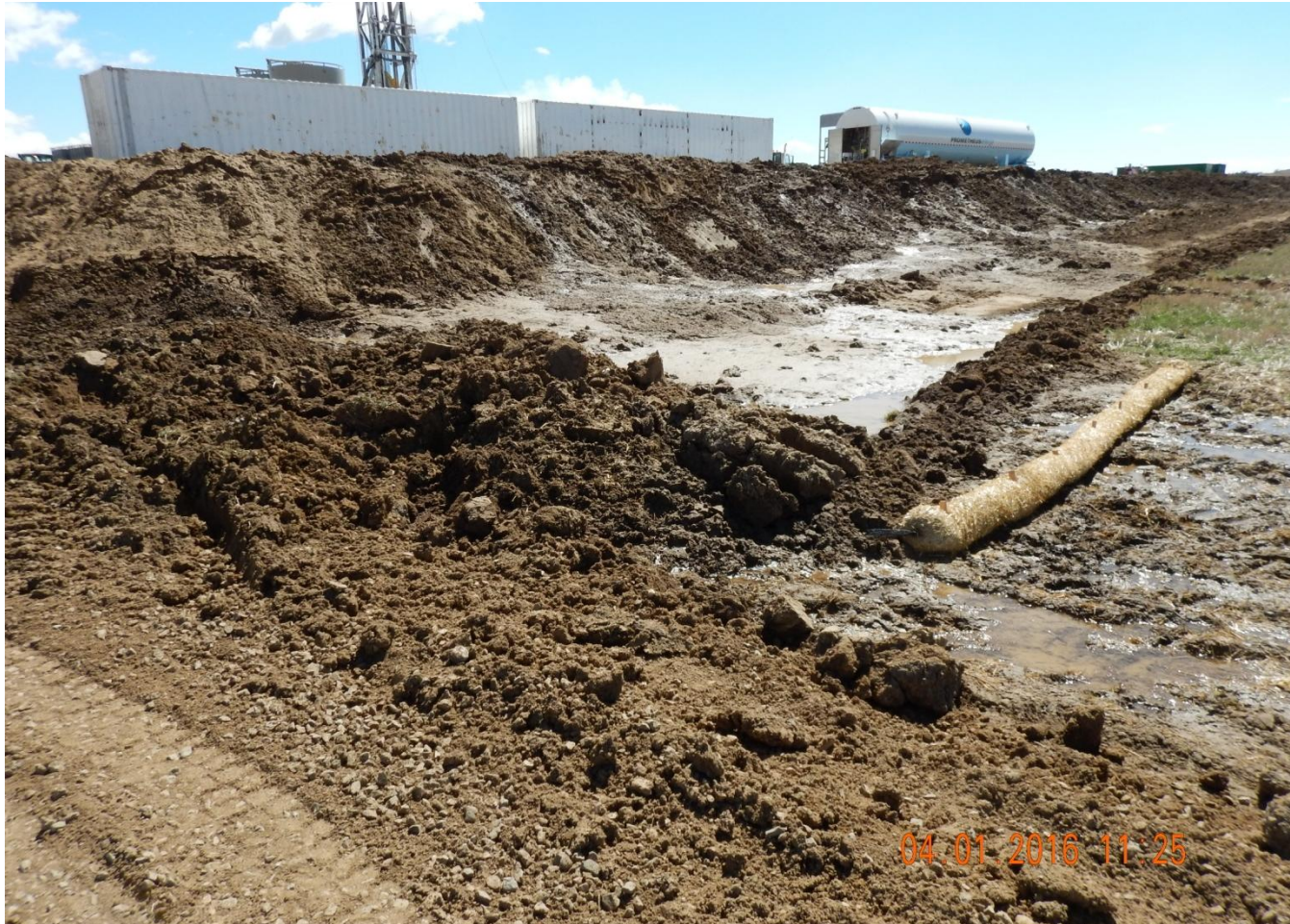
Photo 8. Photo taken from northwest Jacobucci well location, facing South. Need to stabilize perimeter of pad to prevent erosion off location.
