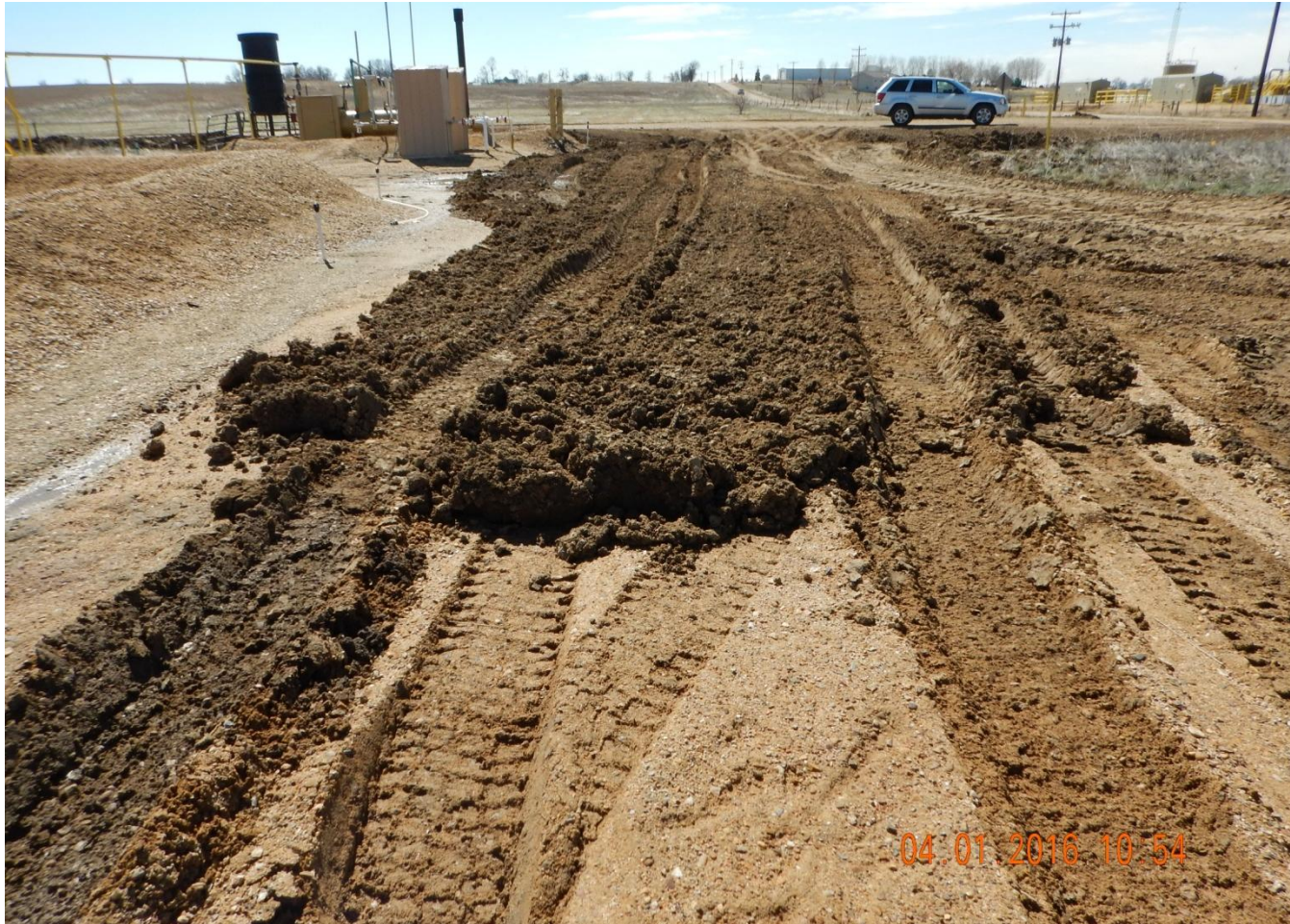
Photo 2. Photo taken from Jacobucci 13, 23-32 tank battery, facing South. Need to maintain location to prevent vehicle tracking and rutting.
