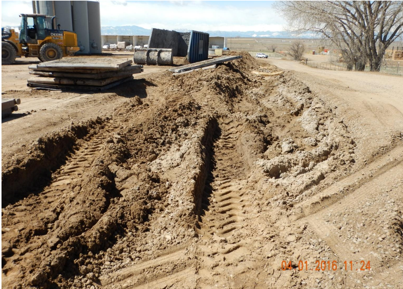
Photo 5. Photo taken from northern Jacobucci well location, facing West. Need to stabilize perimeter of pad to prevent erosion off location.
