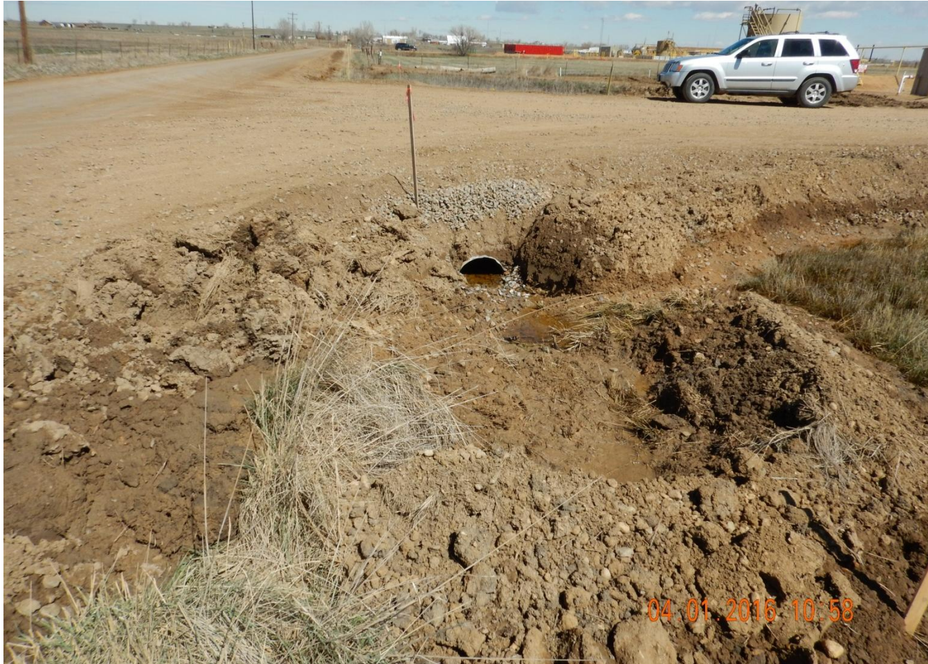
Photo 3. Photo taken from entrance of Jacobucci location, facing North. Need to maintain stormwater BMPs. Culvert is already half full.
