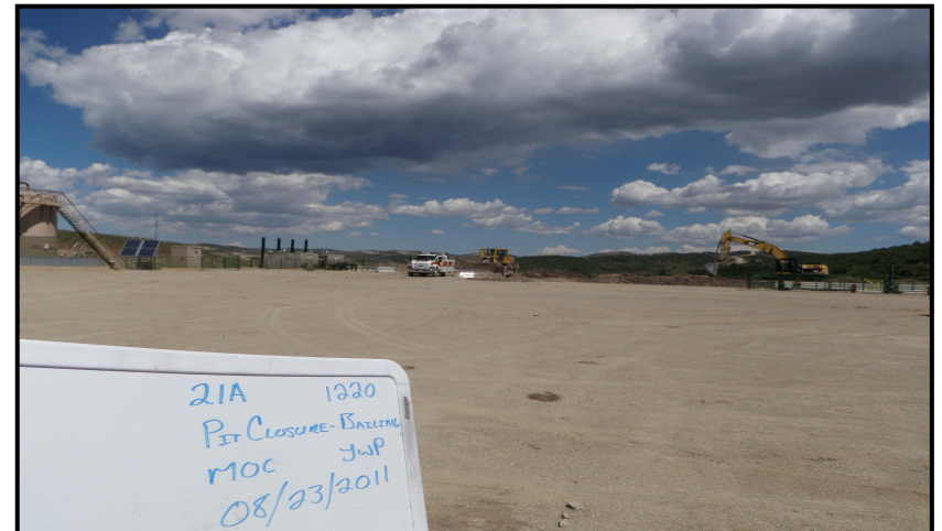
Photo 4 – Track hoe mixing pit contents with clean material within pit liner.
