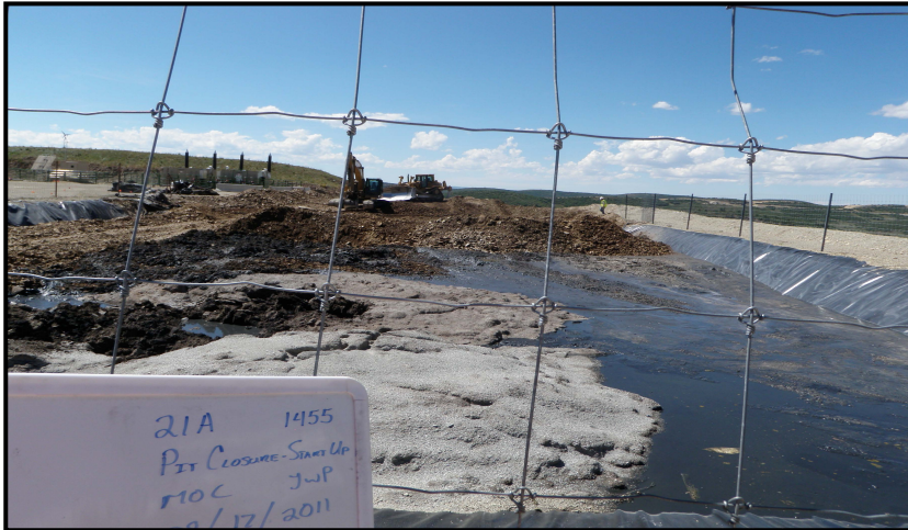
Photo 1 – 697-21A reserve pit containing drill cuttings with some fluids.
