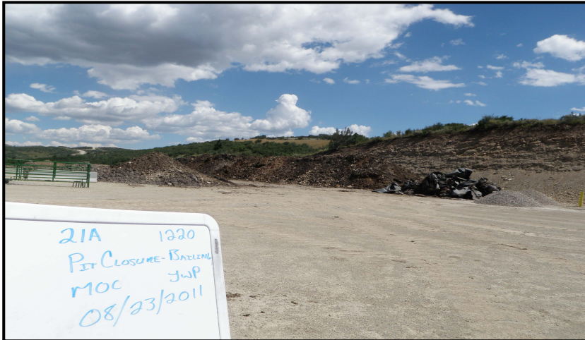
Photo 5 – Mixed material after being rolled with D8 and front end loader.
