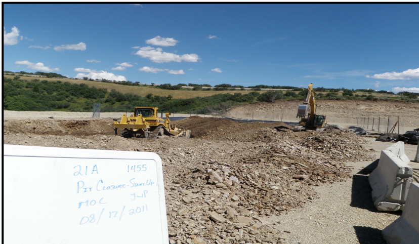
Photo 3 – D8 providing clean fill material from NW corner to track hoe for mixing.
