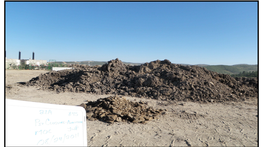
Photo 6 – Mixed material after being rolled with D8 and front end loader.
