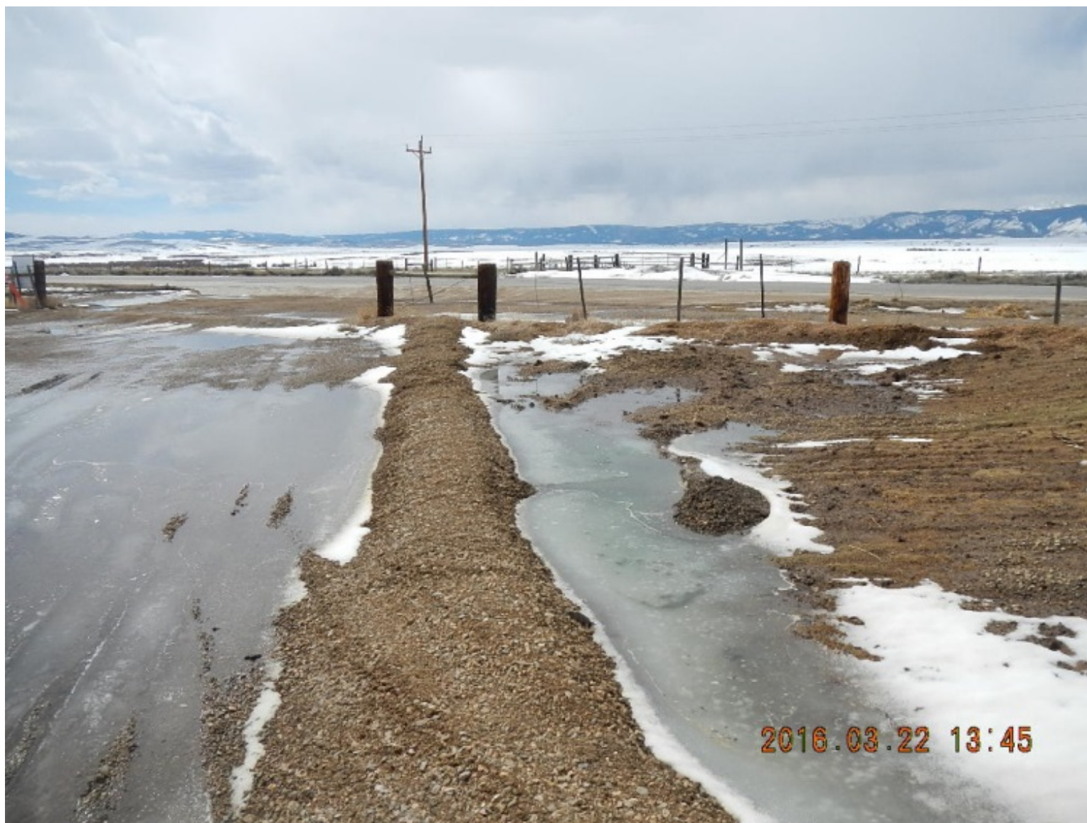
Picture 1A. Access to pad on left. Area where fluid is threatening to top berm on right
