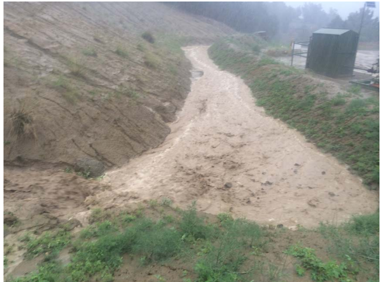
Figure 2: Stormwater flow in the North Diversion Channel. Rock RipRap located at the beginning of the North Diversion Channel is underwater. The RipRap prevented significant erosion. October 10, 2015.
