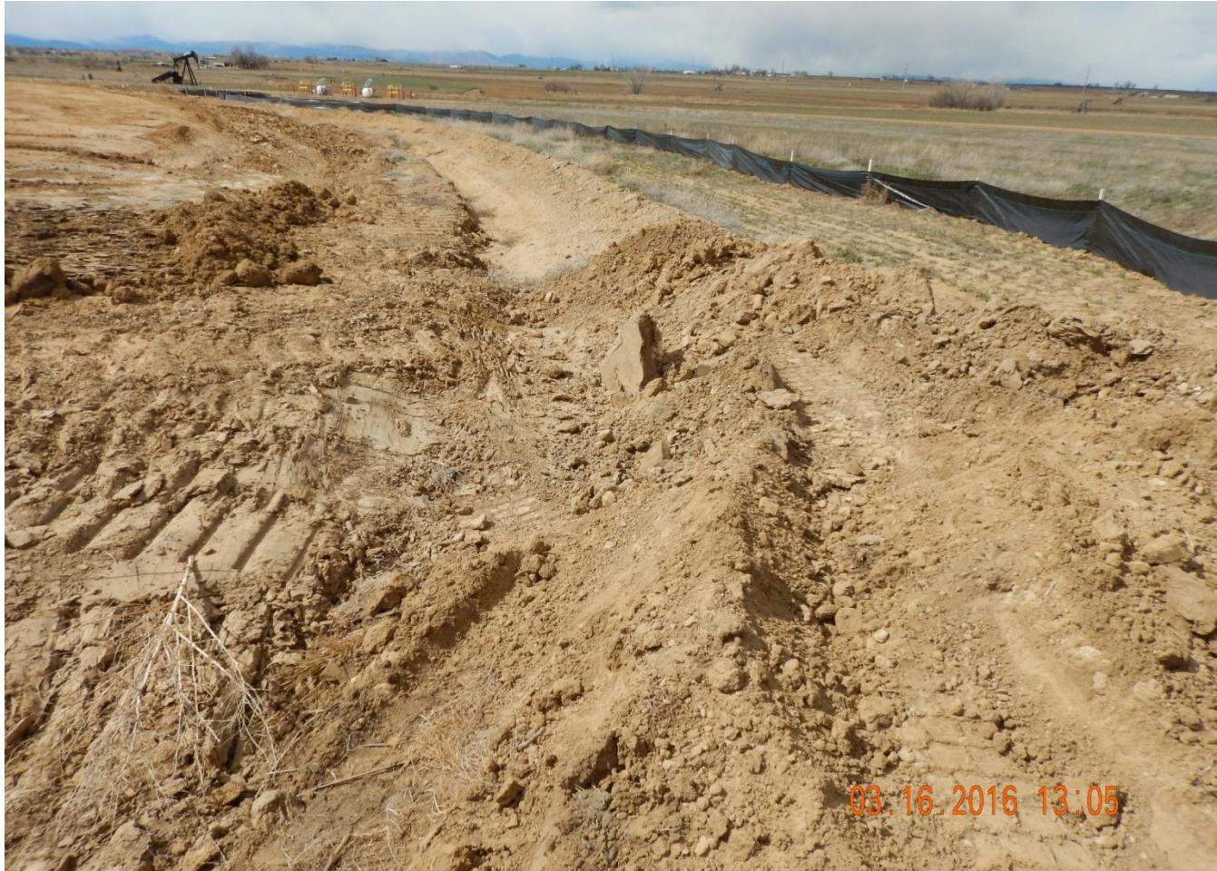
Photo 5. Photo taken from northeast location, facing West. Sediment control (silt fence) installed around perimeter of location.
