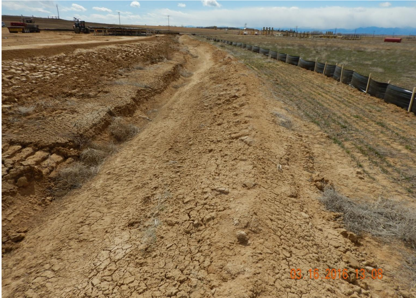
Photo 8. Photo taken from northwest location, facing South. Sediment control (silt fence) installed around perimeter of location.
