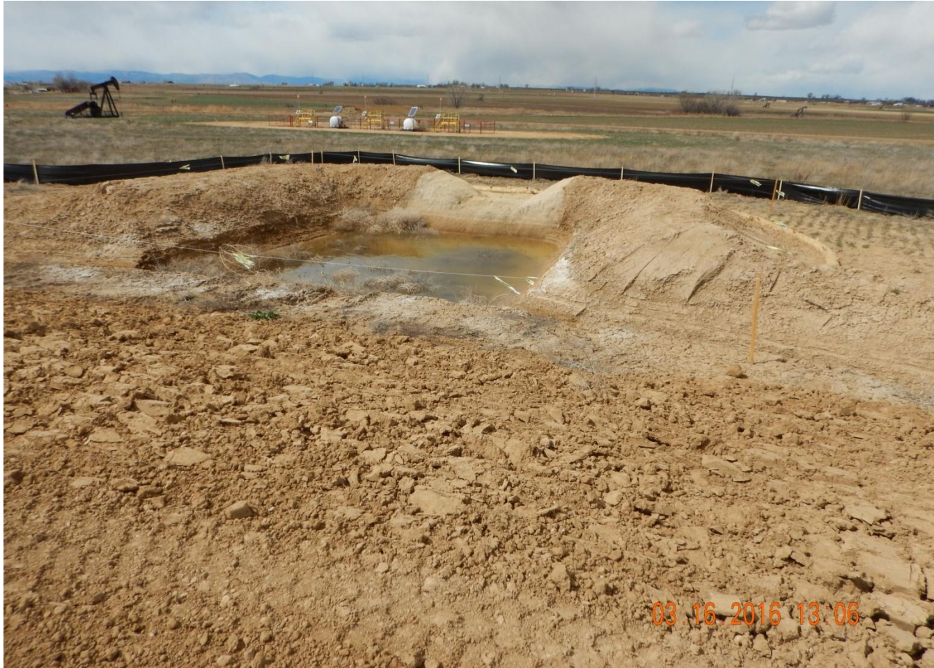
Photo 6. Photo taken from northern location, facing North. Stormwater and sediment control (sediment trap) installed at location low-point.
