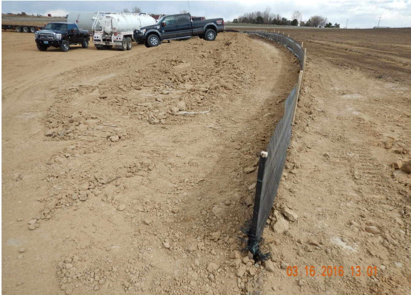
Photo 1. Photo taken from entrance of location, facing East. Sediment control (silt fence) installed around perimeter of location.
