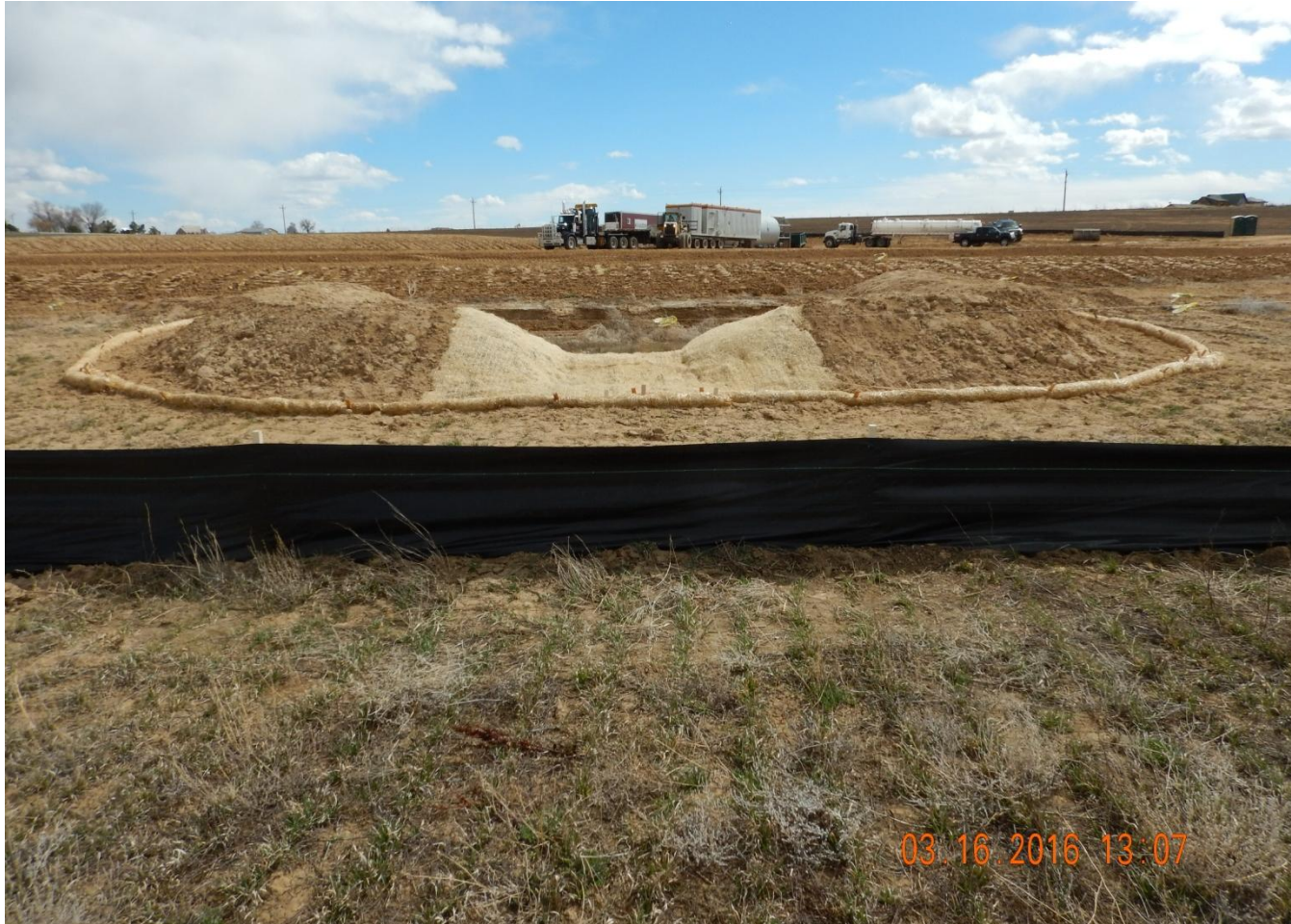
Photo 7. Photo taken from northern location, facing South. Stormwater and sediment control (sediment trap) installed at location low-point.
