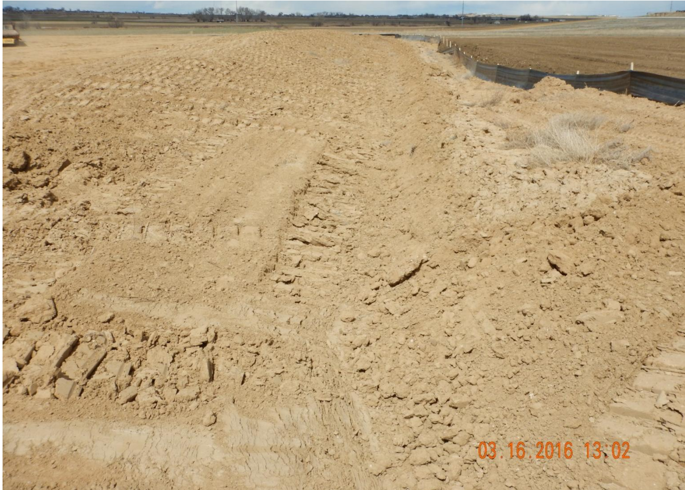
Photo 3. Photo taken from southeast location, facing North. Sediment control (silt fence) installed around perimeter of location.
