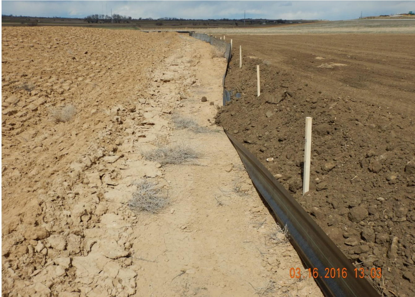
Photo 4. Photo taken from eastern location, facing North. Sediment control (silt fence) installed around perimeter of location. Need to inspect and maintain silt fence frequently.
