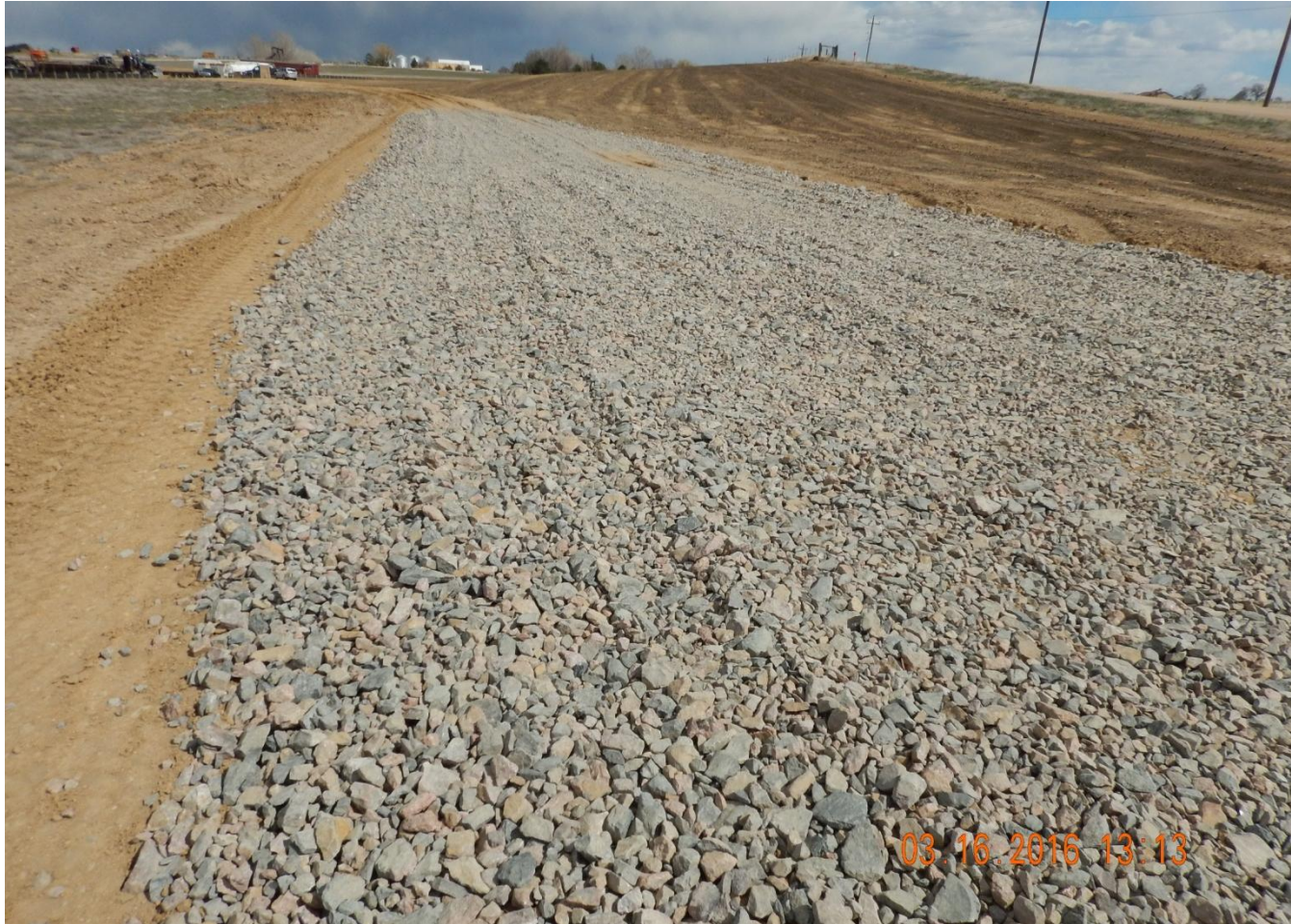
Photo 9. Photo taken from entrance of location, facing Northeast. Vehicle tracking pad installed to minimize sediment leaving location.
