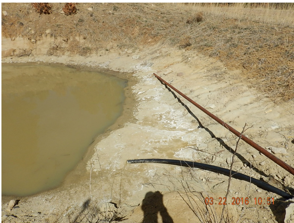
Figure 4 – Piping from wellhead to pit. Metal pipe is disconnected.
