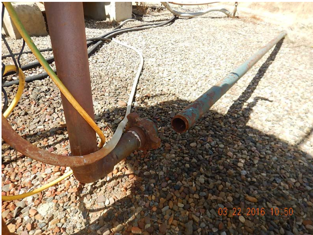
Figure 3 – Pipe to pit is currently disconnected.
