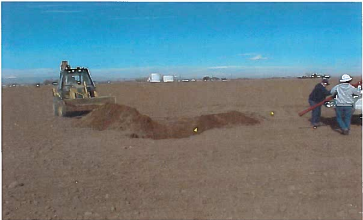
Photo 6 – Looking northwest at backhoe filling test pit 2 with excavated soil after completing assessment.
