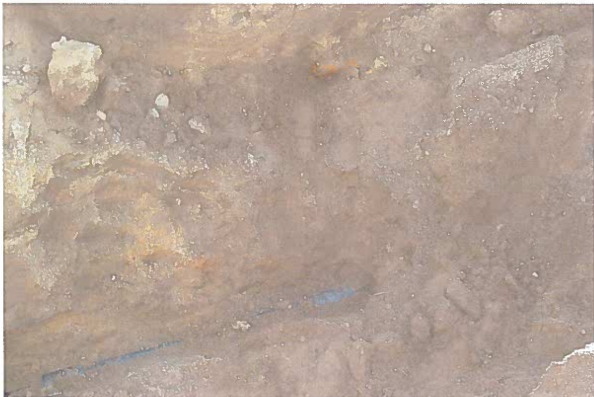
Photo 4 – Looking into test pit 1 at 3-inch DEFS line (bottom) under 2-inch flow line (top).
