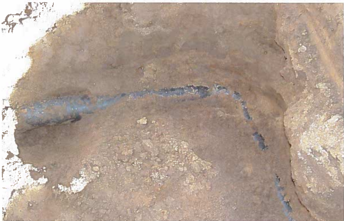
Photo 2 – Looking into test pit 1 at 90 degree elbow where DEFS line changes from 3-inch to 4-inch. No staining or odors observed under line or connections.
