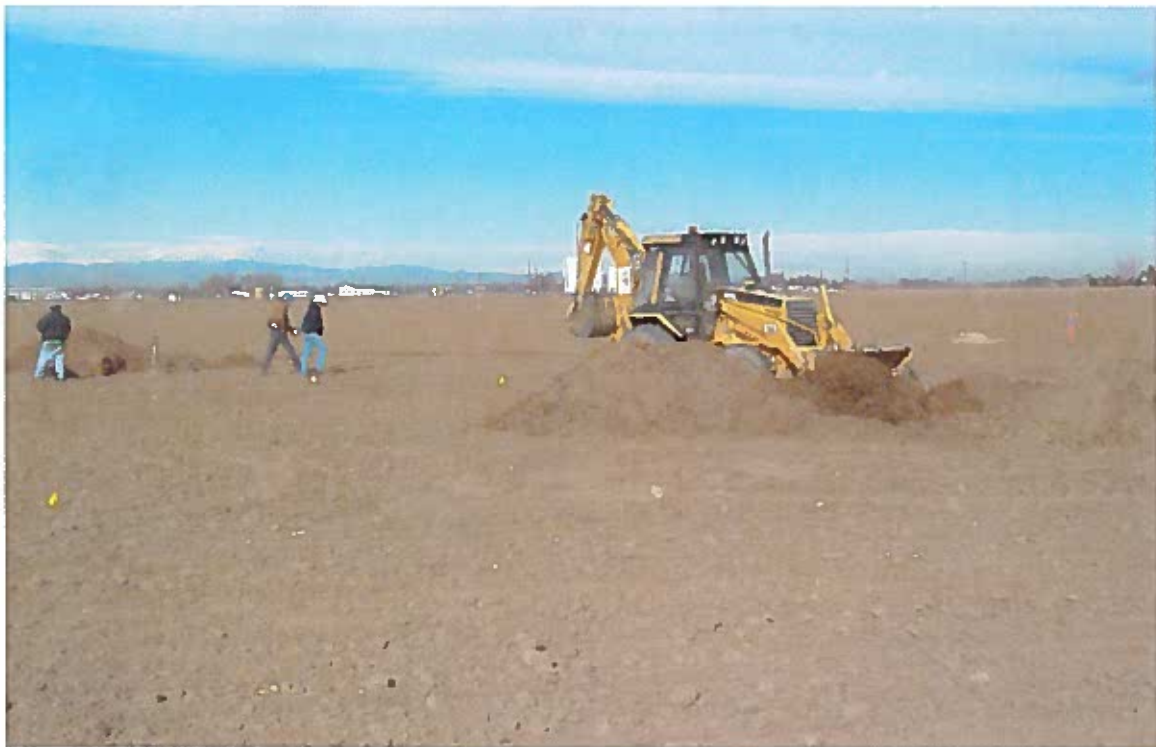
Photo 1 – Looking northwest at test pit 1 (right), test pit 2 (left), and the test boring (right background by orange stake) that encountered hydrocarbon-impacted soil at 19 feet bgs.
