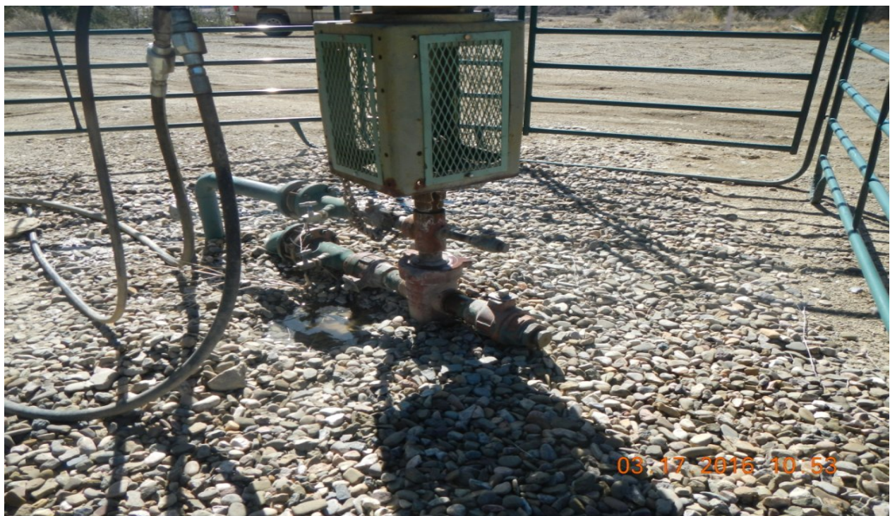
photo 4: Noticed a dripping water leak at the well head.
