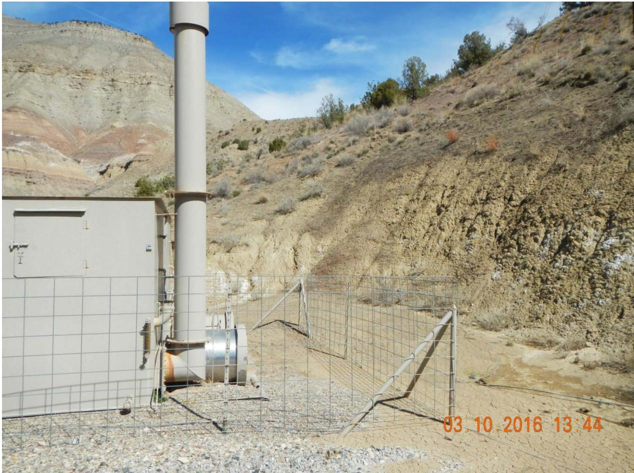
Slope wall used as berm wall allowing storm water inside of berm. Berm walls unmaintained.
