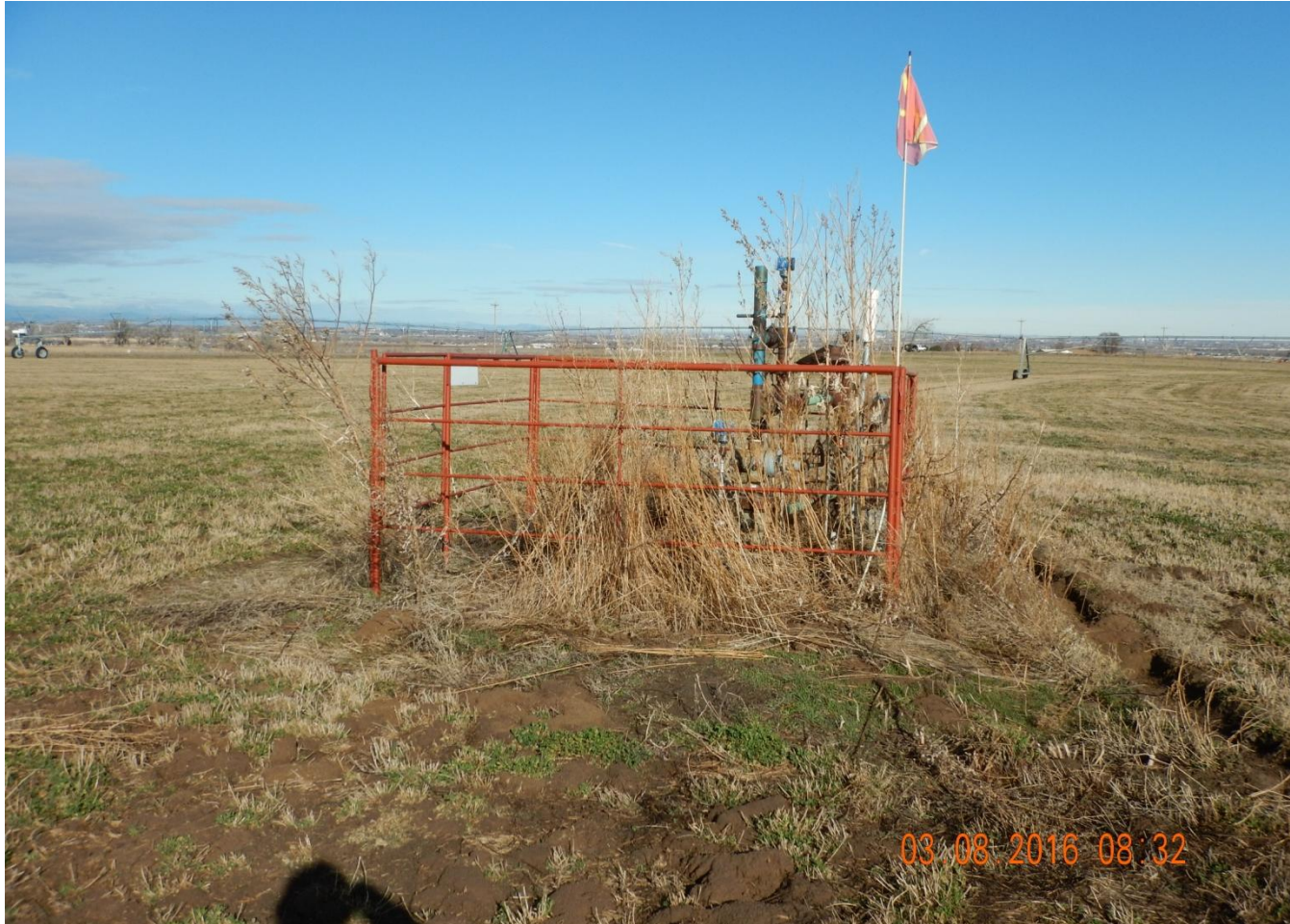
Photo 3. Photo taken from south of location, facing North. Remove weeds around wellhead. Weeds within 25 feet of operating oil and gas equipment are a potential safety or fire concern.
