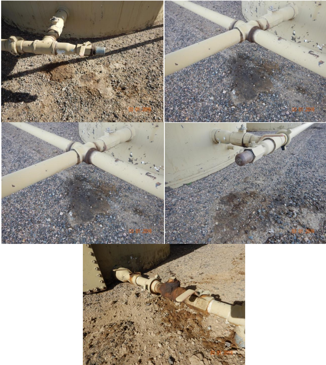
Figure 5 - Localized oil-stained/saturated soil beneath various pipe fittings around the tank battery.
