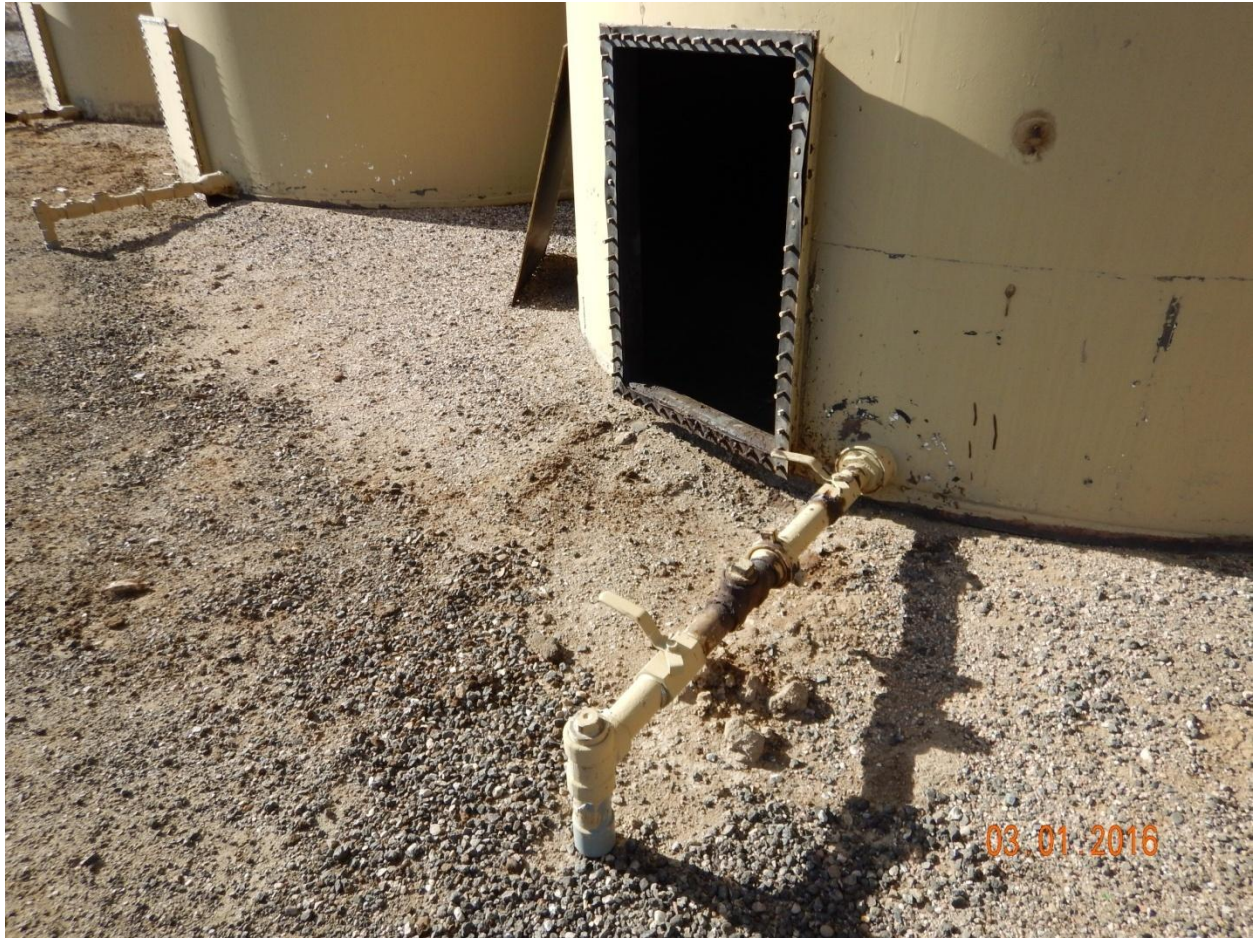
Figure 6 - Open access panel, leaking pipe fittings, and stained soil at south produced water tank.
