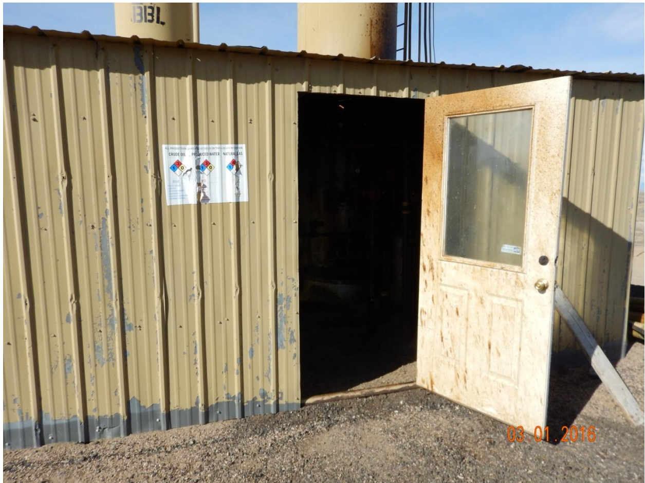
Figure 9 - Oil-staining inside door to separator shed.
