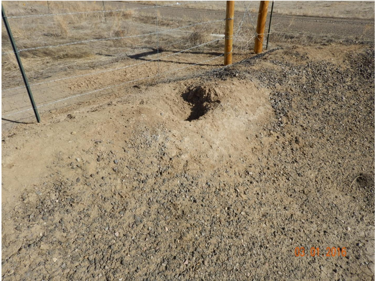
Figure 3 – Damage to berm at northwest corner of tank battery.
