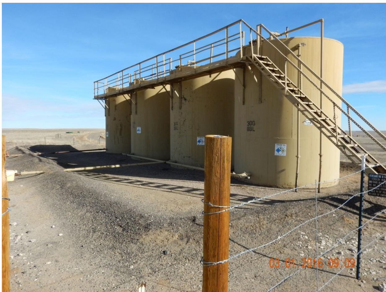
Figure 2 - Steel ASTs at tank battery, earthen berm appears to be too shallow/eroded to provide adequate containment volume.
