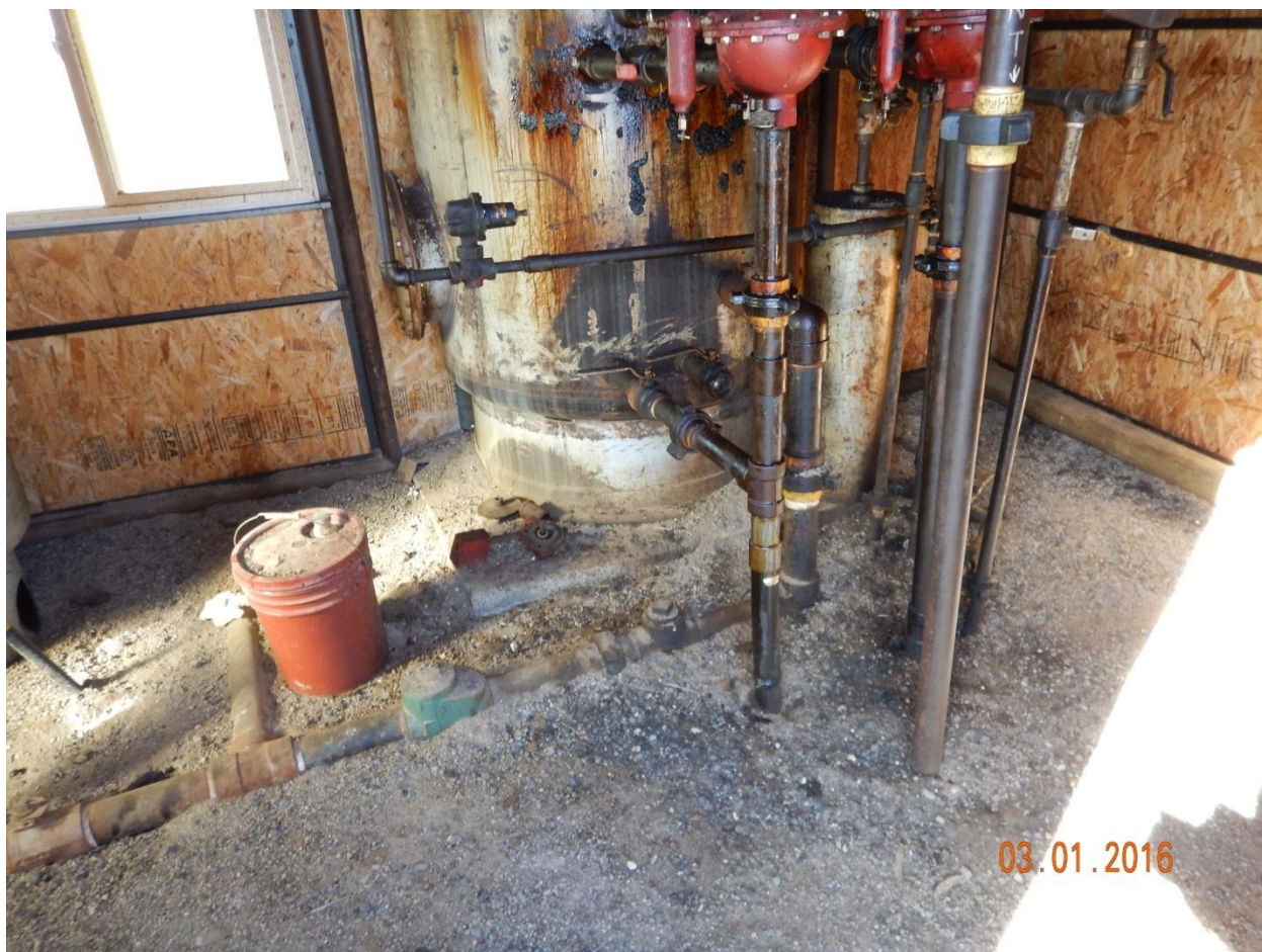
Figure 10 - Oil-stained soil and equipment (and unlabeled bucket) inside of separator shed.
