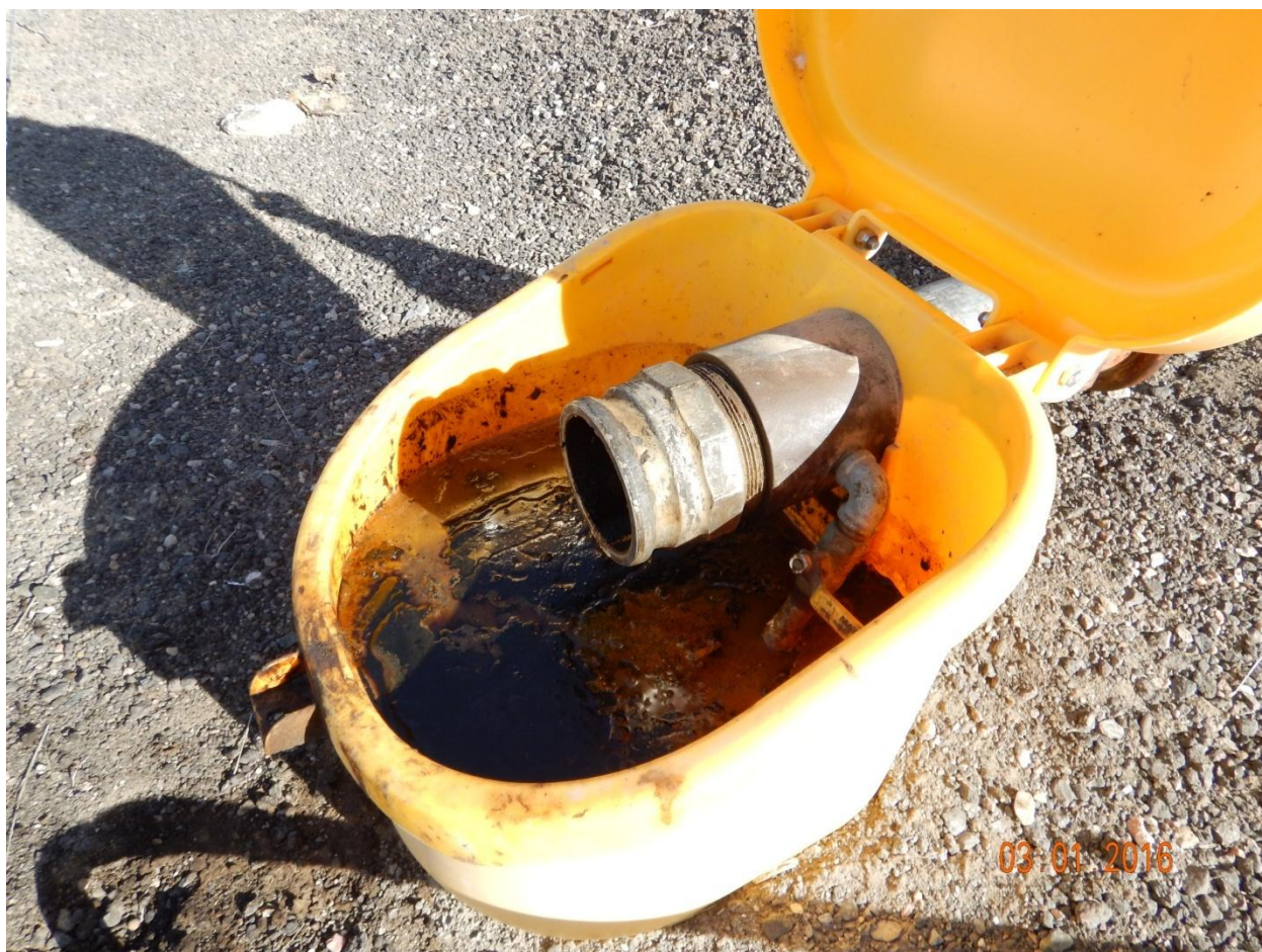
Figure 4 - North tank loadout within 1-2" of overflowing with crude oil. Oil should be removed and properly disposed of during routine maintenance to prevent a spill.
