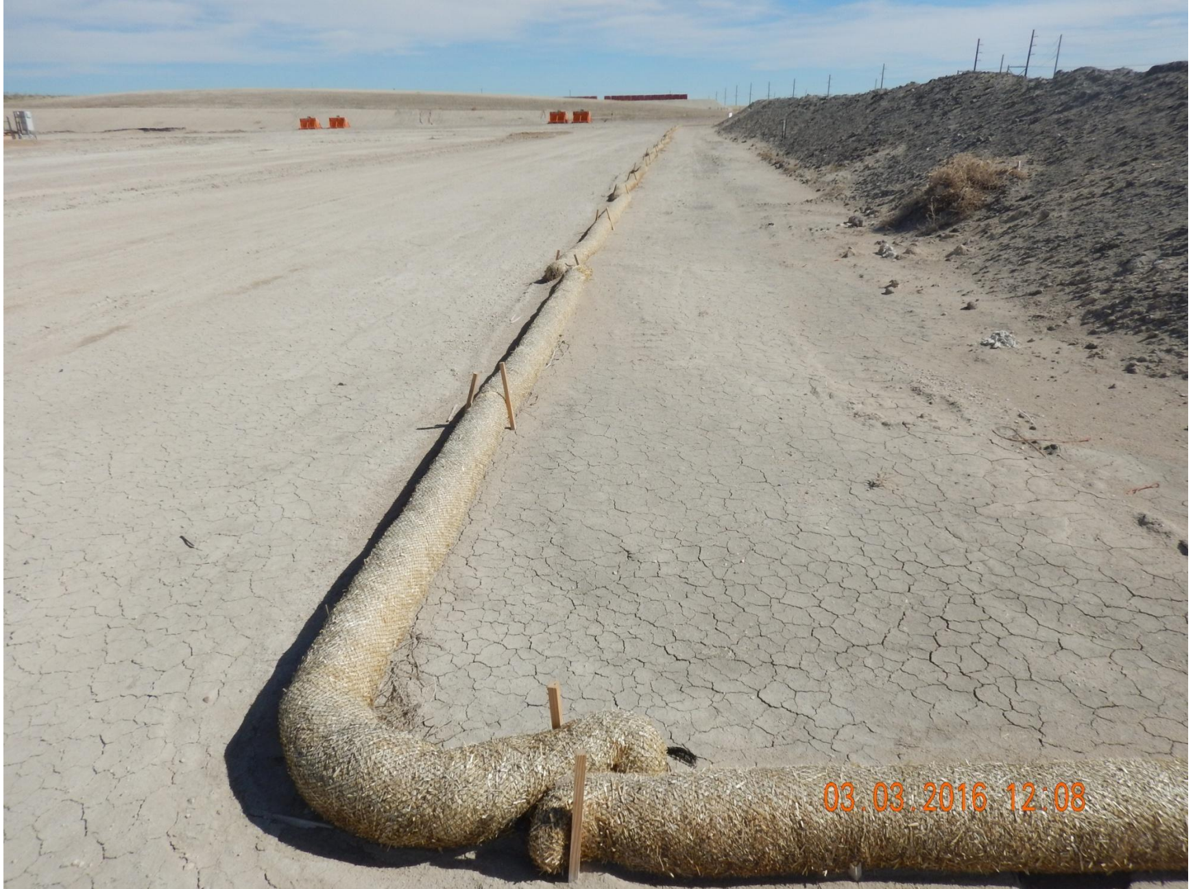
Figure 40: Photo taken from the southwestern end of location, facing east. Photo of straw wattles used as a stormwater and sediment control BMP around drill cuttings.
