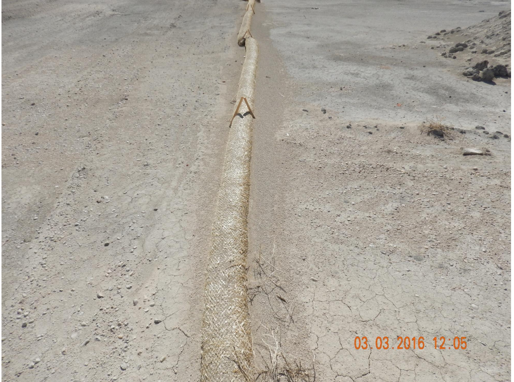
Figure 38: Photo taken from the south east end of project area. Photo shows straw wattle used as a sediment control BMP filled in with sediment. Will require cleaning or replacement in order to function properly.
