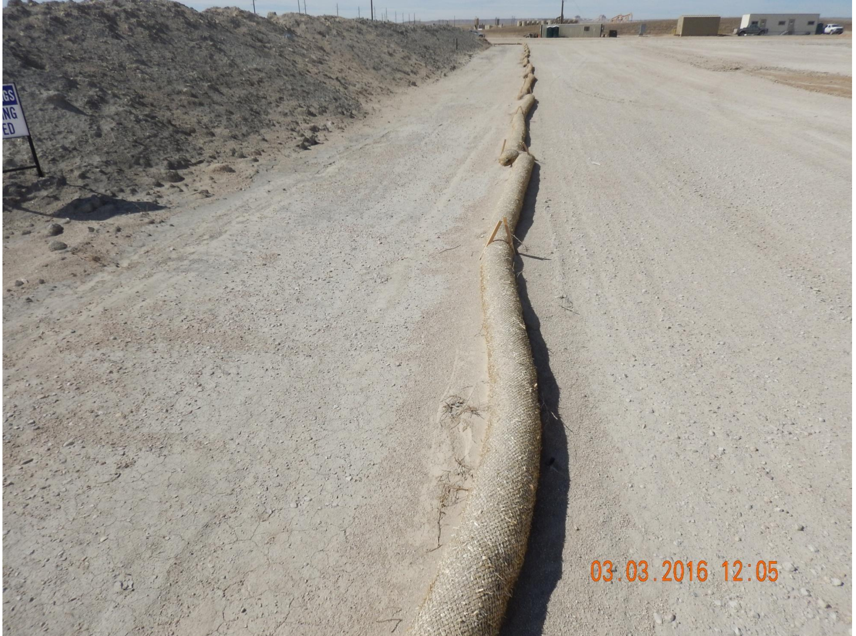
Figure 39: Photo taken from the southeast end of location, facing west. Photo of straw wattles used as a stormwater and sediment control BMP around drill cuttings
