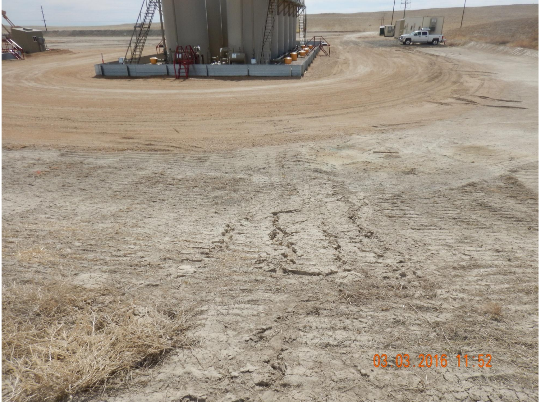
Figure 14: Photo taken from the north end of the location, facing south. Photo show rill erosion on slope.
