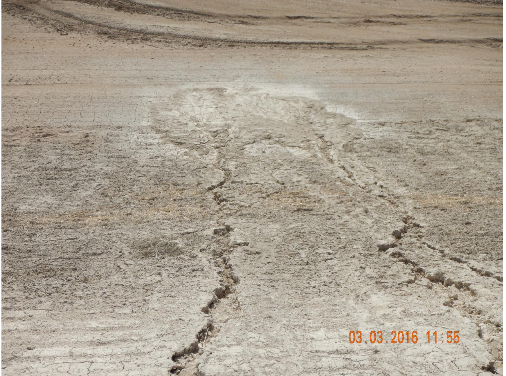
Figure 18: Photo taken from the north end of the location, facing south. Photo of rill erosion on slope, and sediment deposition on location. It appears rill erosion originates from the stormwater control ditch.
