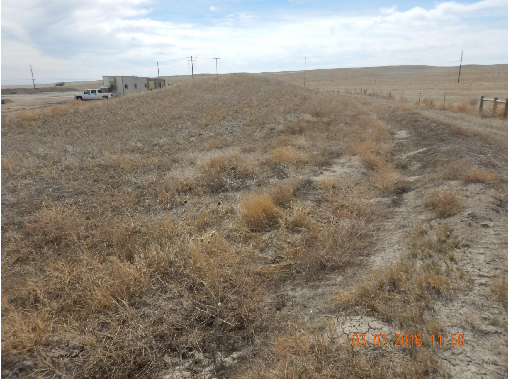
Figure 9: Photo taken the northwest end of location, facing south. Photo shows topsoil berm center of photo, stormwater and sediment control ditch to the right, and western interim area.
