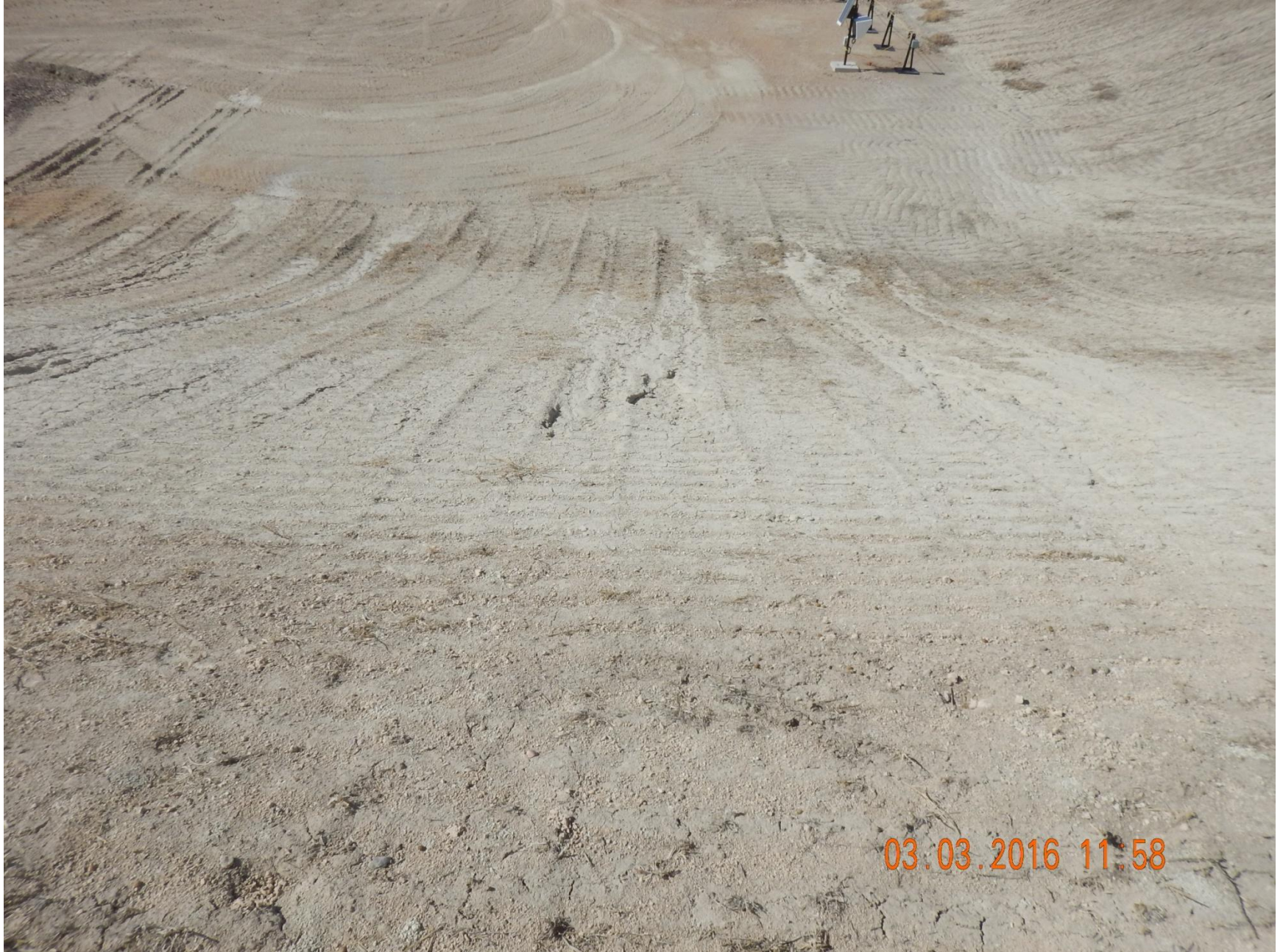
Figure 24: Photo taken from the northeast end of the location, facing west. Photo shows rill erosion and sediment deposition on slope.
