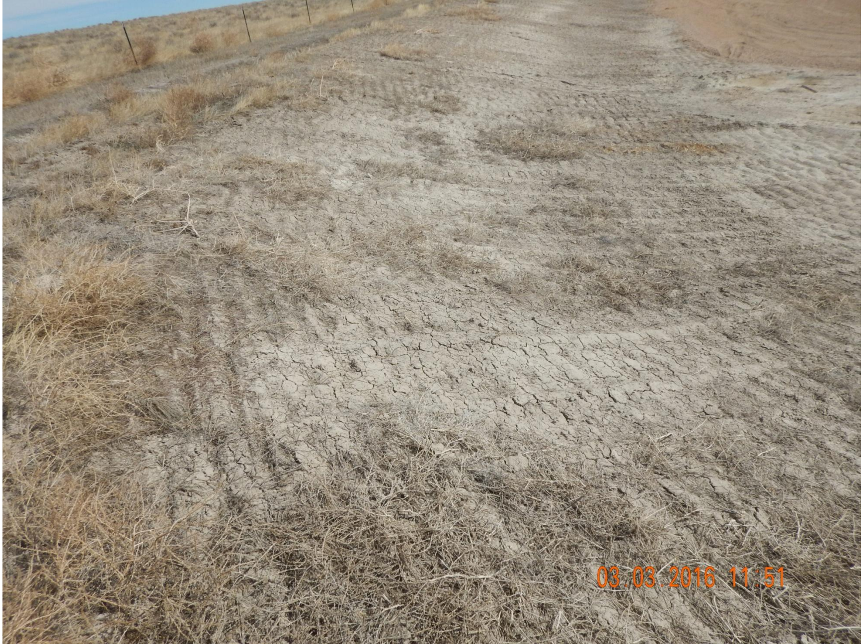
Figure 11: Photo taken from the northwest corner of project area. Photo shows vehicle tracking used as a stormwater and sediment control BMP.
