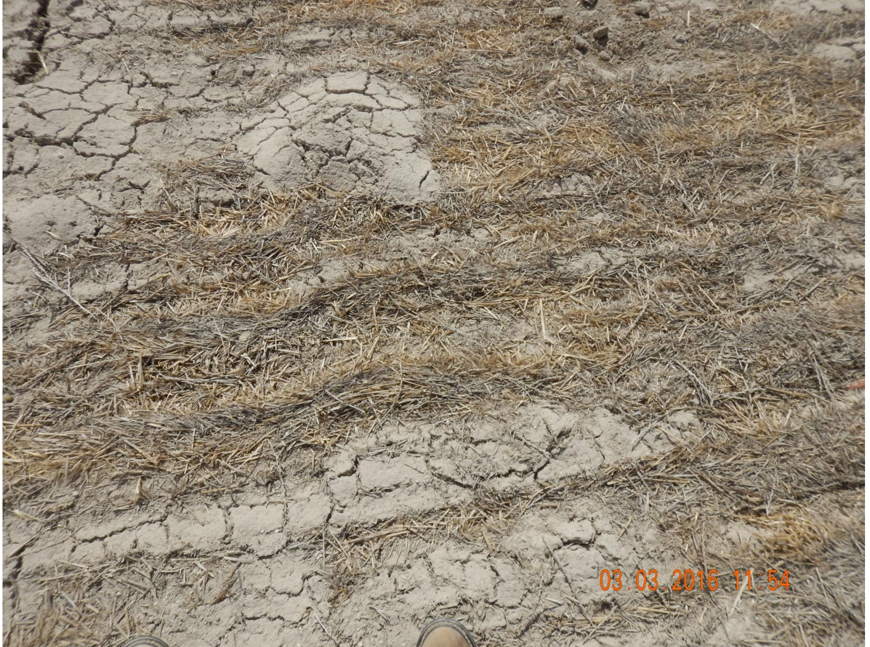
Figure 16: Photo taken from the north end of the location. Photo shows straw mulch crimped into slope.
