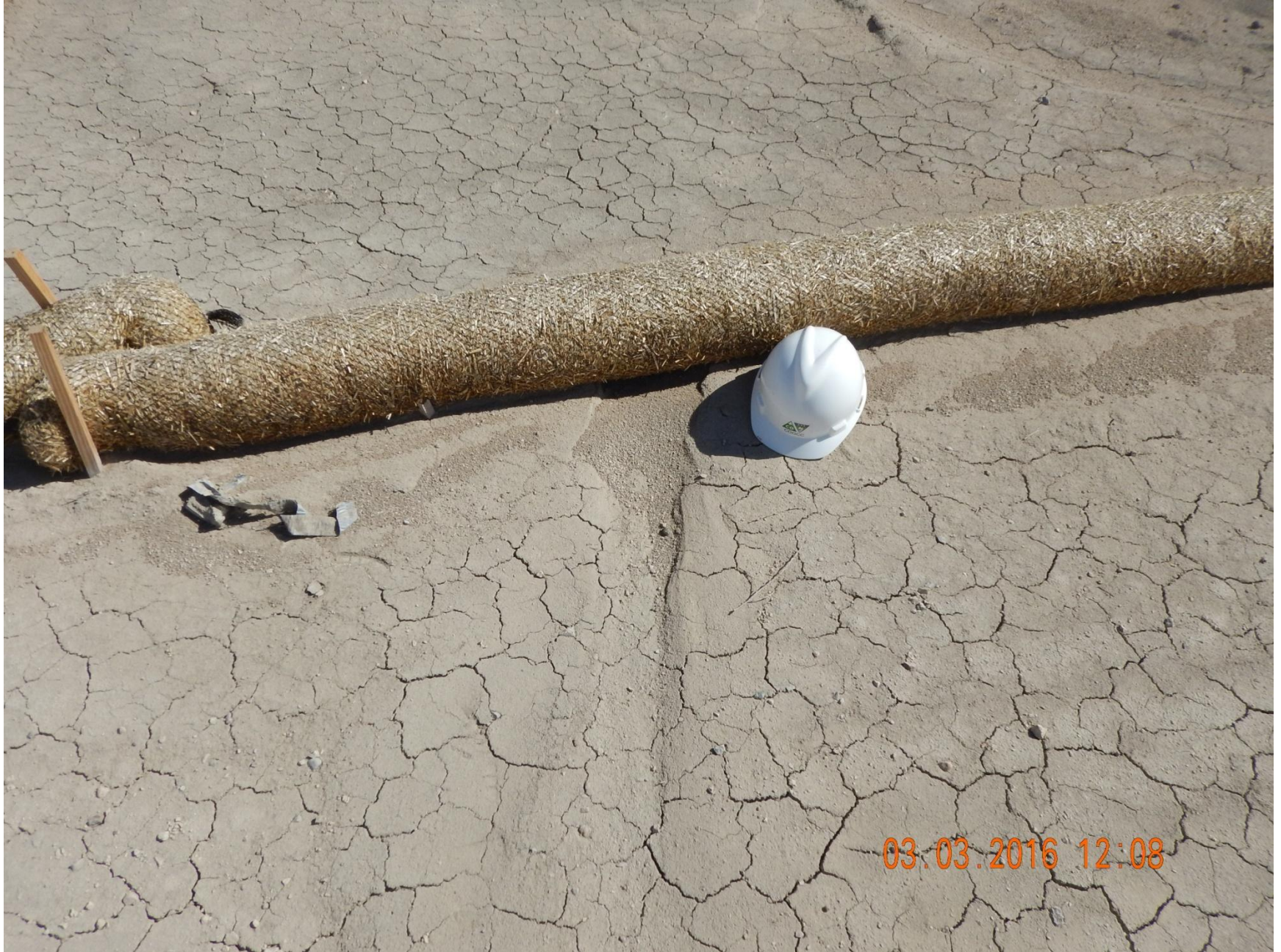
Figure 41: Photo taken from the southwestern end of location, facing east. Photo of straw wattles used as a stormwater and sediment control BMP not in proper functioning condition. Photo shows stormwater and sediment travel beneath the straw wattle.
