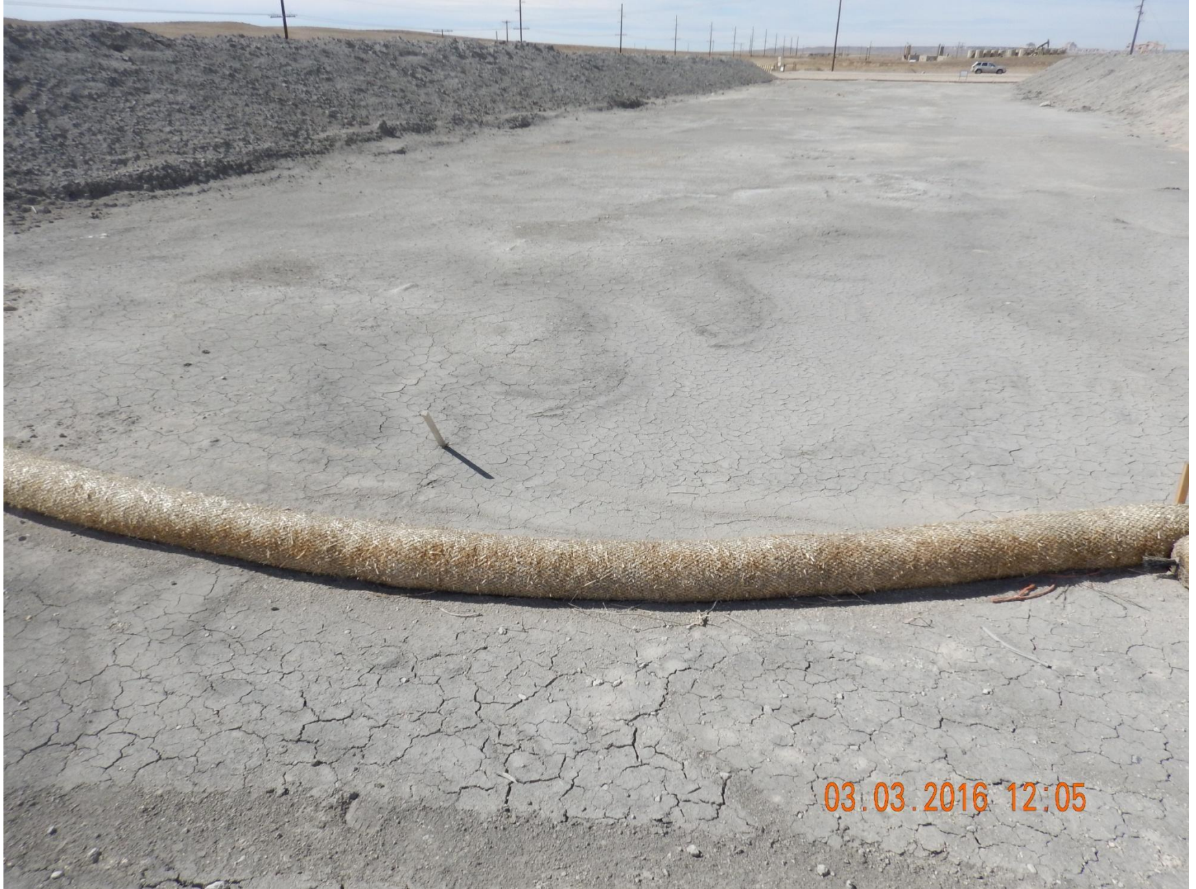
Figure 37: Photo taken from the southeast end of location, facing west. Photo shows straw wattle not in proper functioning condition.
