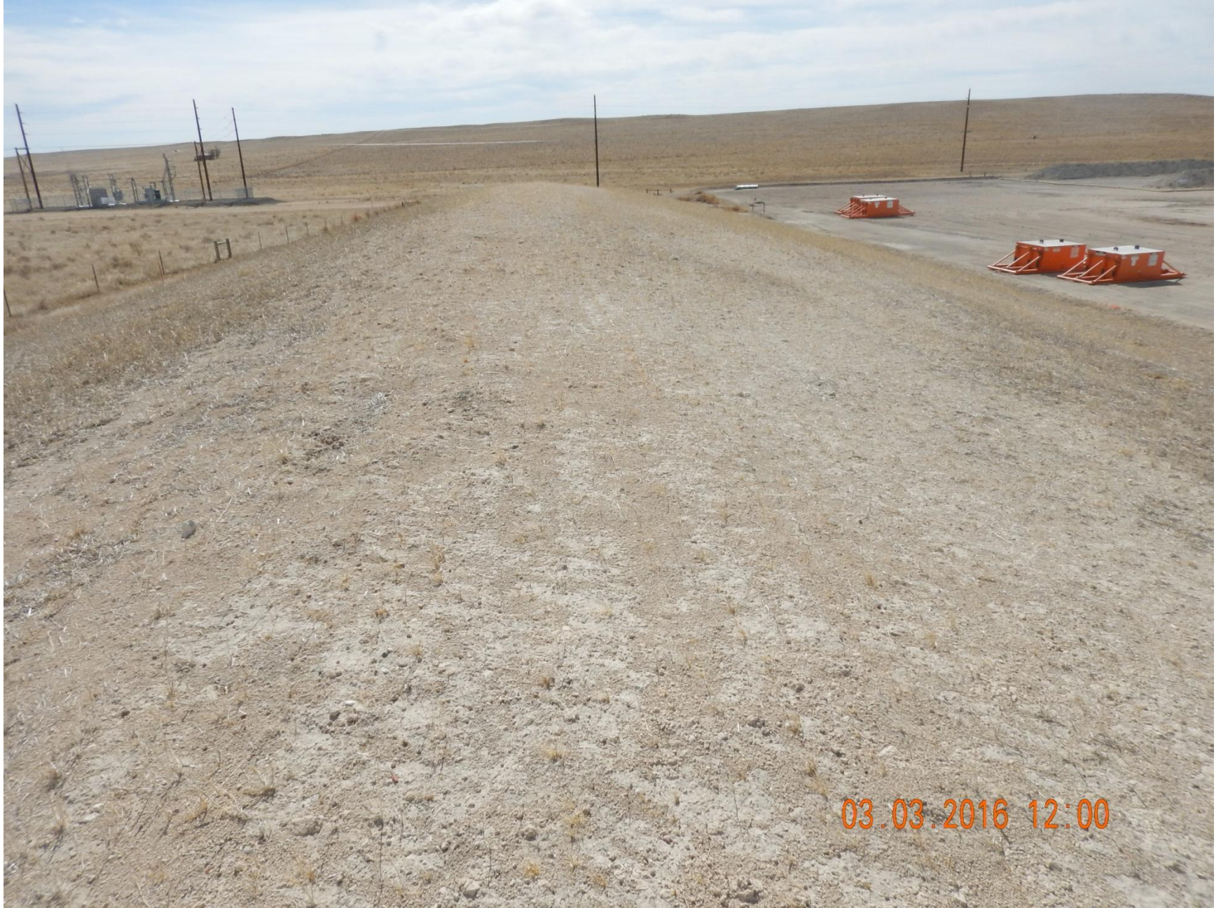
Figure 27: Photo taken from the east end of the project area, facing south. Photo shows portion of the interim lacking uniform vegetation. Note the left and right side of the photo shows vegetative growth.
