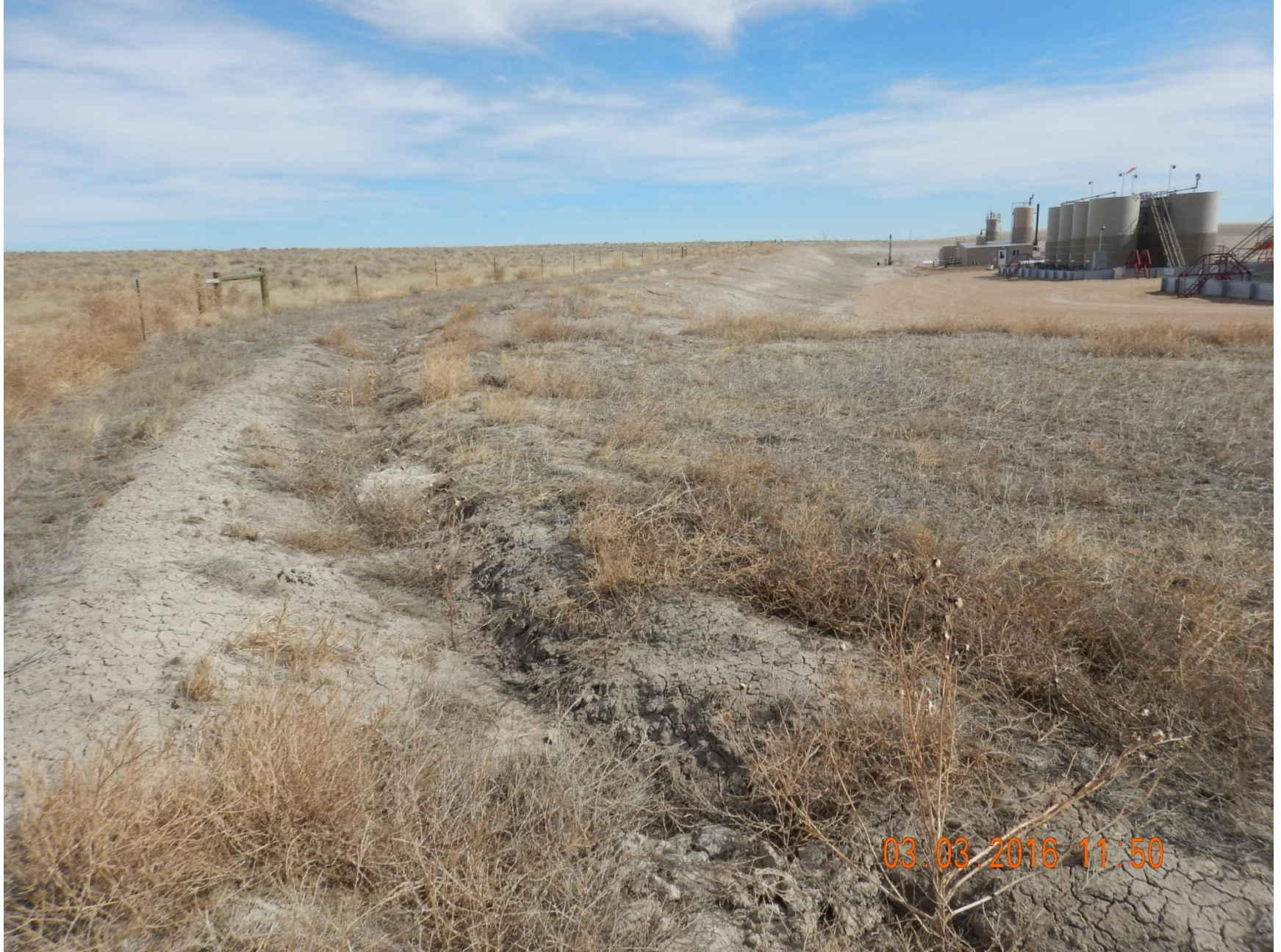
Figure 10: Photo taken the northwest end of location, facing northeast. Photo shows stormwater and sediment control ditch and the northern interim area.
