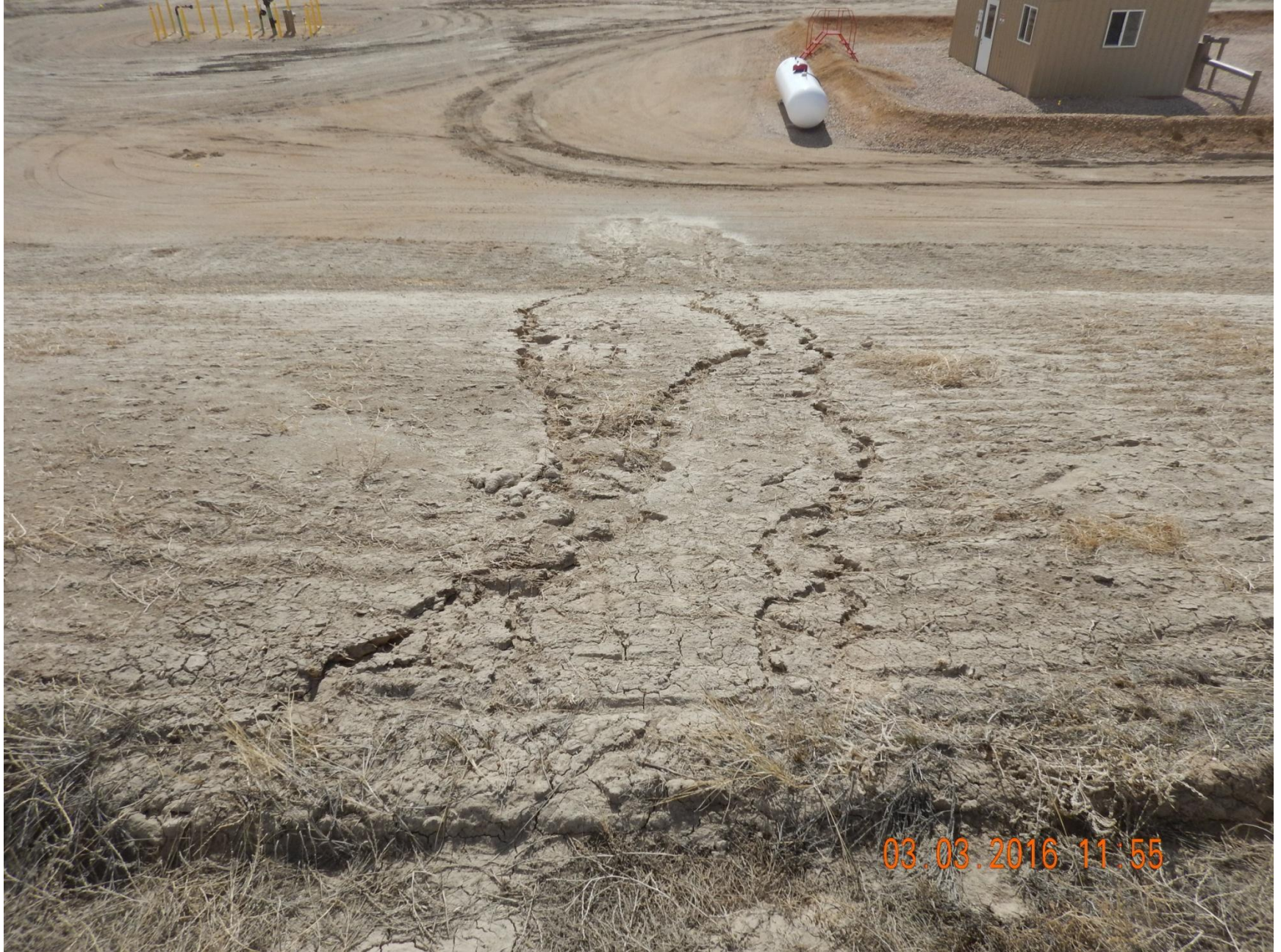
Figure 17: Photo taken from the north end of the location, facing south. Photo of rill erosion on slope, and sediment deposition on location. It appears rill erosion originates from the stormwater control ditch.
