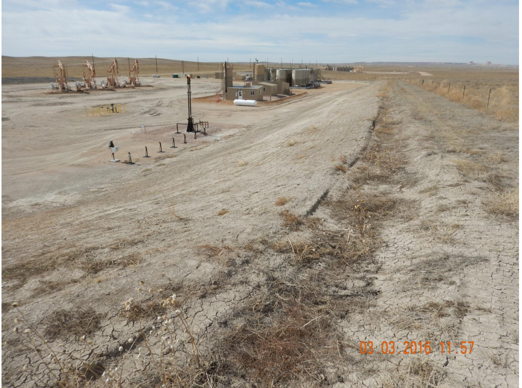
Figure 22: Photo taken from the northeast end of location, facing west. Photo shows project and interim areas, and stormwater and sediment control ditch on northern perimeter.
