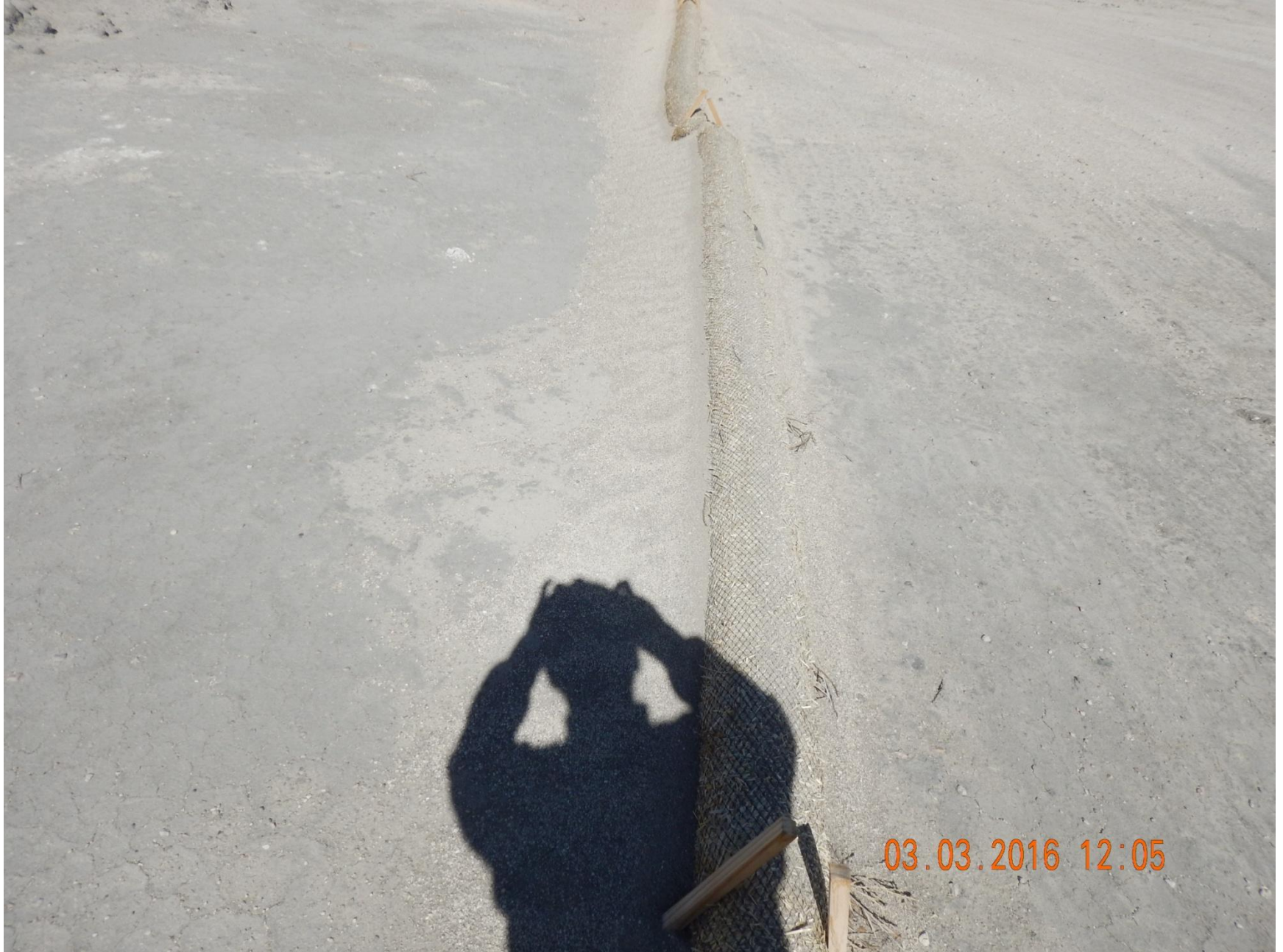
Figure 36: Photo taken from the south east end of project area. Photo shows straw wattle used as a sediment control BMP filled in with sediment. Will require cleaning or replacement in order to function properly.
