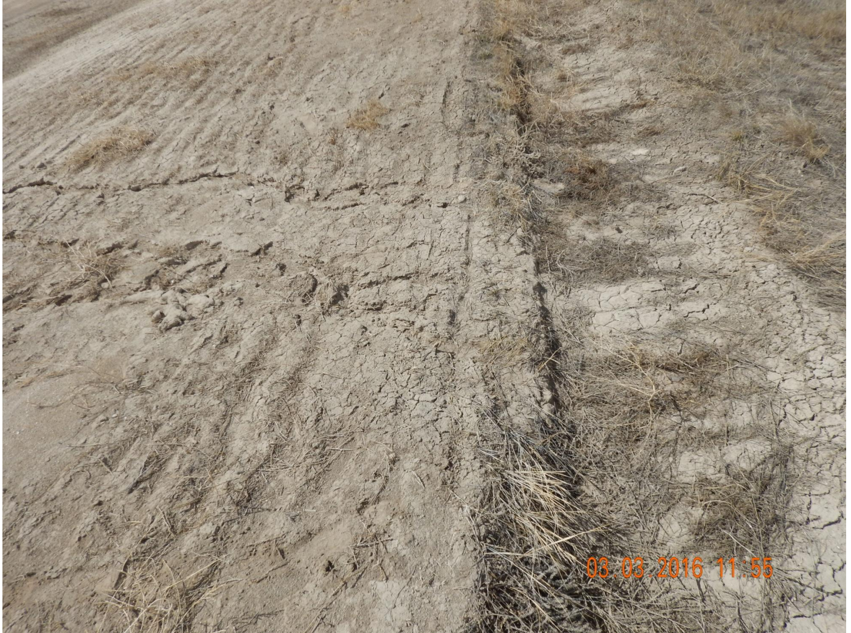
Figure 19: Photo taken from the north end of the location. Photo of rill erosion on slope. It appears rill erosion originates from the stormwater control ditch.
