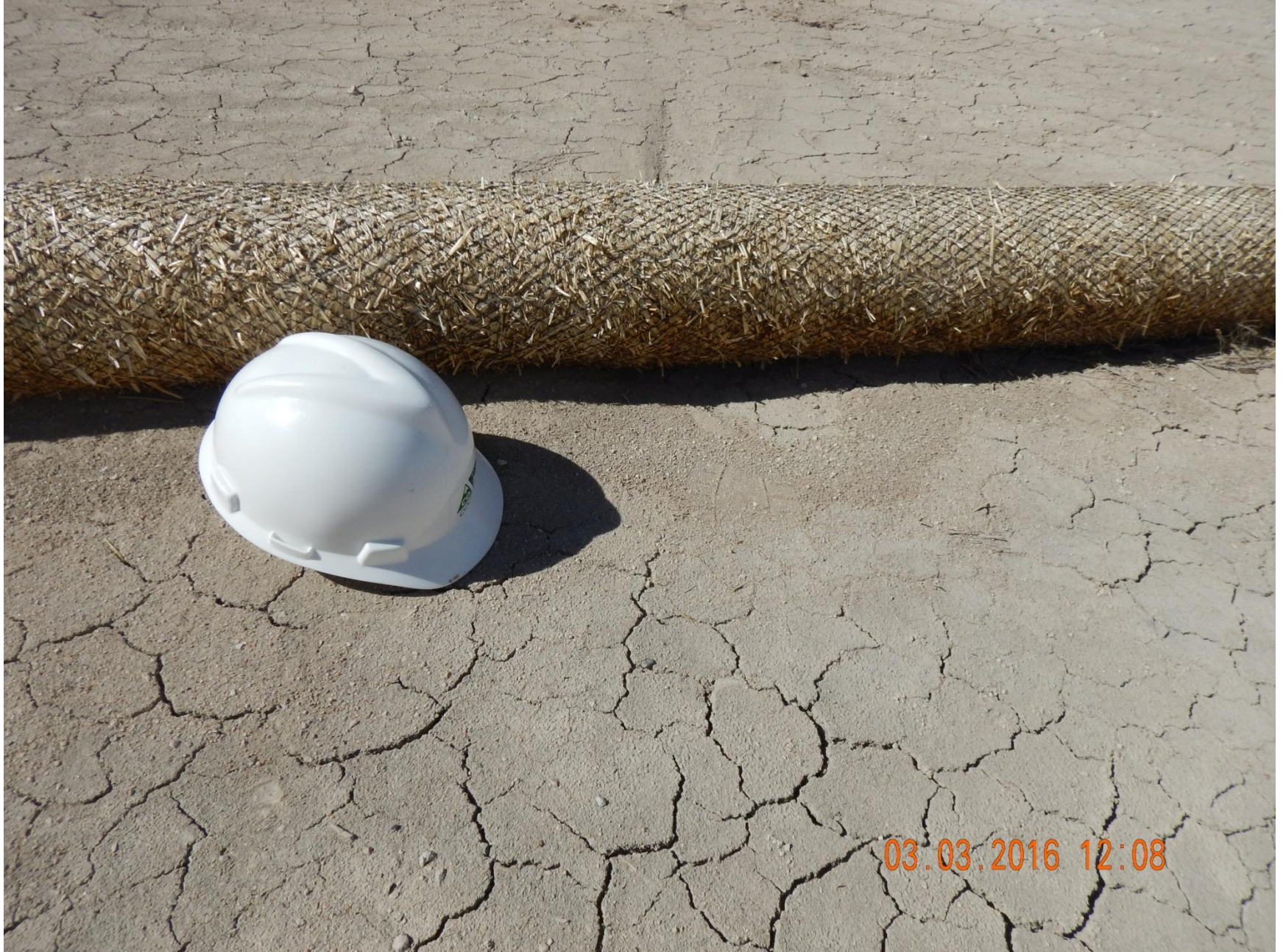
Figure 42: Photo taken from the southwestern end of location, facing west. Photo of straw wattles used as a stormwater and sediment control BMP not in proper functioning condition. Photo shows stormwater and sediment travel beneath the straw wattle.
