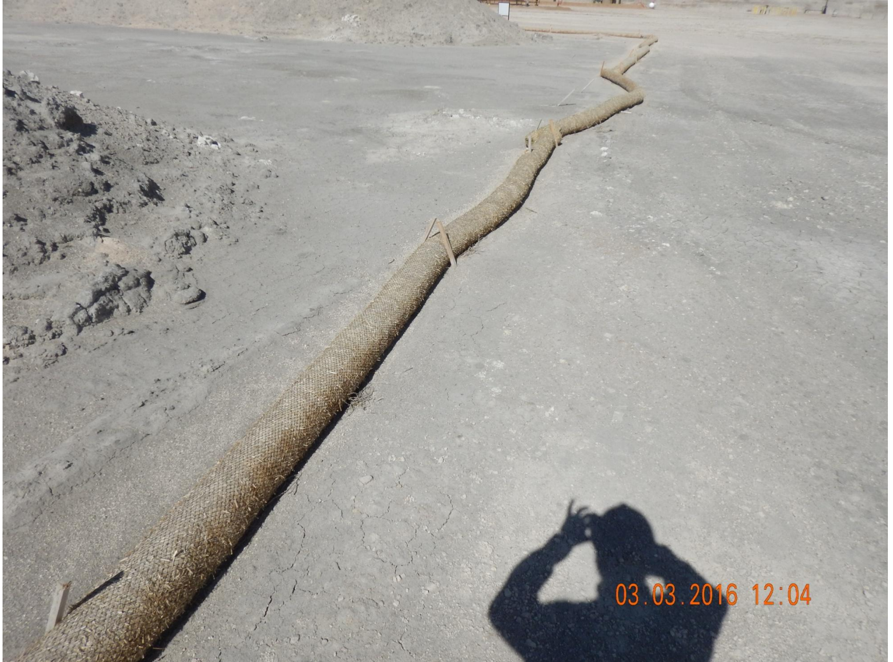
Figure 32: Photo taken from the southeast end of project area, facing north. Photo of straw wattle; wattle does not appear to be properly installed, and it appears water movement has dislodged the BMP. Straw wattle not in proper functioning condition.
