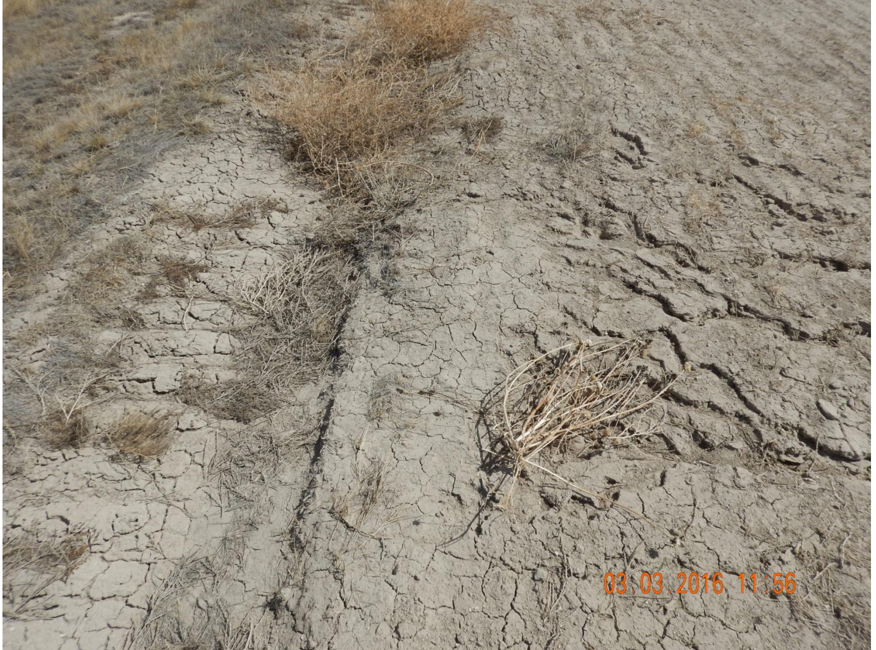
Figure 20: Photo taken from the north end of the location. Photo of rill erosion on slope. It appears rill erosion originates from the stormwater control ditch.
