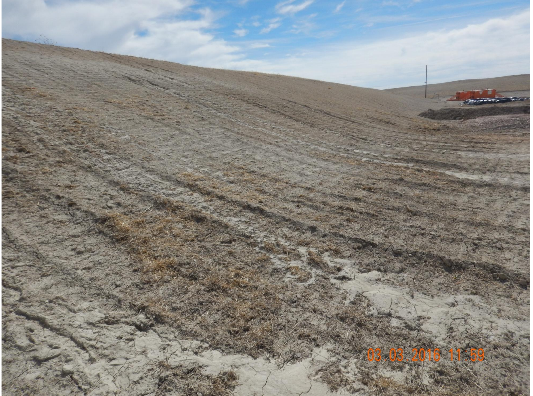
Figure 26: Photo taken from the northeast end of the project area, facing southeast towards the interim area. Photo shows the steep grade of the slope, rill erosion and sediment deposition.
