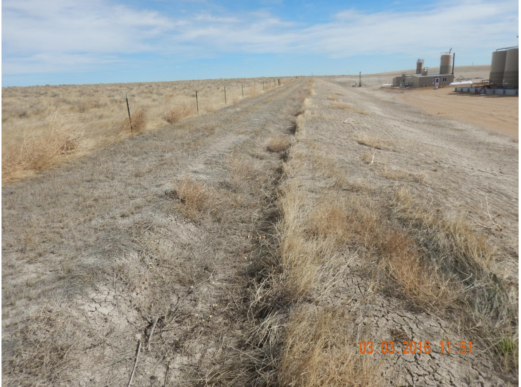
Figure 12: Photo taken from the northwest end of location, facing east. Photo shows stormwater and sediment control ditch used to divert stormwater on the northern perimeter of the location.
