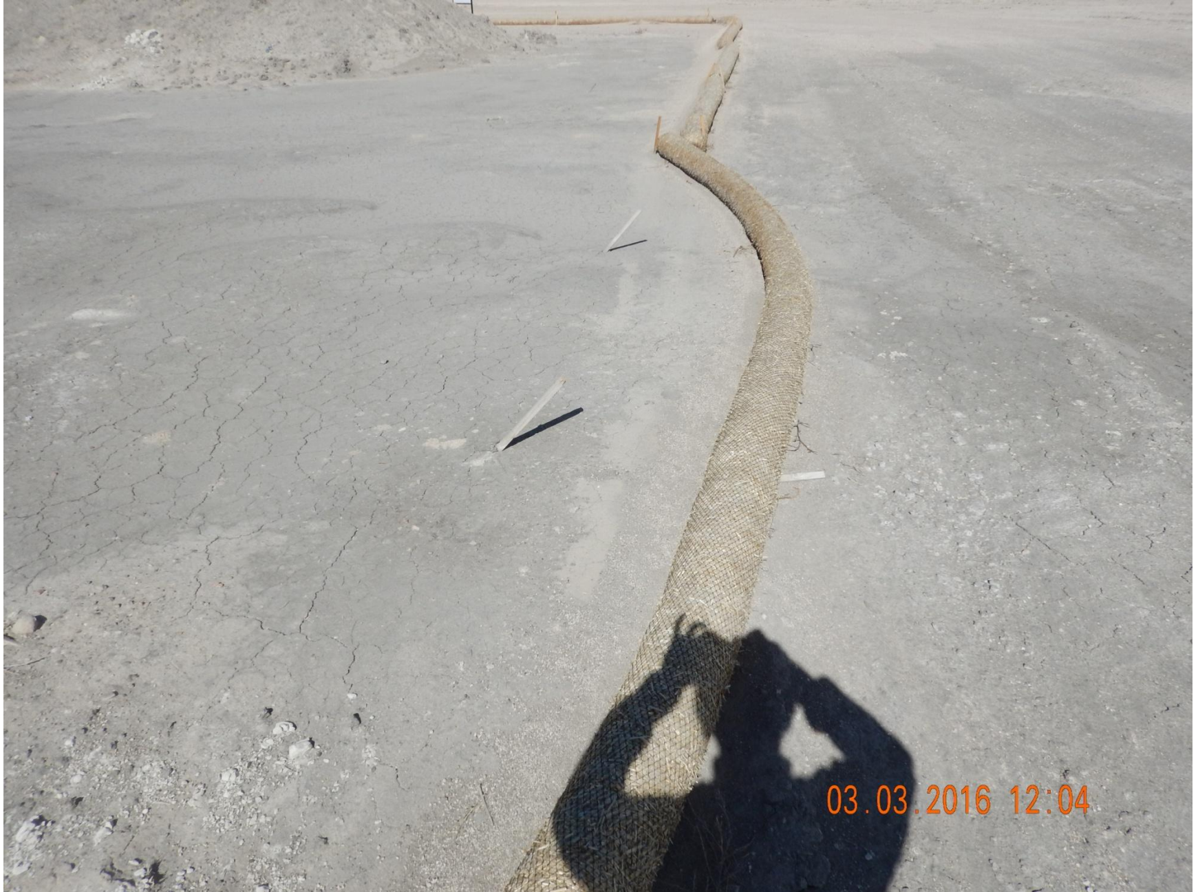
Figure 35: Photo taken from the southeast end of project area, facing north. Photo of straw wattle; wattle does not appear to be properly installed, and it appears water movement has dislodged the BMP. Straw wattle not in proper functioning condition.
