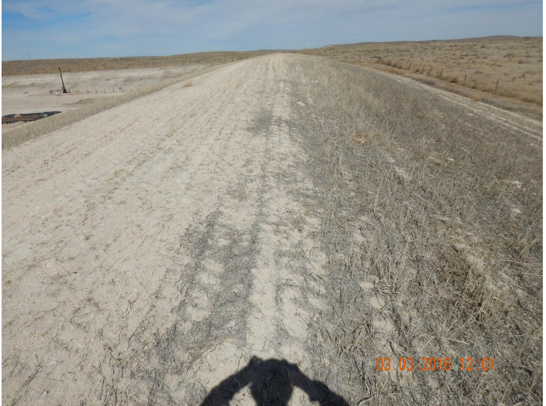
Figure 28: Photo taken from the east end of the project area, facing north. Photo shows portion of the interim lacking uniform vegetation.
