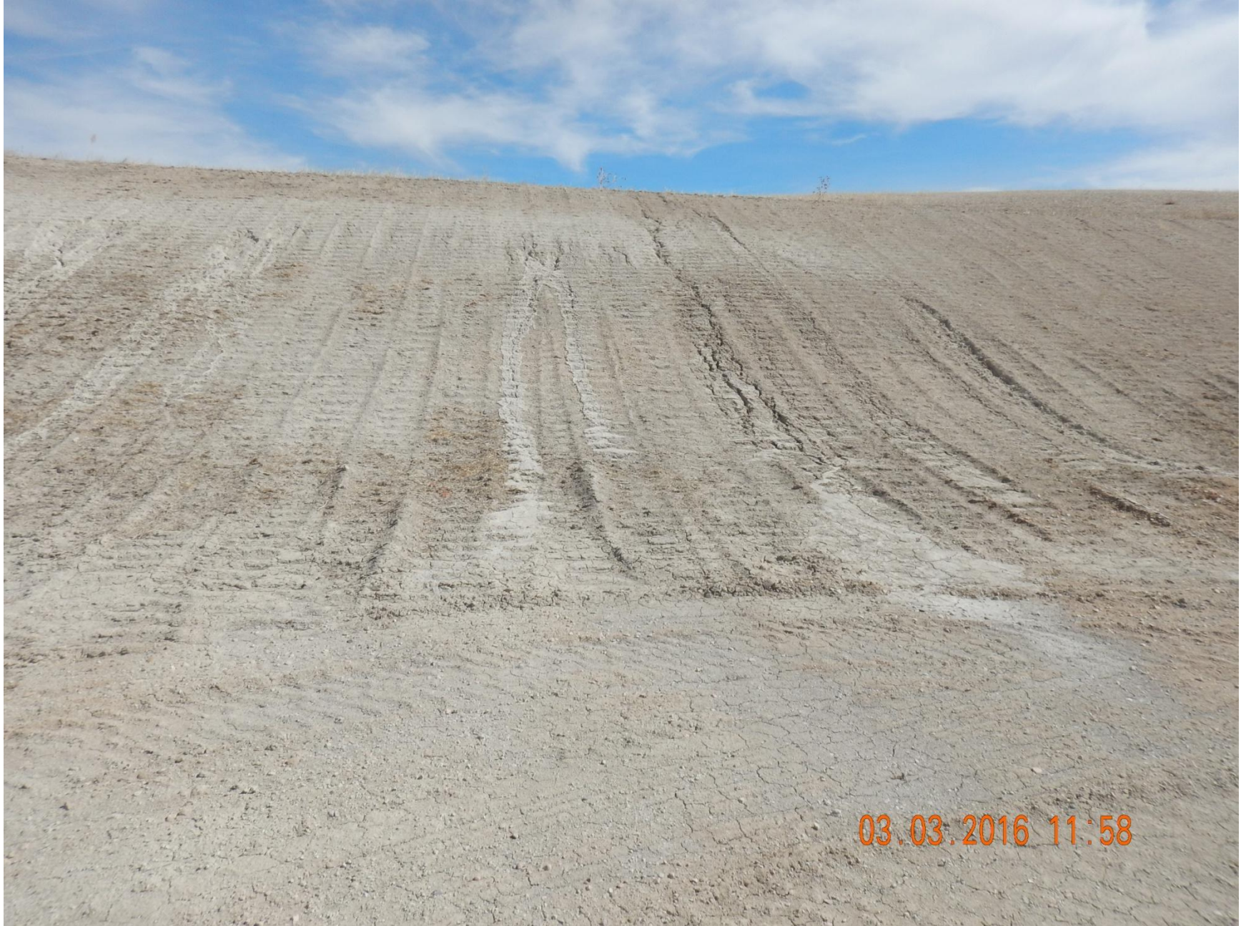
Figure 25: Photo taken from the northeast end of the project area, facing east towards the interim area. Photo shows the steep grade of the slope, rill erosion and sediment deposition.
