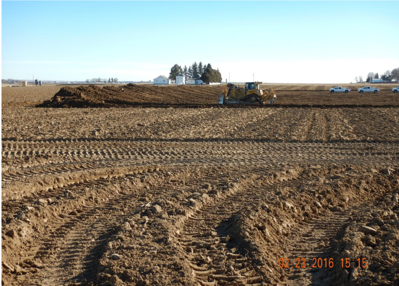
Photo 12. Photo taken from the northern location, facing Northeast. Topsoil salvage in process.
