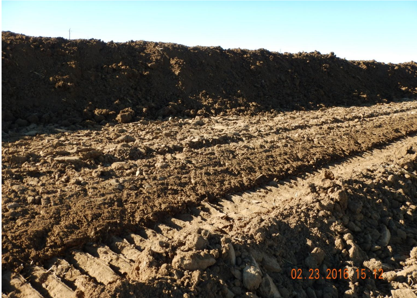
Photo 10. Photo taken from the eastern location, facing West. Topsoil stockpile in center of photo. Need to stabilize topsoil stockpile upon completion of topsoil salvage process.
