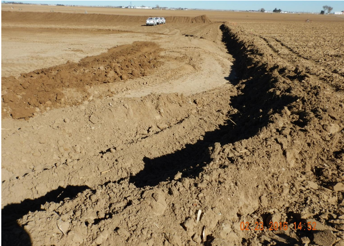
Photo 2. Photo taken from southwestern location, facing East. Stormwater and sediment control BMPs installed in center of photo.
