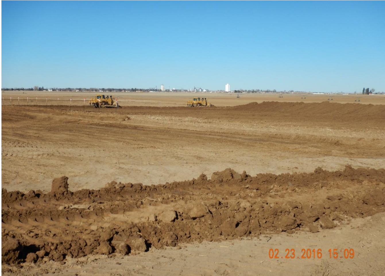
Photo 11. Photo taken from the southern location, facing Northeast. Topsoil salvage in process.
