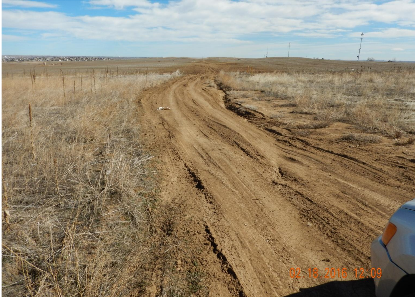
Photo 8. Photo taken from access road east of location, facing East. Appears to be noticeable erosion occurring along both sides of the access road ditch. Sediment traveling east, down slope towards the agricultural field.
