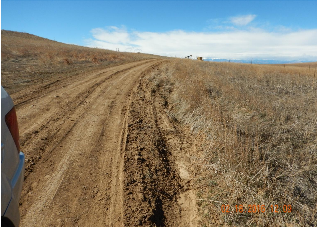
Photo 7. Photo taken from access road east of location, facing West. Appears to be noticeable erosion occurring along both sides of the access road ditch (see following photo).
