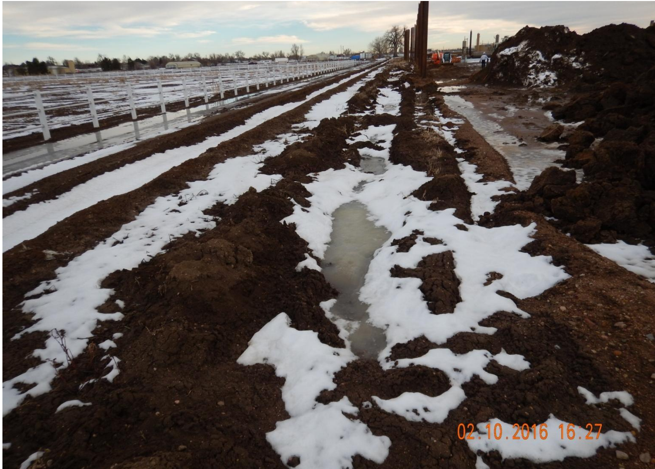
Photo 6. Photo taken from northeast location, facing South. Stormwater BMP installed along perimeter of location. Need to stabilize topsoil stockpile and prevent soil leaving location. Operator said topsoil stockpile is in process of being moved from the western area to create space for operations.
