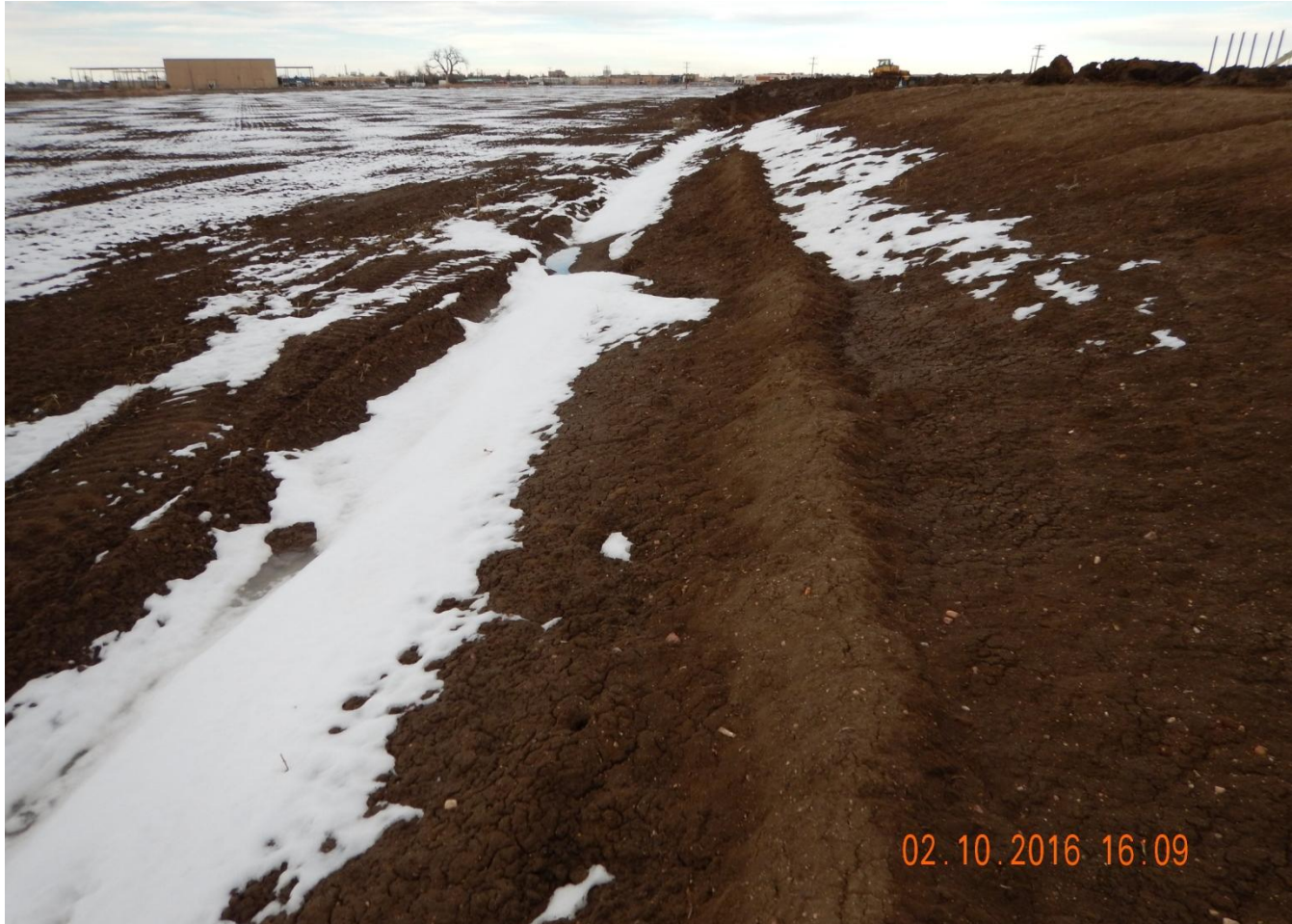
Photo 3. Photo taken from southwest location, facing North. Topsoil stockpile in center of photo and stormwater and sediment BMP along west-facing toe.
