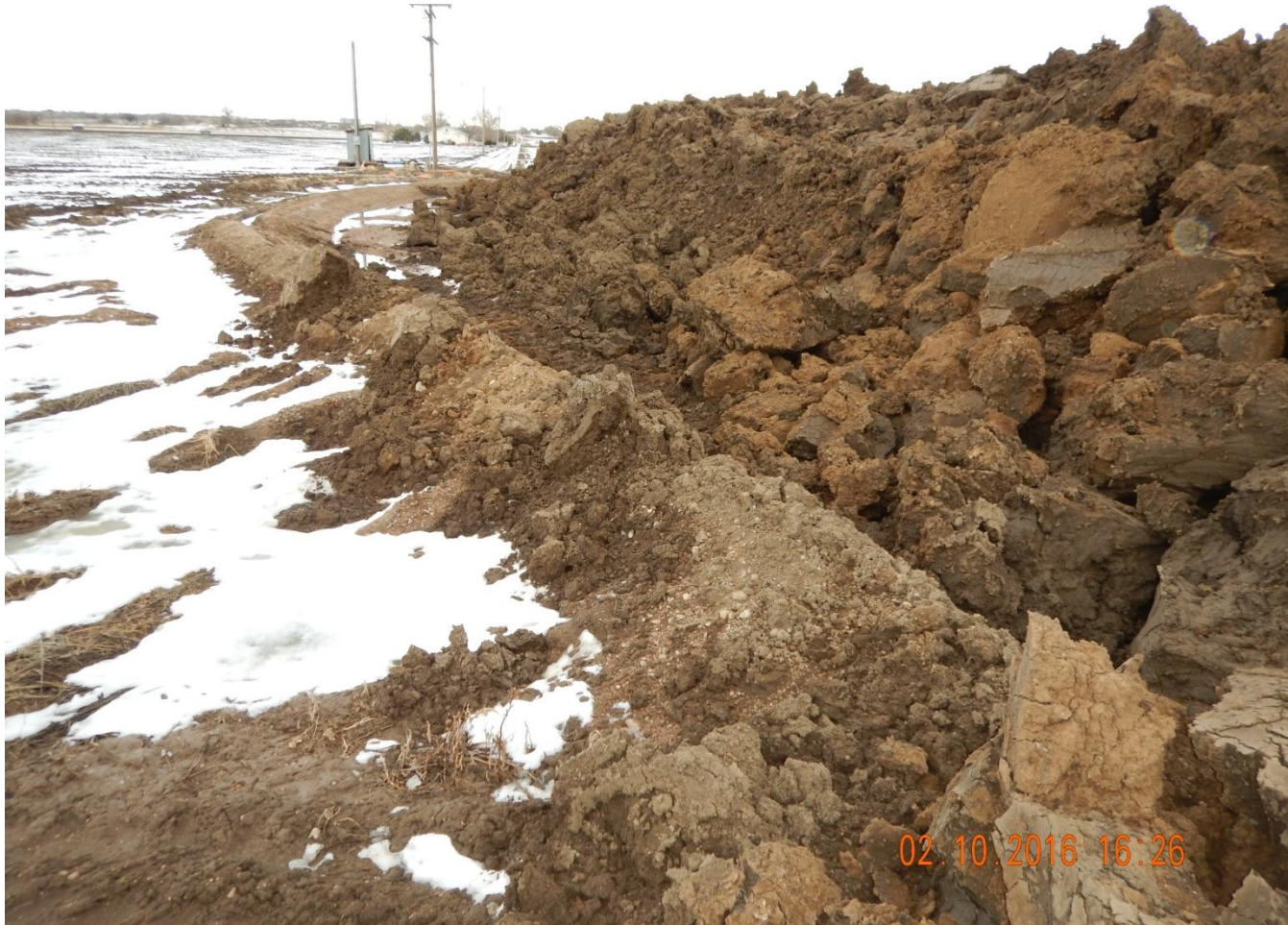
Photo 5. Photo taken from northwest location, facing East. Stormwater BMP installed along perimeter of location. Need to stabilize topsoil stockpile and prevent soil leaving location. Operator said topsoil stockpile is in process of being moved from the western area to create space for operations.
