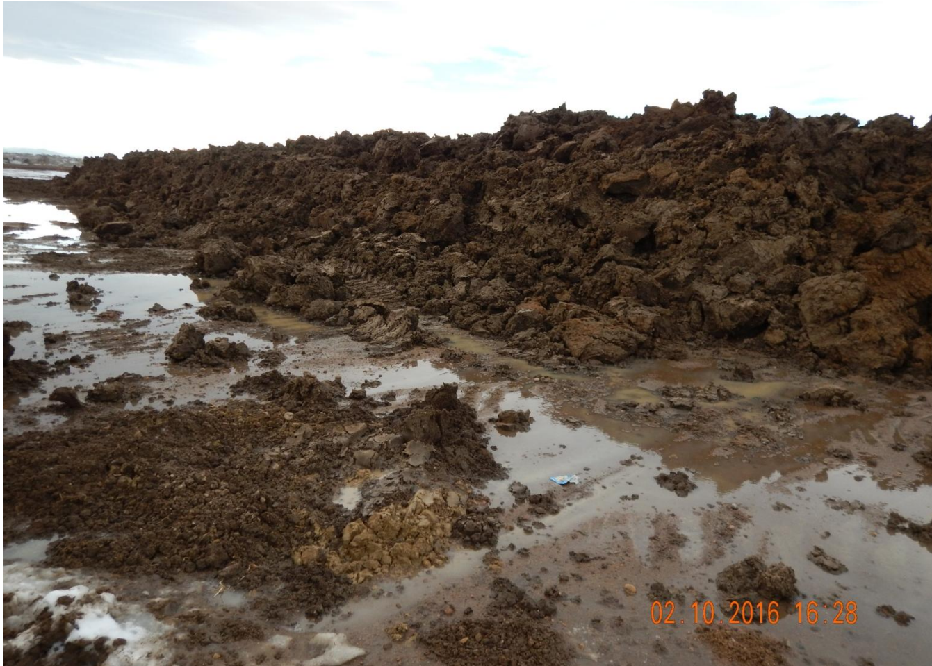
Photo 7. Photo taken from northeast location, facing West. Need to stabilize topsoil stockpile and prevent soil leaving location. Operator said topsoil stockpile is in process of being moved from the western area to create space for operations.
