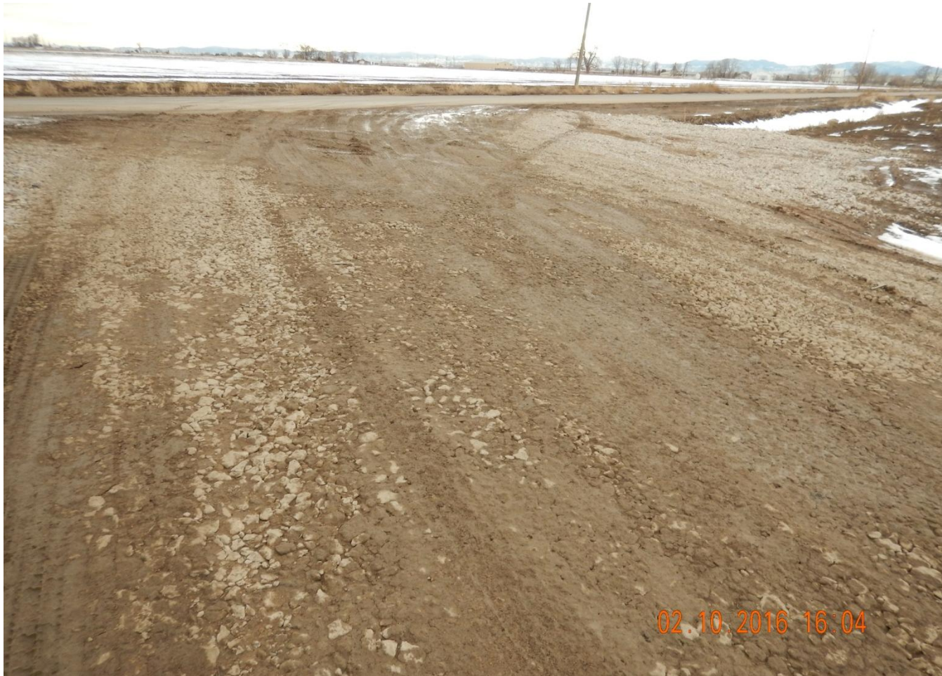
Photo 1. Photo taken from entrance of location, facing South. Tracking device installed to prevent sediment leaving location. Operator said gravel will be fluffed up to maintain proper functional use.
