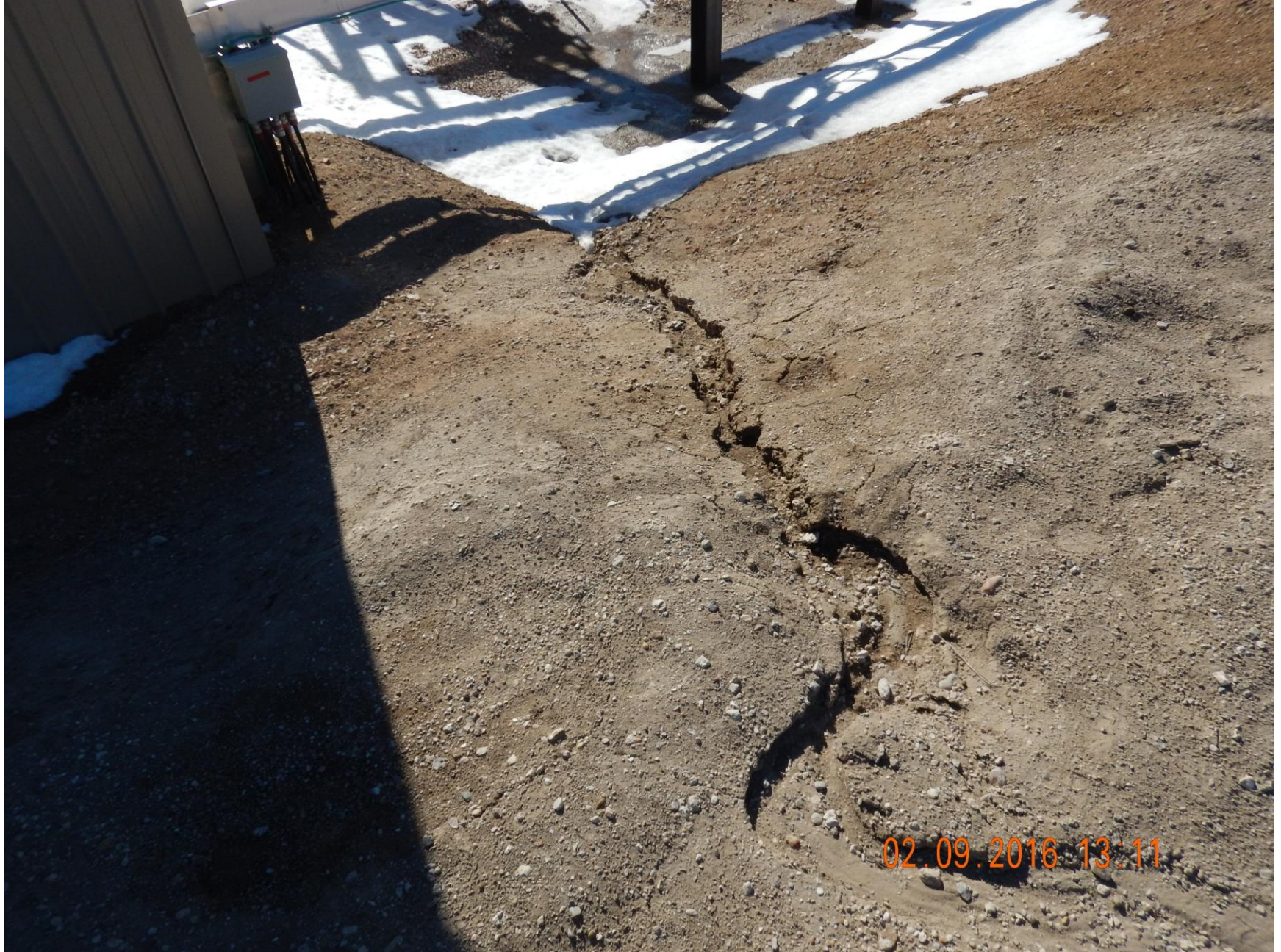
Figure 9: Photo taken from the north end of the location. Photo of erosion forming on slope of the perimeter. This is evidence that slope is not stabilized.
