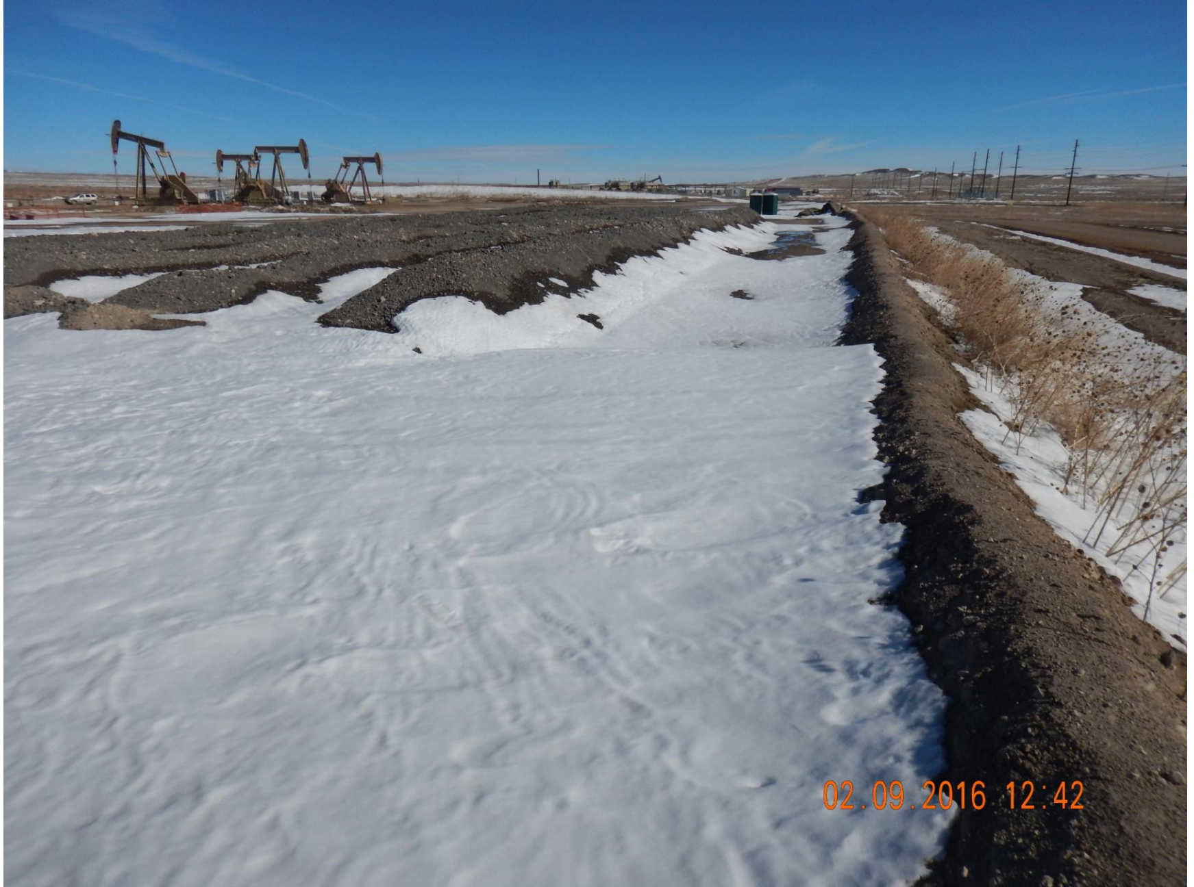
Figure 13: Photo taken southwest end of location, facing east. Photo of drill cuttings stored on location, and stormwater berm.
