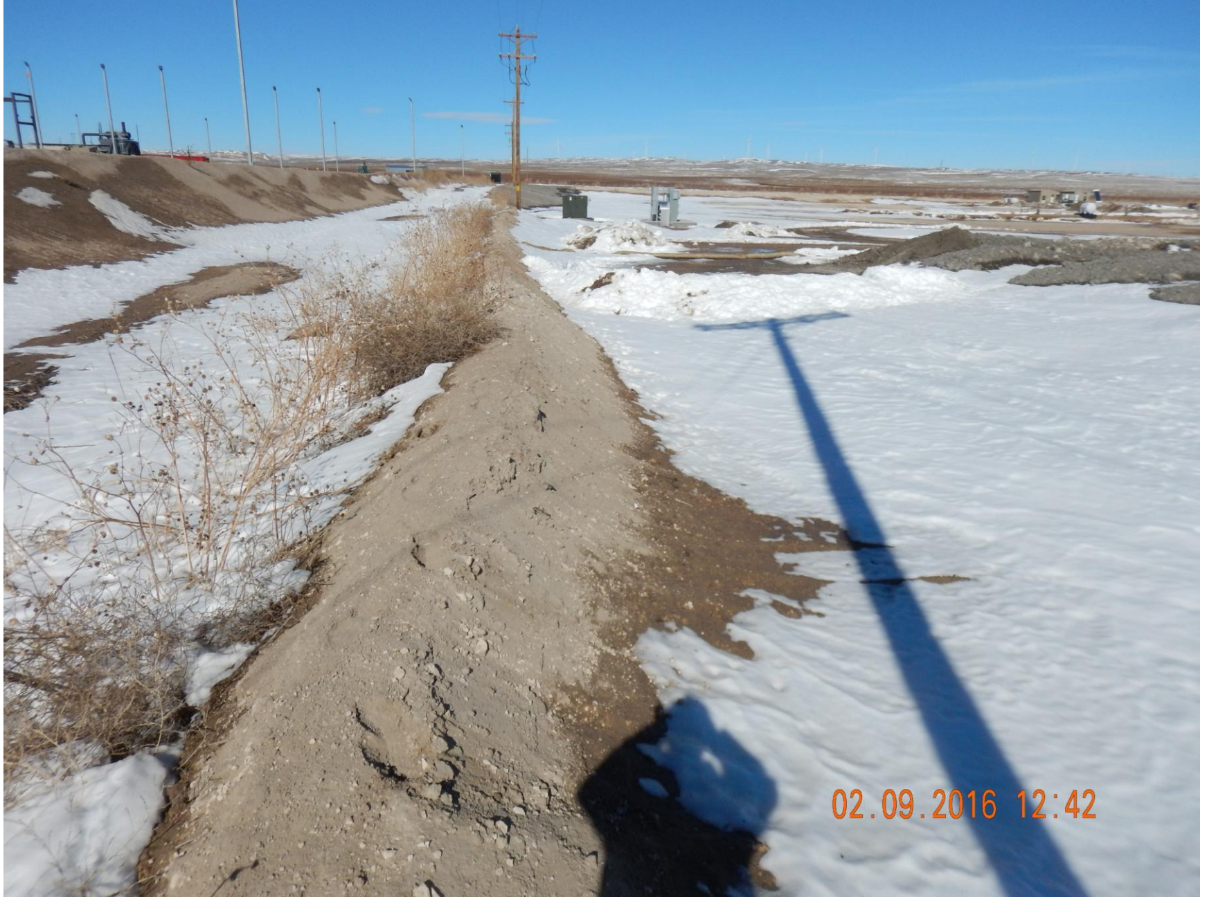
Figure 12: Photo taken southwest end of location, facing north. Photo of stormwater control berm.
