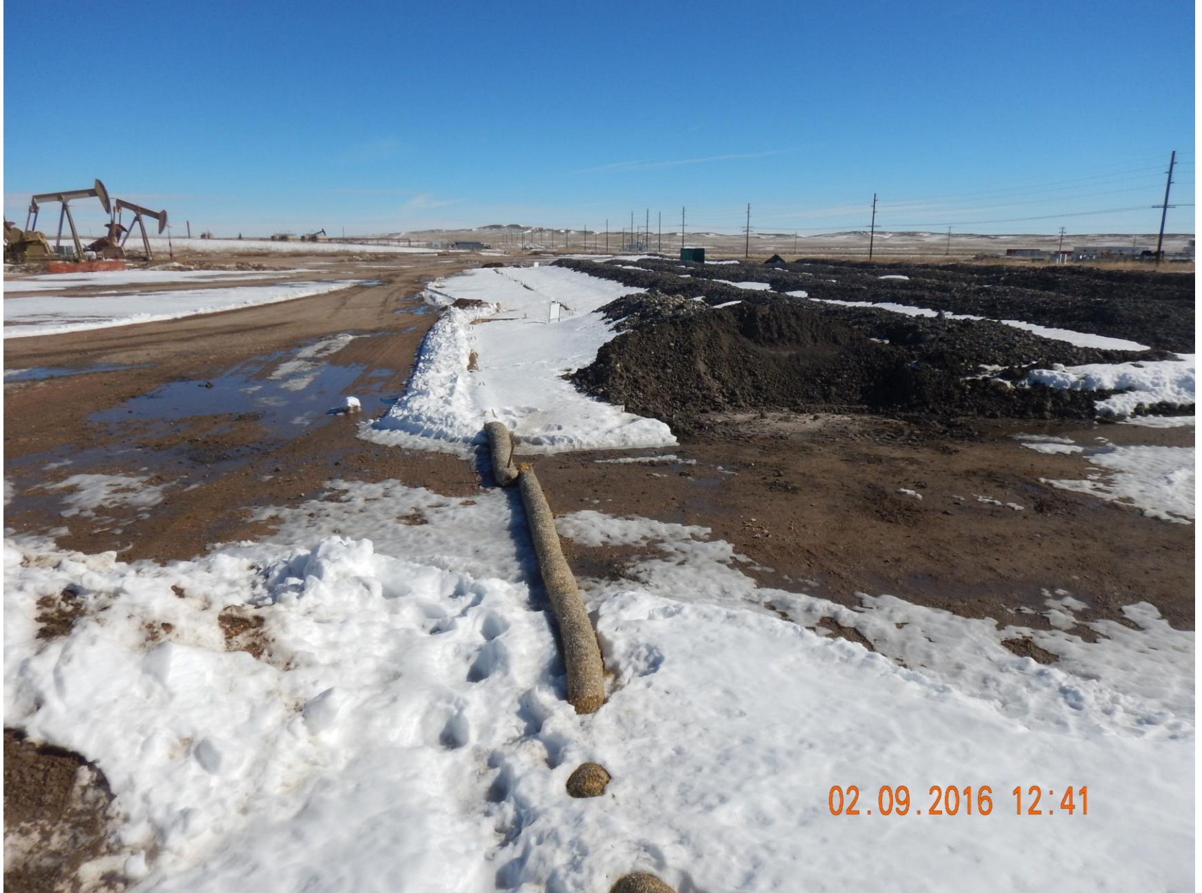
Figure 11: Photo taken southwest end of location, facing east. Photo of drill cuttings stored on location, and stormwater waddles.
