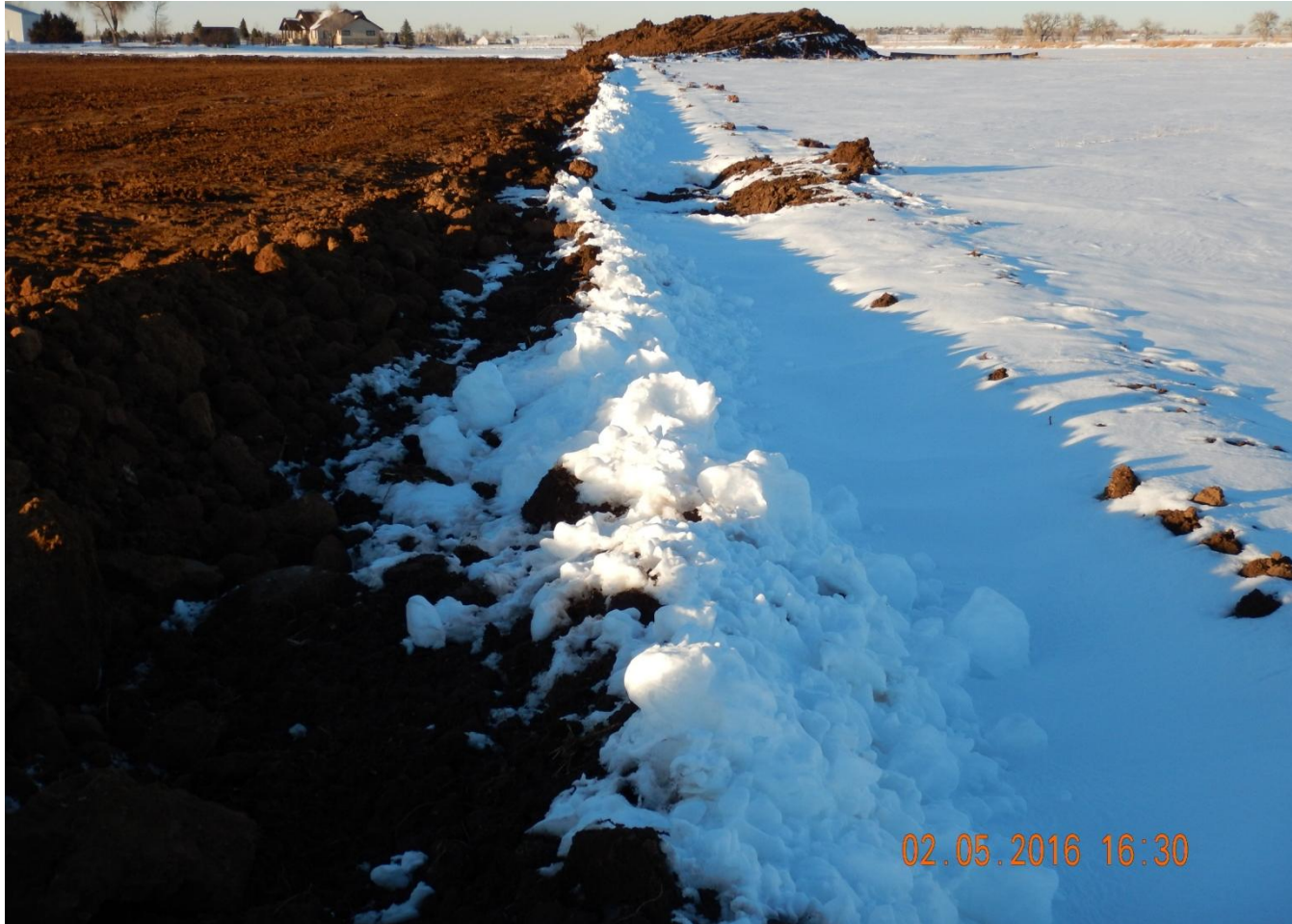
Photo 2. Photo taken from southeast location, facing North. Stormwater and sediment control BMPs installed along perimeter of location.
