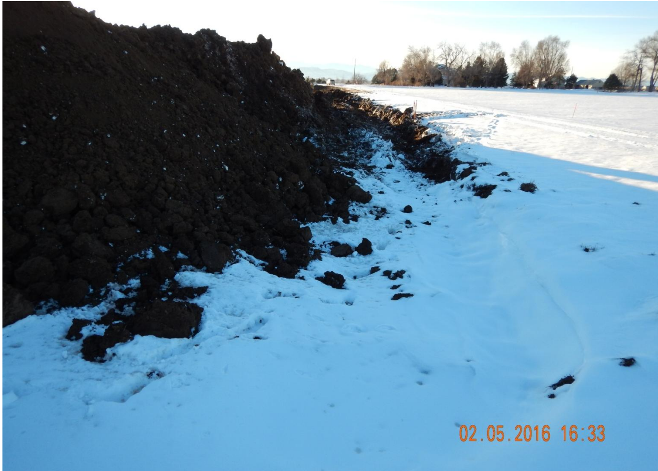
Photo 4. Photo taken from northeast location, facing West. Stormwater and sediment control BMPs installed along perimeter of location. Topsoil stockpile needs to be stabilized upon completion of salvage operations.
