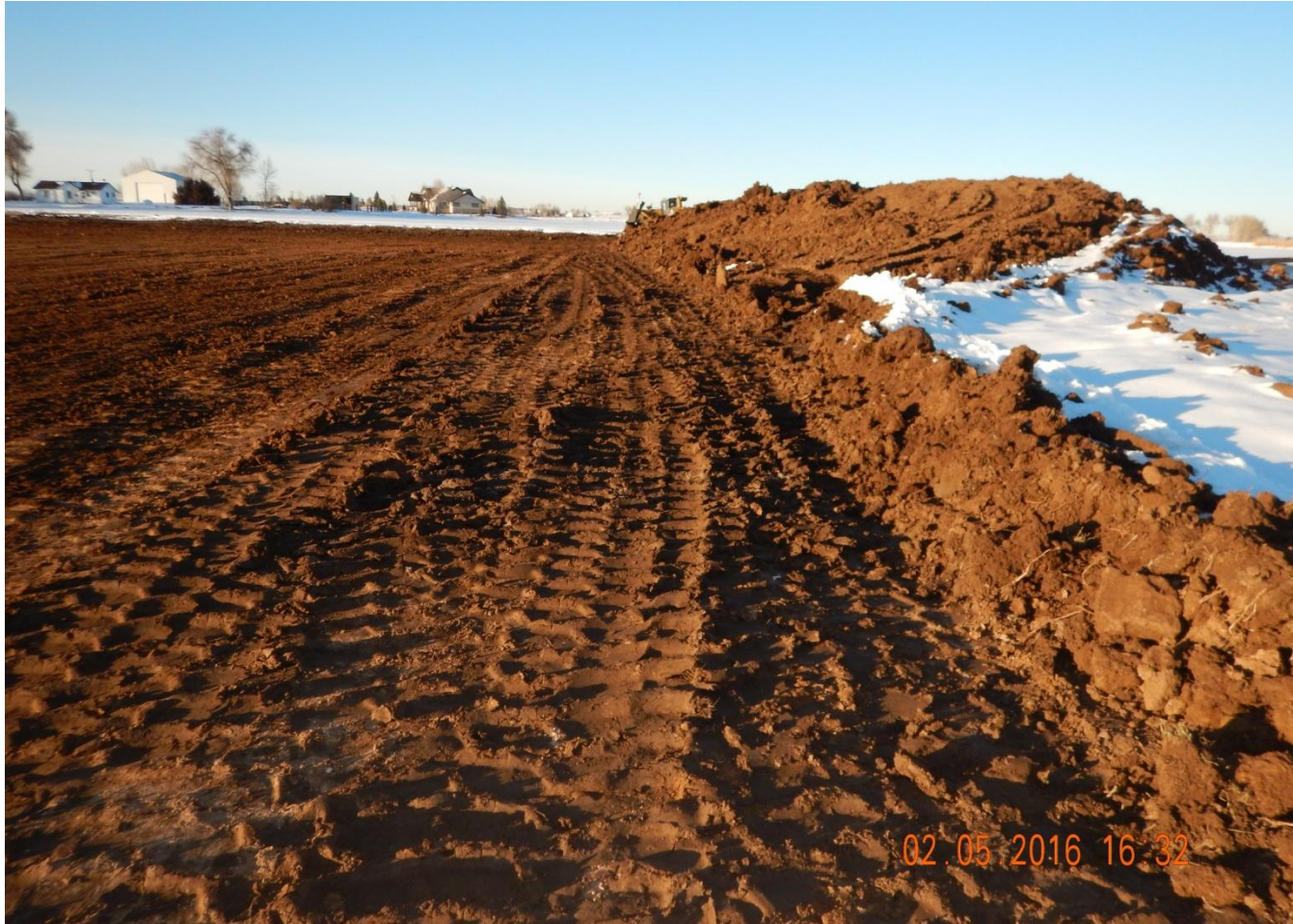
Photo 5. Photo taken from eastern location, facing North. Topsoil stockpile located in center of photo. Topsoil stockpile needs to be stabilized upon completion of salvage operations.
