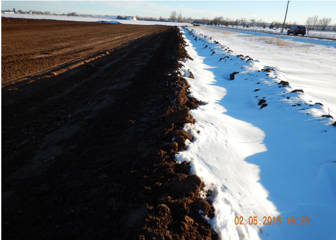
Photo 1. Photo taken from northwest location, facing South. Stormwater and sediment control BMPs installed along perimeter of location.
