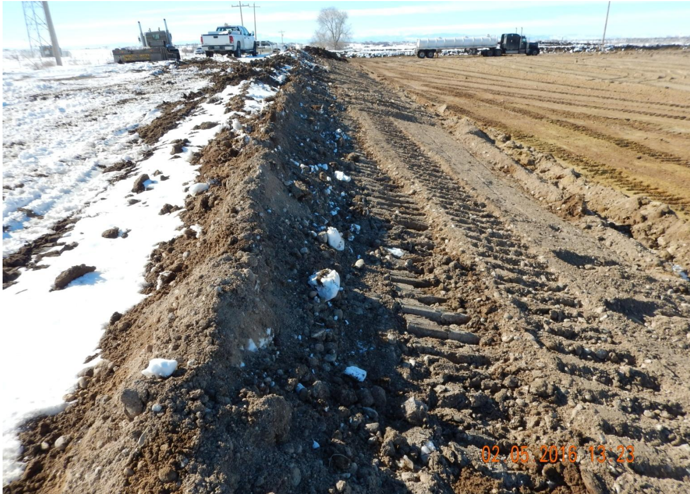
Photo 8. Photo taken from southern location, facing West. Stormwater and sediment control BMPs installed along perimeter of location. CDOT recommends that berms be properly compacted with no breaks in the berm. Operator said that perimeter berms will be compacted once favorable conditions are permitted.
