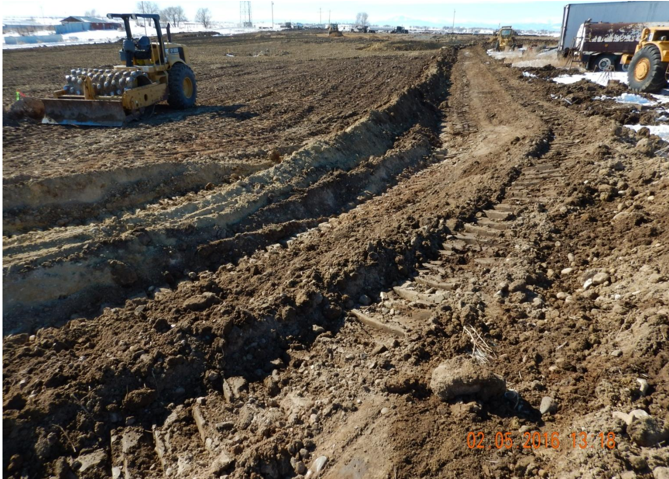
Photo 5. Photo taken from eastern location, facing West. Stormwater and sediment control BMPs installed along perimeter of location. CDOT recommends that berms be properly compacted with no breaks in the berm. Operator said that perimeter berms will be compacted once favorable conditions are permitted.
