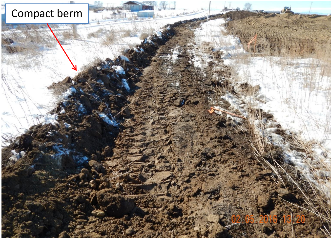
Photo 6. Photo taken from southeast location, facing West. Stormwater and sediment control BMPs installed along perimeter of location. CDOT recommends that berms be properly compacted with no breaks in the berm. Operator said that perimeter berms will be compacted once favorable conditions are permitted.
