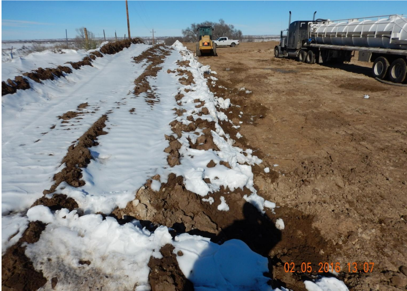
Photo 2. Photo taken from southwest location, facing North. Stormwater and sediment control BMPs installed along perimeter of location.
