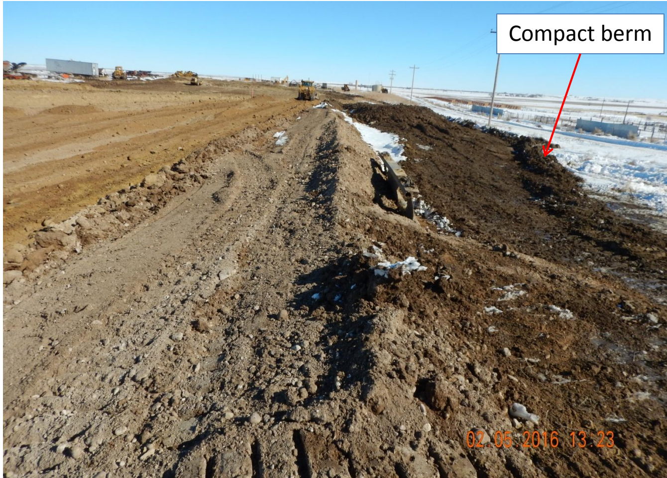
Photo 7. Photo taken from southern location, facing East. Stormwater and sediment control BMPs installed along perimeter of location. CDOT recommends that berms be properly compacted with no breaks in the berm. Operator said that perimeter berms will be compacted once favorable conditions are permitted.
