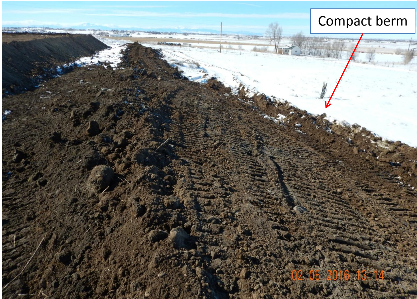
Photo 3. Photo taken from northern location, facing West. Stormwater and sediment control BMPs installed along perimeter of location. CDOT recommends that berms be properly compacted with no breaks in the berm. Operator said that perimeter berms will be compacted once favorable conditions are permitted.
