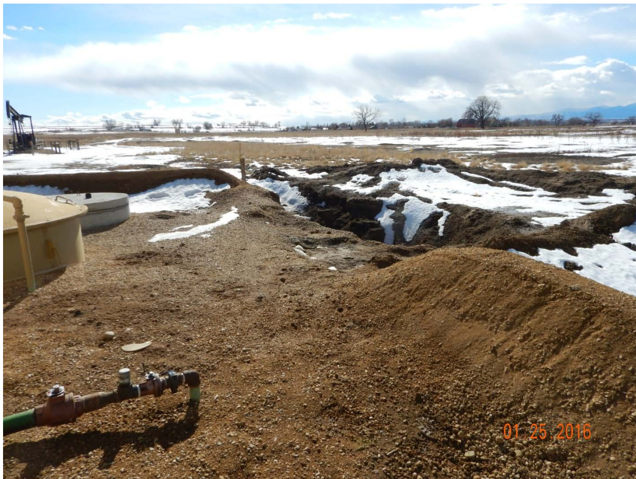
Figure 4 - Excavation and compromised containment at SW corner of tank battery
