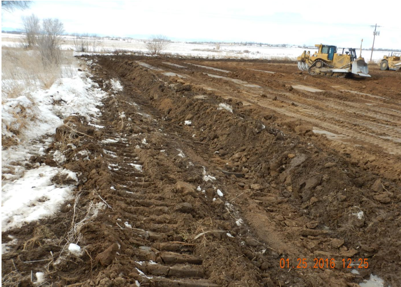
Photo 6. Photo taken from southern location, facing West. Stormwater and sediment control BMPs installed before construction.
