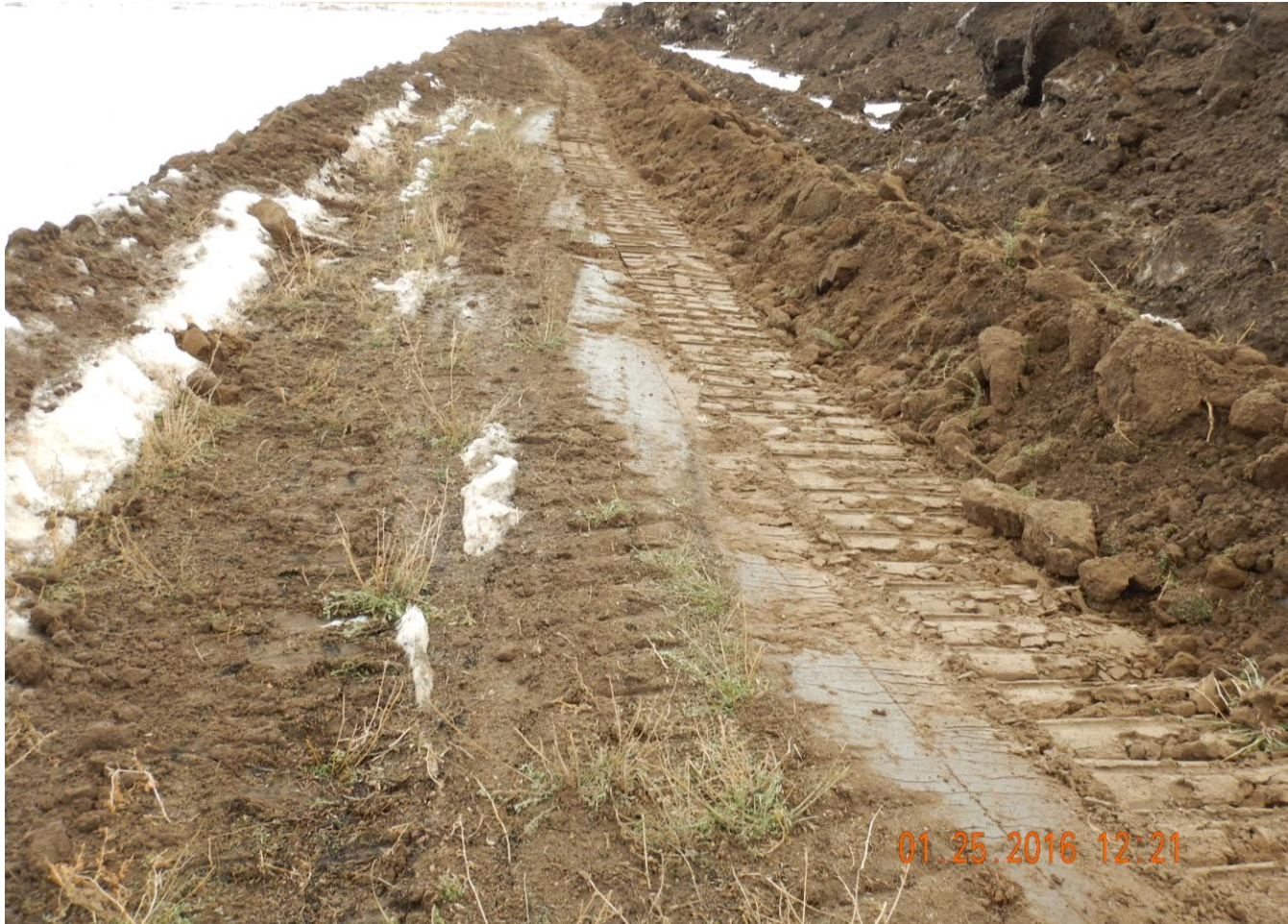
Photo 5. Photo taken from eastern location, facing South. Stormwater and sediment control BMPs installed before construction.
