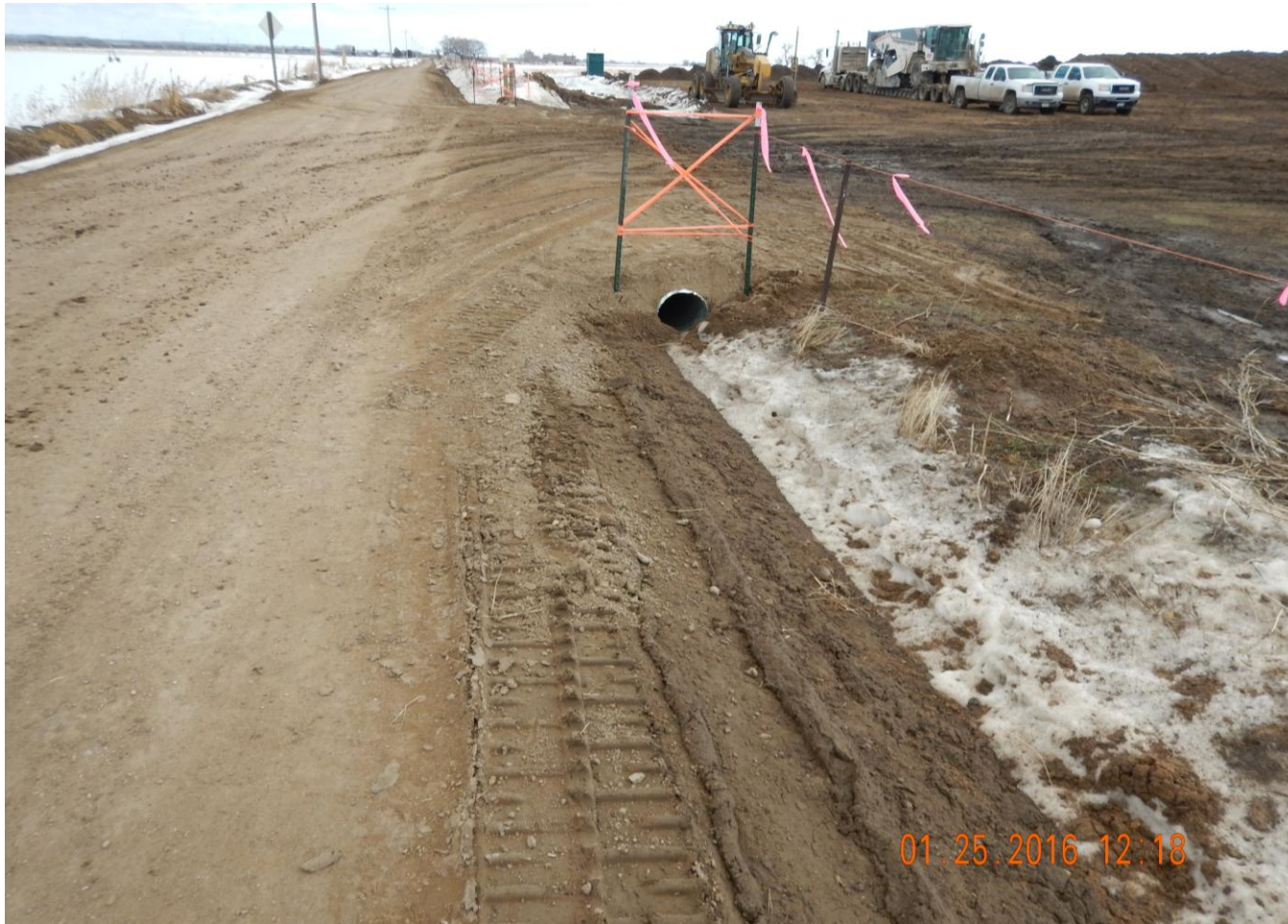
Photo 1. Photo taken from entrance, facing East. Stormwater and sediment control BMPs installed before construction.
