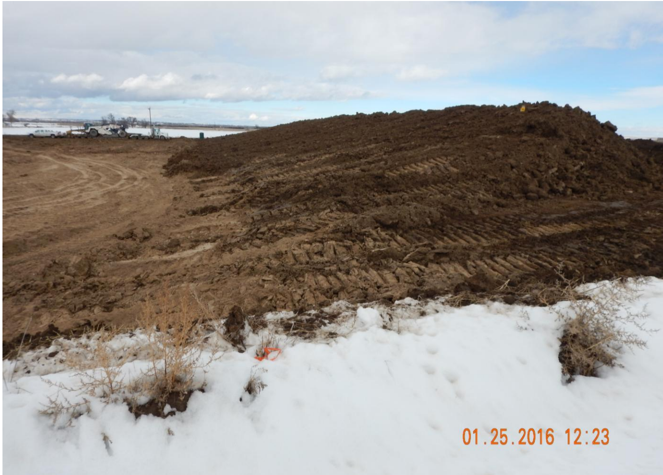
Photo 8. Photo taken from southern location, facing North. Topsoil salvage in process. Need to stabilize topsoil stockpile upon completion of topsoil separation.
