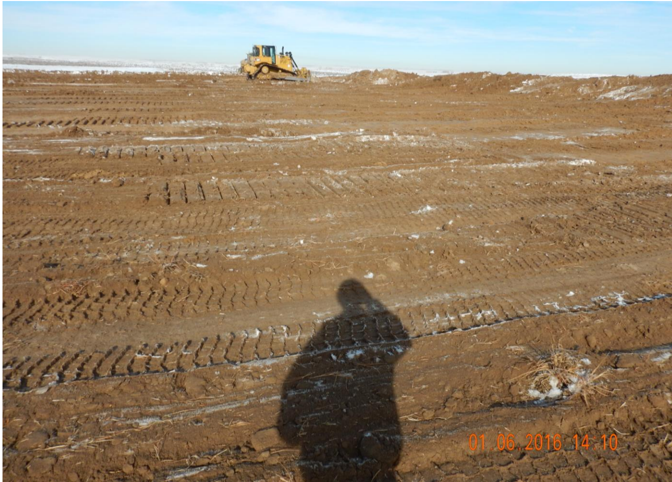
Photo 2. Photo taken from the southern location, facing North. Topsoil salvage in process.
