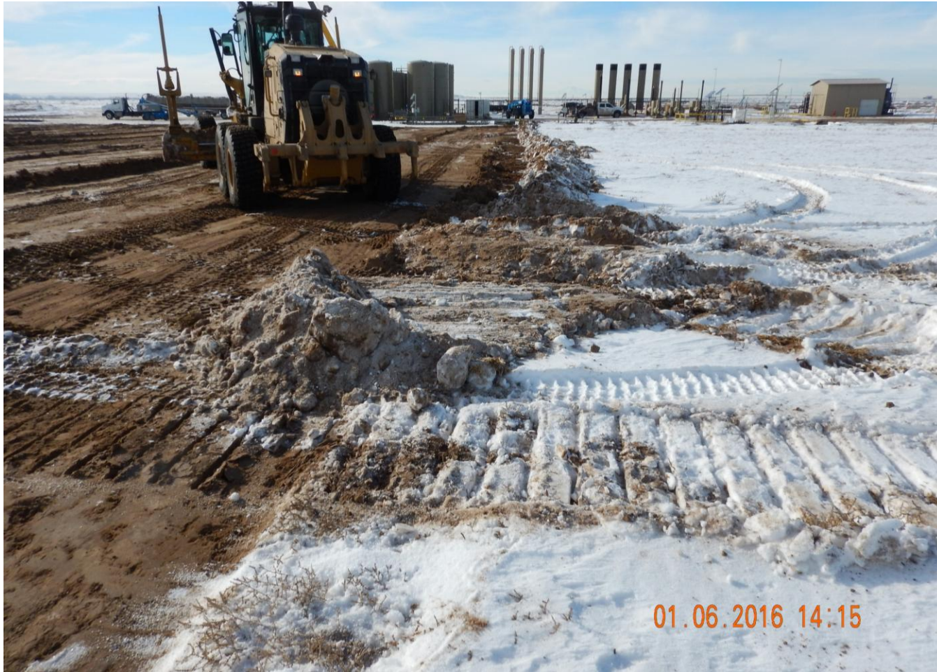
Photo 3. Photo taken from the northeast location, facing West. Stormwater BMPs need to be installed before construction starts.
