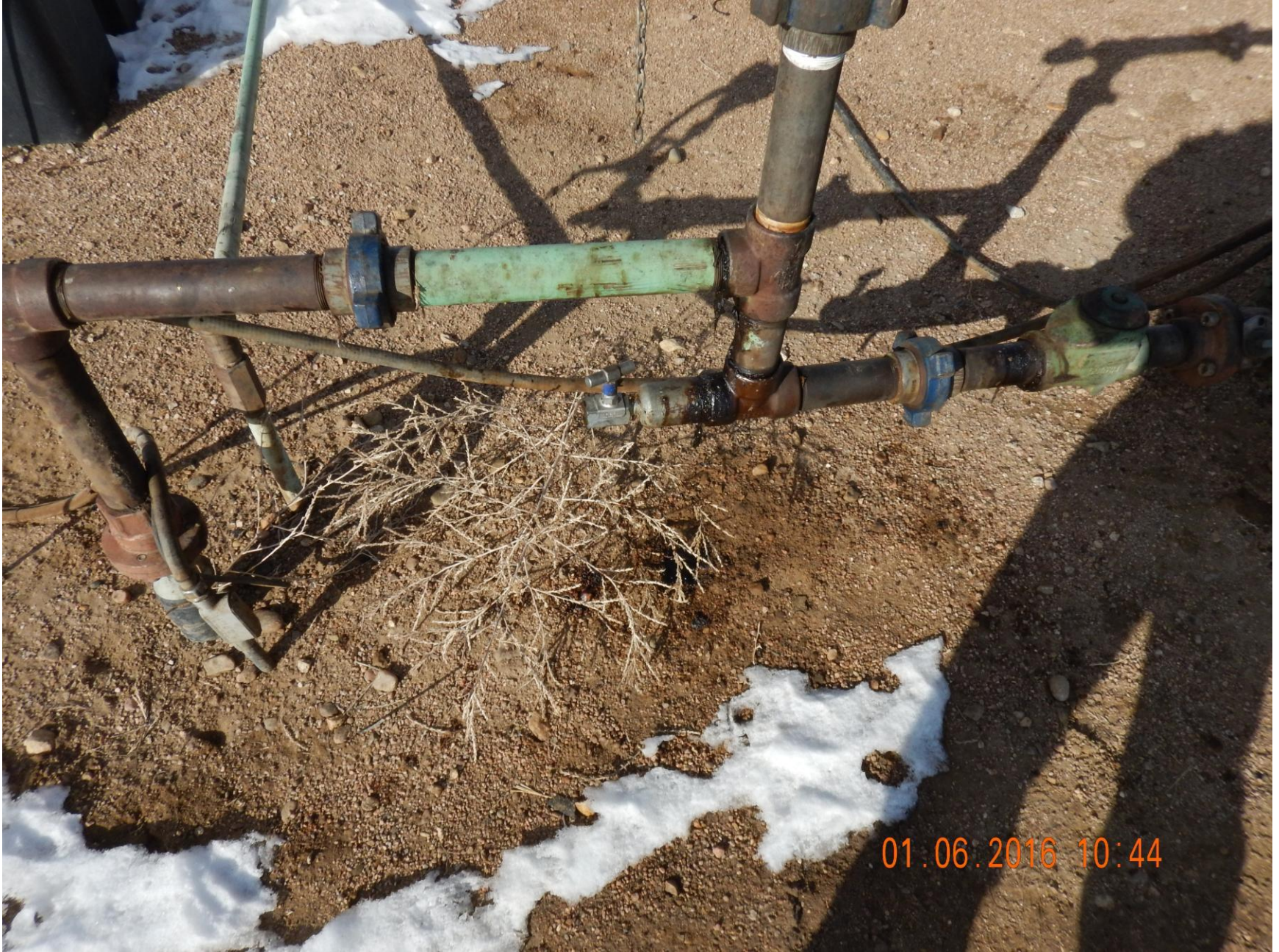
Figure 2: Photo taken at well. Photo shows stained soil and small leak.
