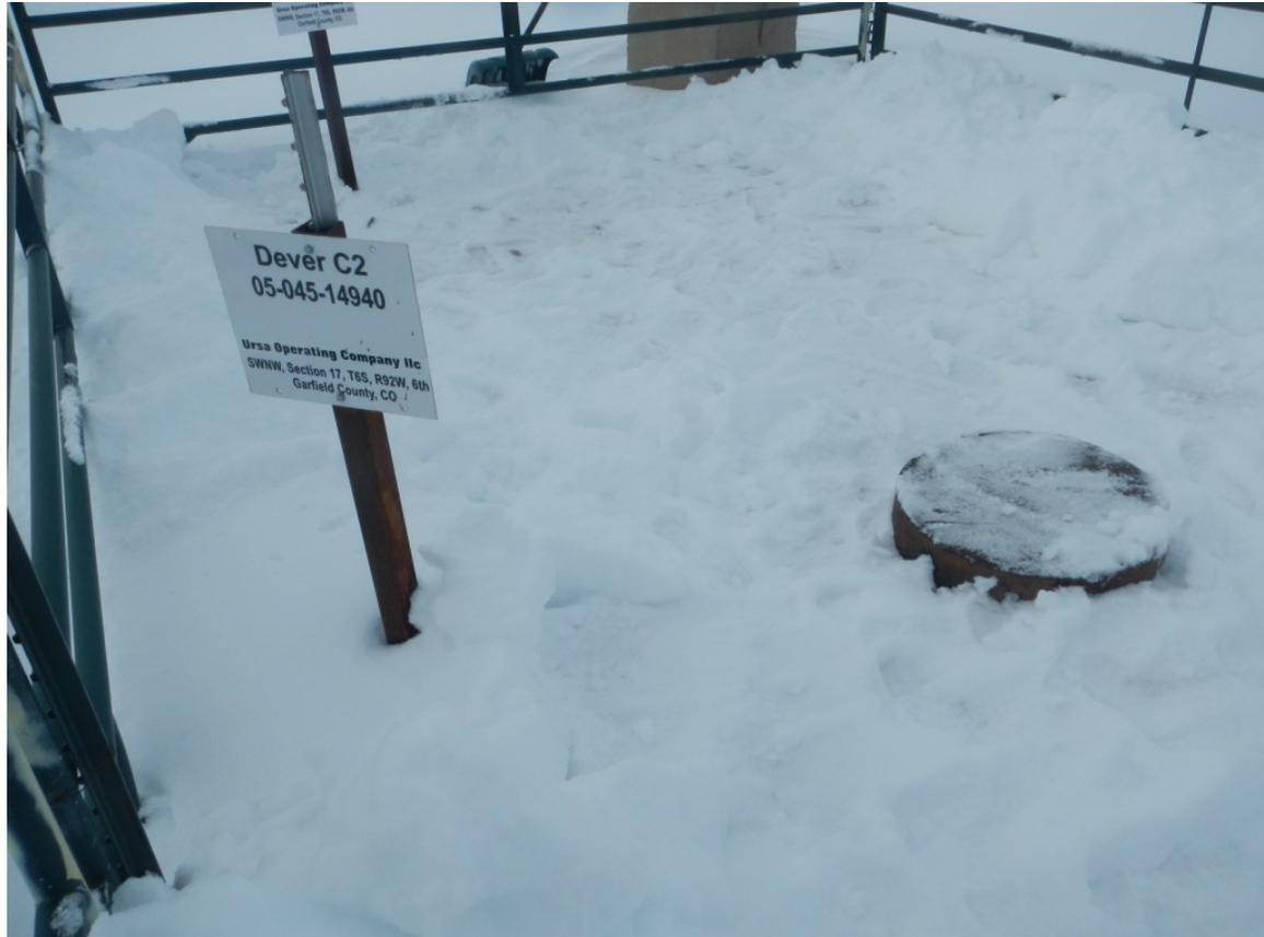
Photo#2: AL Well 045- 14940 has Identifying Sign and Conductor Set .
