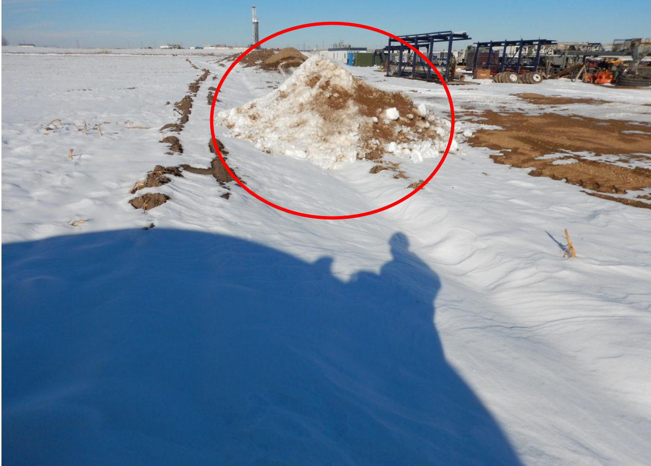
Photo 4. Photo taken from southwest location, facing North. Stormwater BMP installed in center of photo. DO NOT scrape sediment into stormwater ditches. Stormwater ditches need to be maintained.
