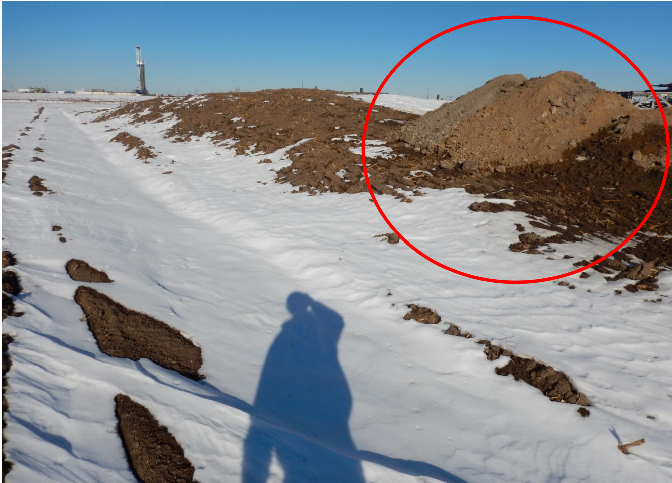
Photo 5. Photo taken from western location, facing North. Stormwater BMP installed in center of photo. DO NOT pile other soil material onto topsoil stockpile. Need to remove soil pile from topsoil stockpile.
