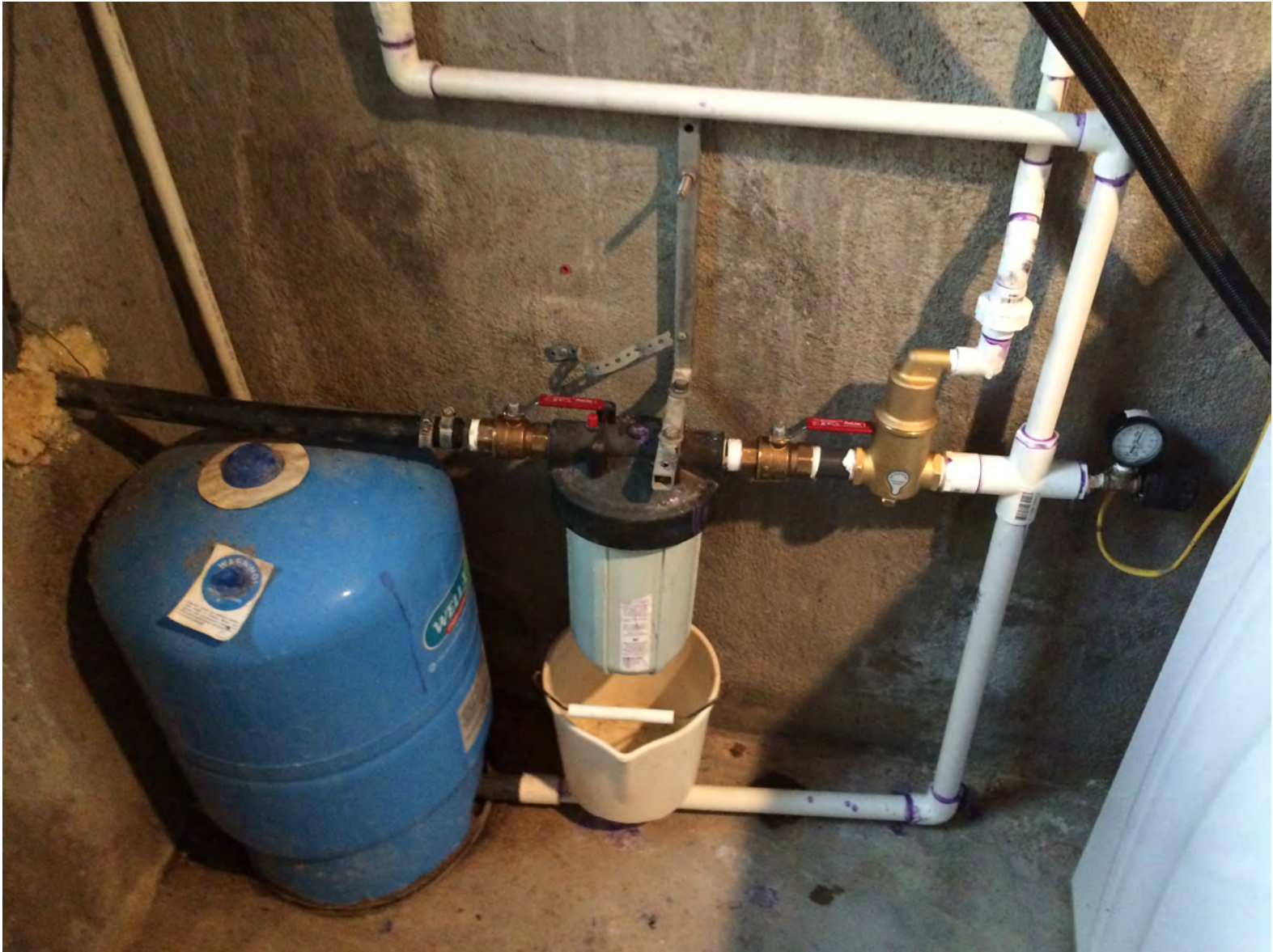
Inline Separator / Air Eliminator -- Post Installation
