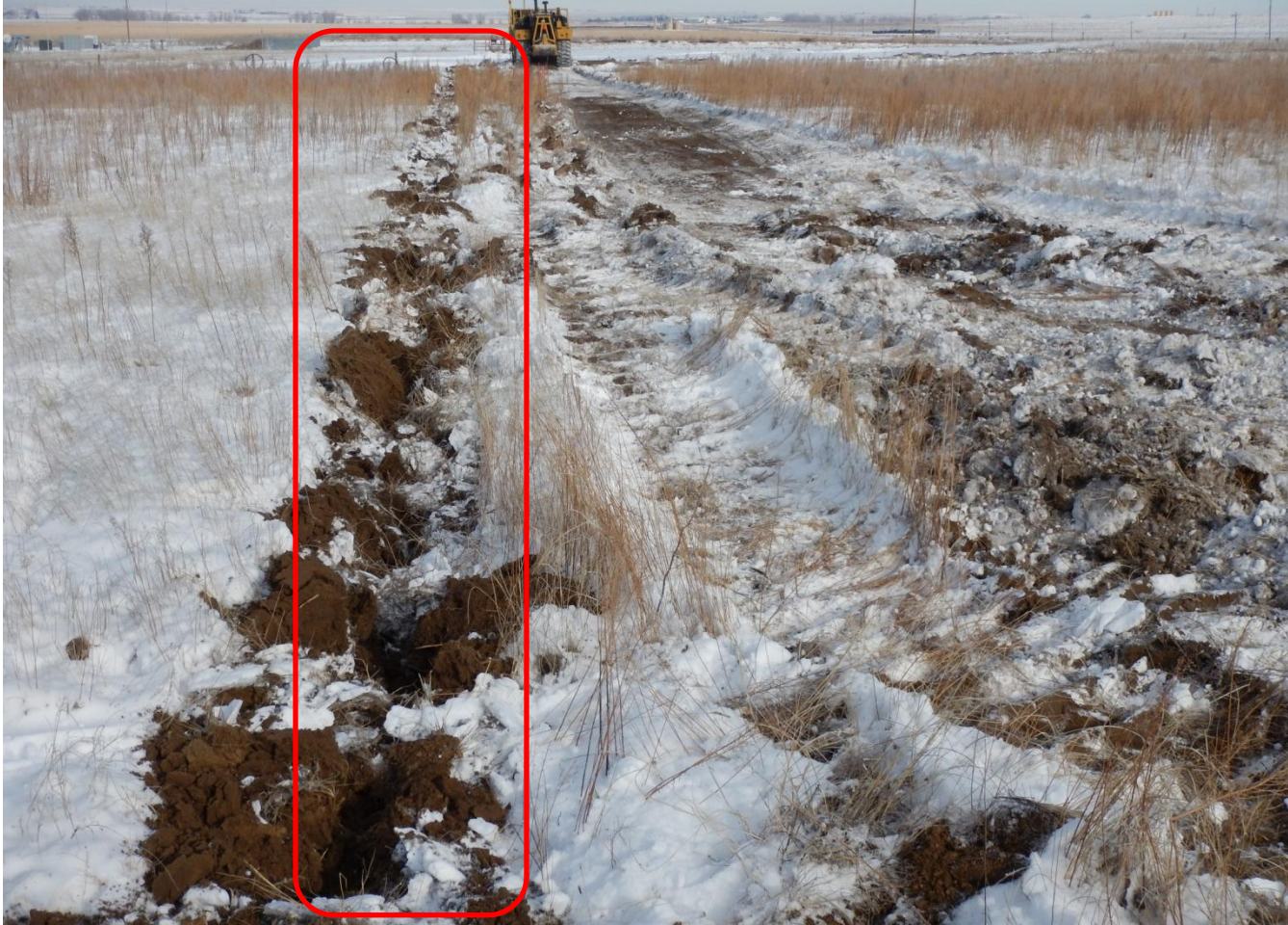
Photo 2. Photo taken from southwestern corner, facing North. Stormwater BMP installed prior to construction of well pad (highlighted in red). Surface roughening is a temporary BMP and should be used in conjunction with other BMPs.
