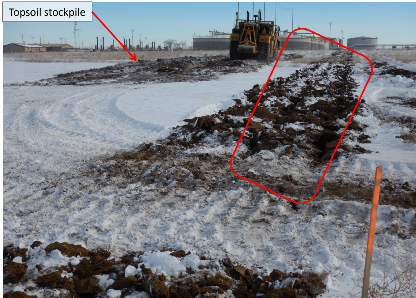
Photo 3. Photo taken from northwestern corner, facing East. Stormwater BMP installed prior to construction of well pad (highlighted in red). Surface roughening is a temporary BMP and should be used in conjunction with other BMPs.
