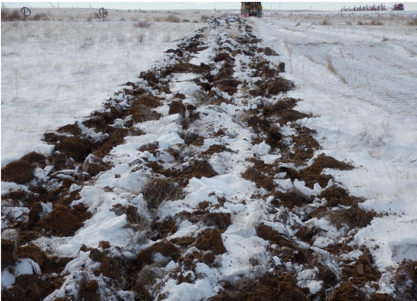
Photo 4. Photo taken from northeast corner, facing South. Stormwater BMP installed prior to construction of well pad (highlighted in red). Surface roughening is a temporary BMP and should be used in conjunction with other BMPs.
