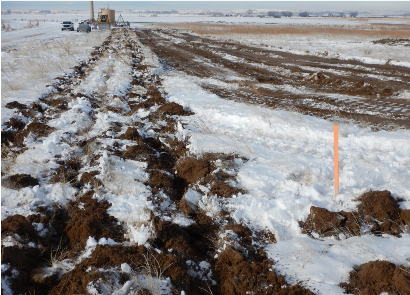
Photo 5. Photo taken from southeast corner, facing West. Stormwater BMP installed prior to construction of well pad (highlighted in red). Surface roughening is a temporary BMP and should be used in conjunction with other BMPs.
