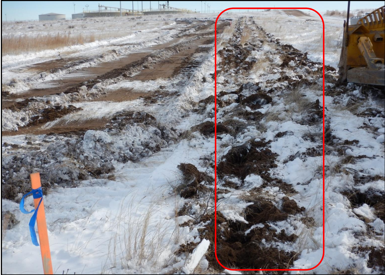
Photo 1. Photo taken from southwestern corner, facing East. Stormwater BMP installed prior to construction of well pad (highlighted in red). Surface roughening is a temporary BMP and should be used in conjunction with other BMPs.
