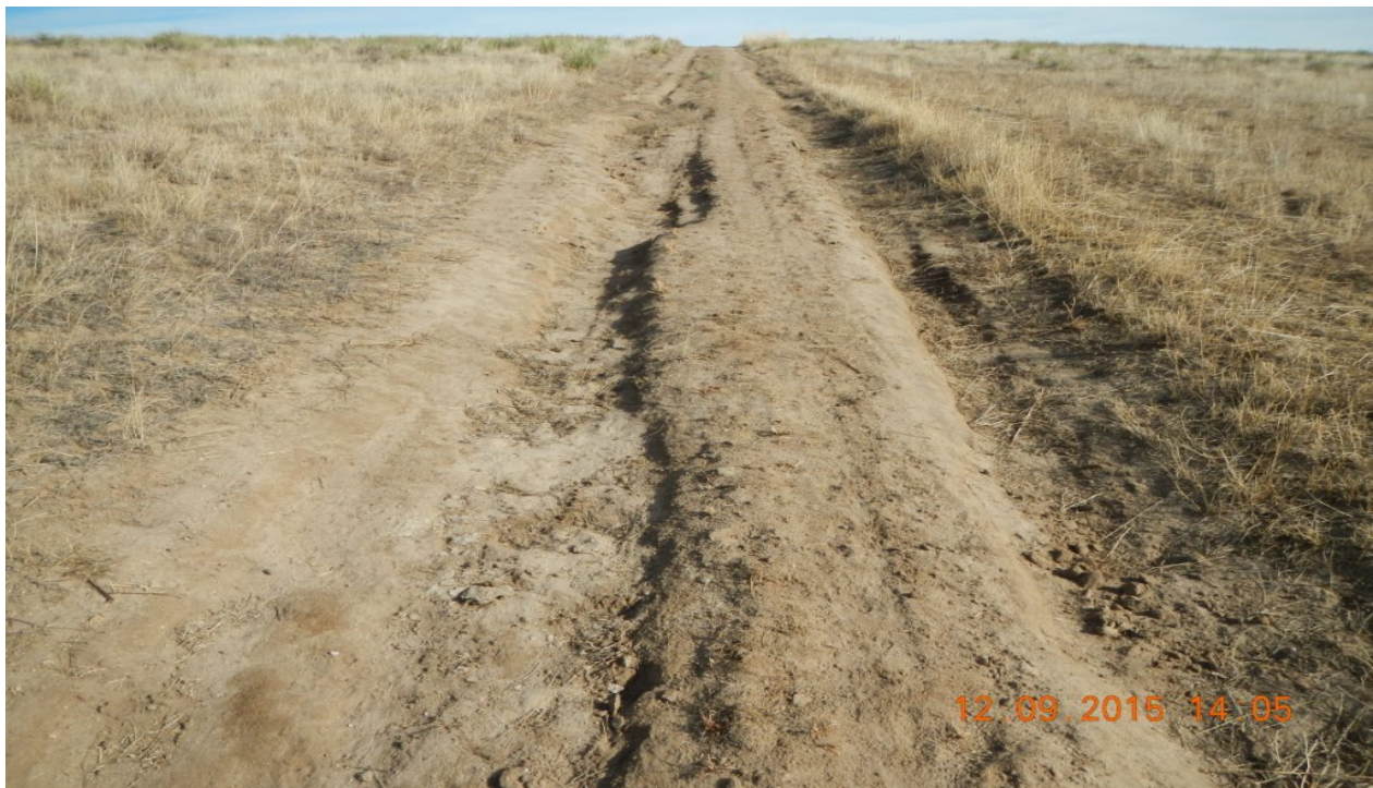
photo 2: Erosion occurring along the access road.
